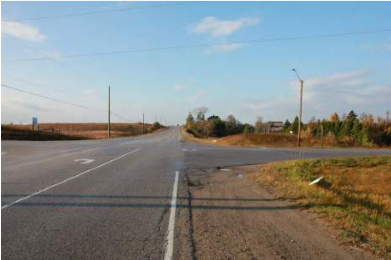
Figure 4 – Wellington Rd 52 facing West from 10 th Line Intersection
