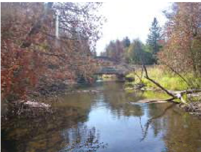
Photo 33: Upstream view of 10 th Line Bridge.
