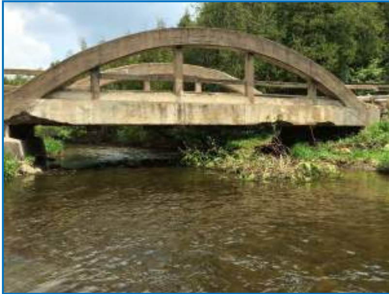
Photograph 11. Bridge located at 10 th Line, looking downstream
