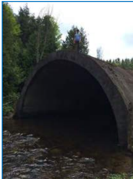
Photograph 12. East side of culvert located at Winston Churchill Blvd., looking upstream
