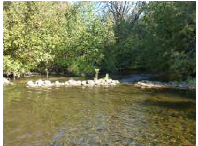
Photo 23: Downstream view at rock dam.
