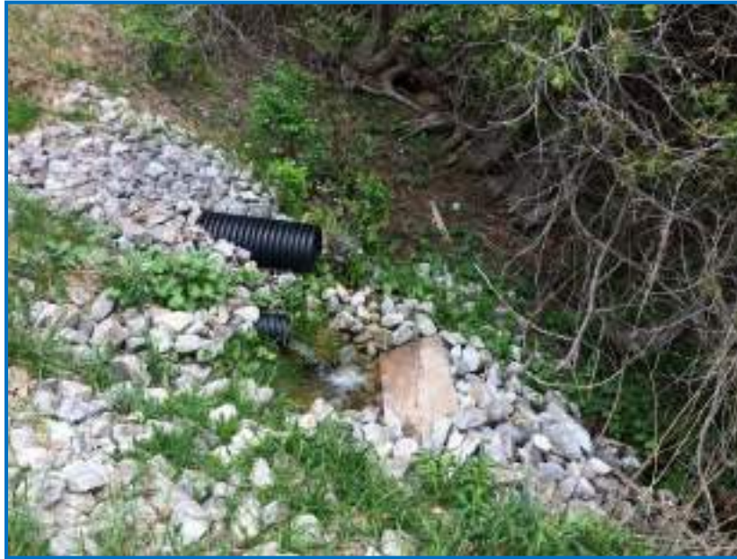
Photograph 13. Groundwater seep at Winston Churchill Blvd
