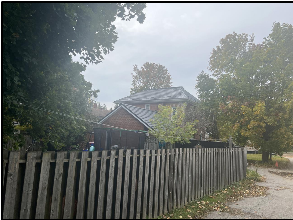
Image 10: Rear Elevation of 81 Trafalgar Road (Photo taken on October 19, 2023; Facing South)
