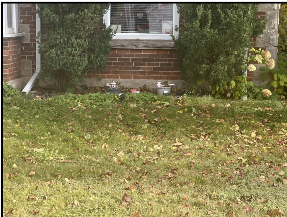
Image 4: Detail of Foundation of 81 Trafalgar Road (Photo taken October 19, 2023; Facing Northeast)
