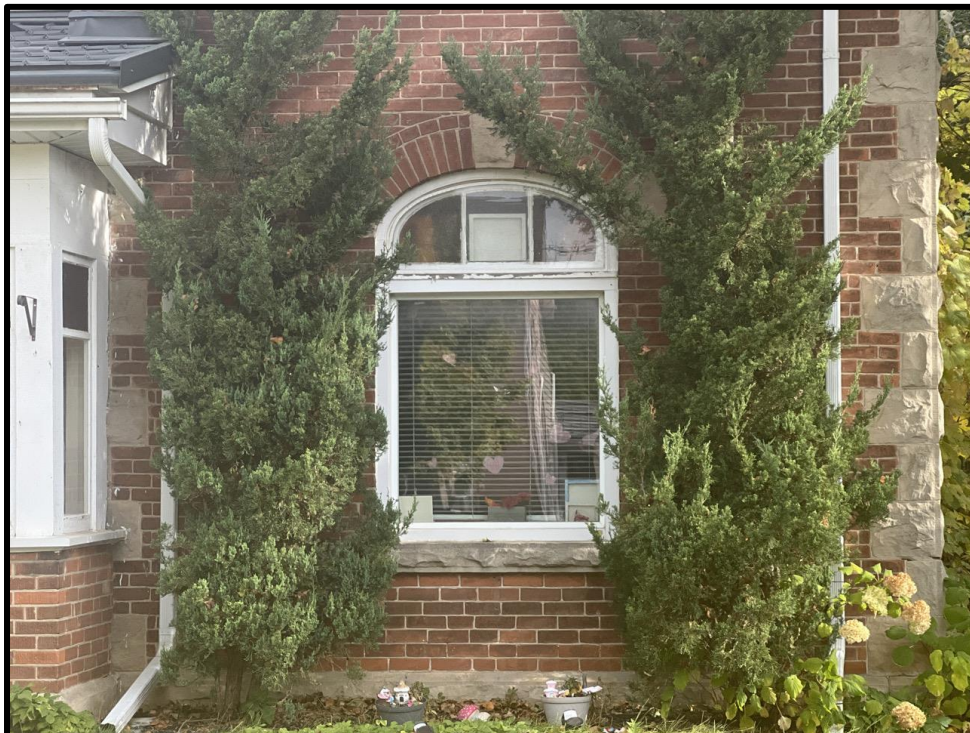
Image 2: Detail of Elliptical Arch Window Opening of 81 Trafalgar Road (Photo taken October 19, 2023; Facing Northeast)
