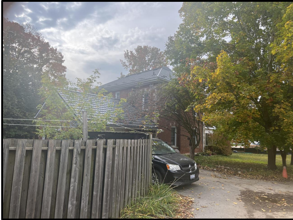
Image 9: Northeast Corner of 81 Trafalgar Road (Photo taken on October 19, 2023; Facing South)
