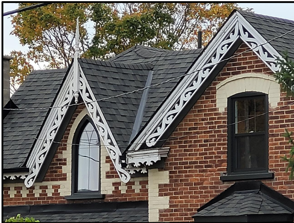
Image 2: Detail of Roofline and Second Storey Openings of 114 Trafalgar Road (Photo taken October 19, 2023; Facing West)
