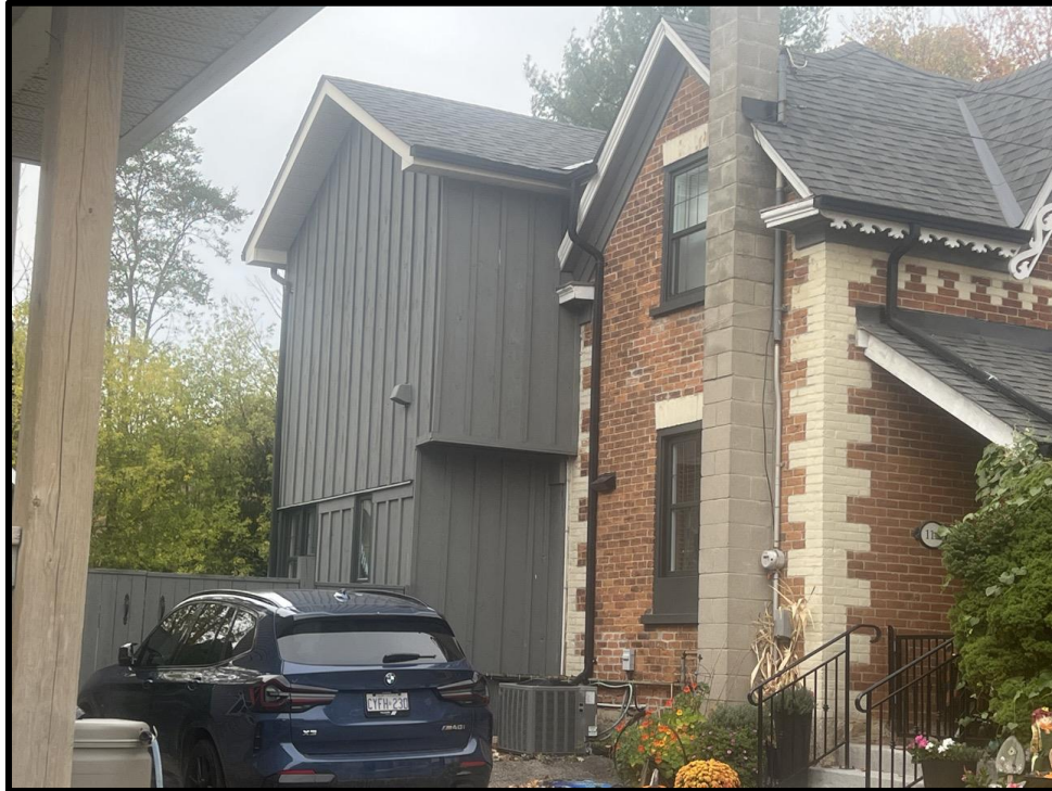
Image 8: South Elevation and Rear Addition of 114 Trafalgar Road (Photo taken October 19, 2023; Facing West)
