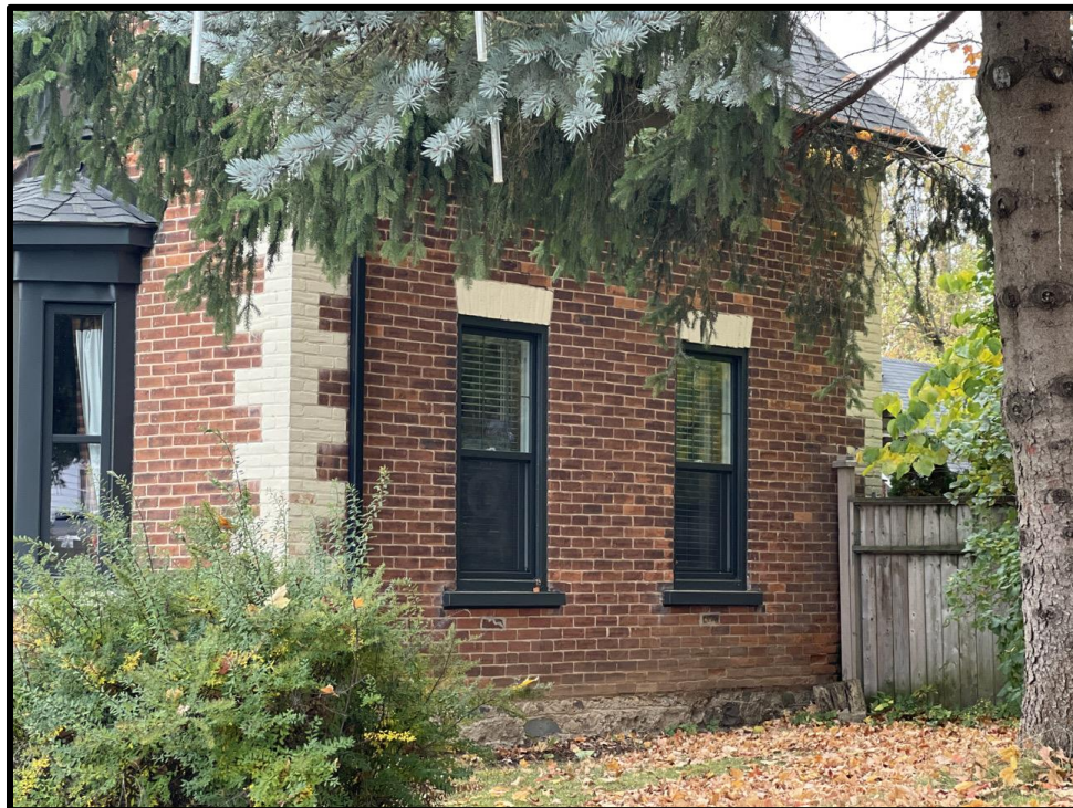
Image 4: North Elevation of 114 Trafalgar Road (Photo taken on October 19, 2023; Facing Southwest)
