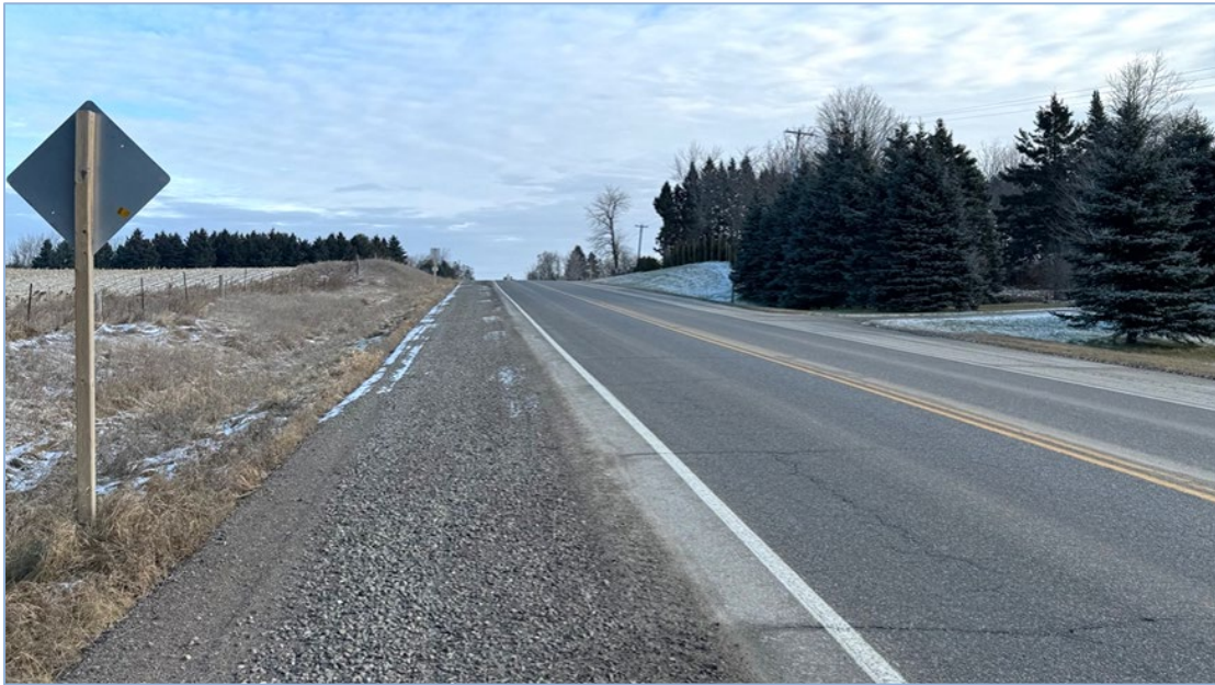
Wellington Road 22 at East Collector Rd – looking east
