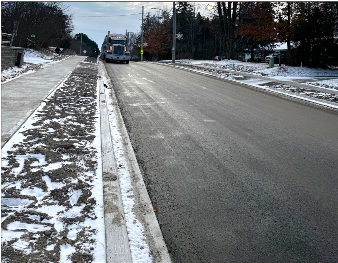
Trafalgar Road (Wellington Road 24) at Station Street – looking south
