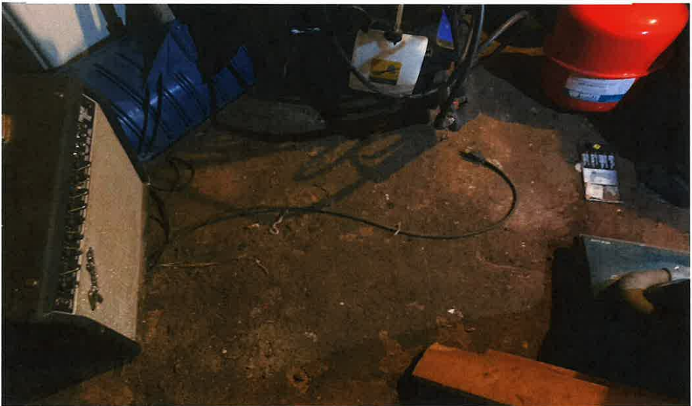
General view the basement floor at the residential building
