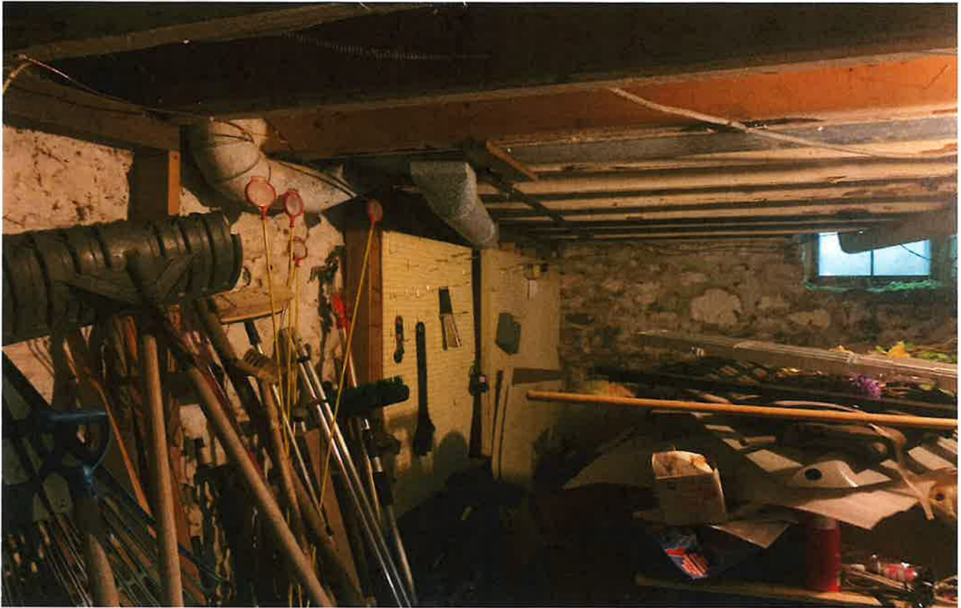
General view of basement at the residential building
