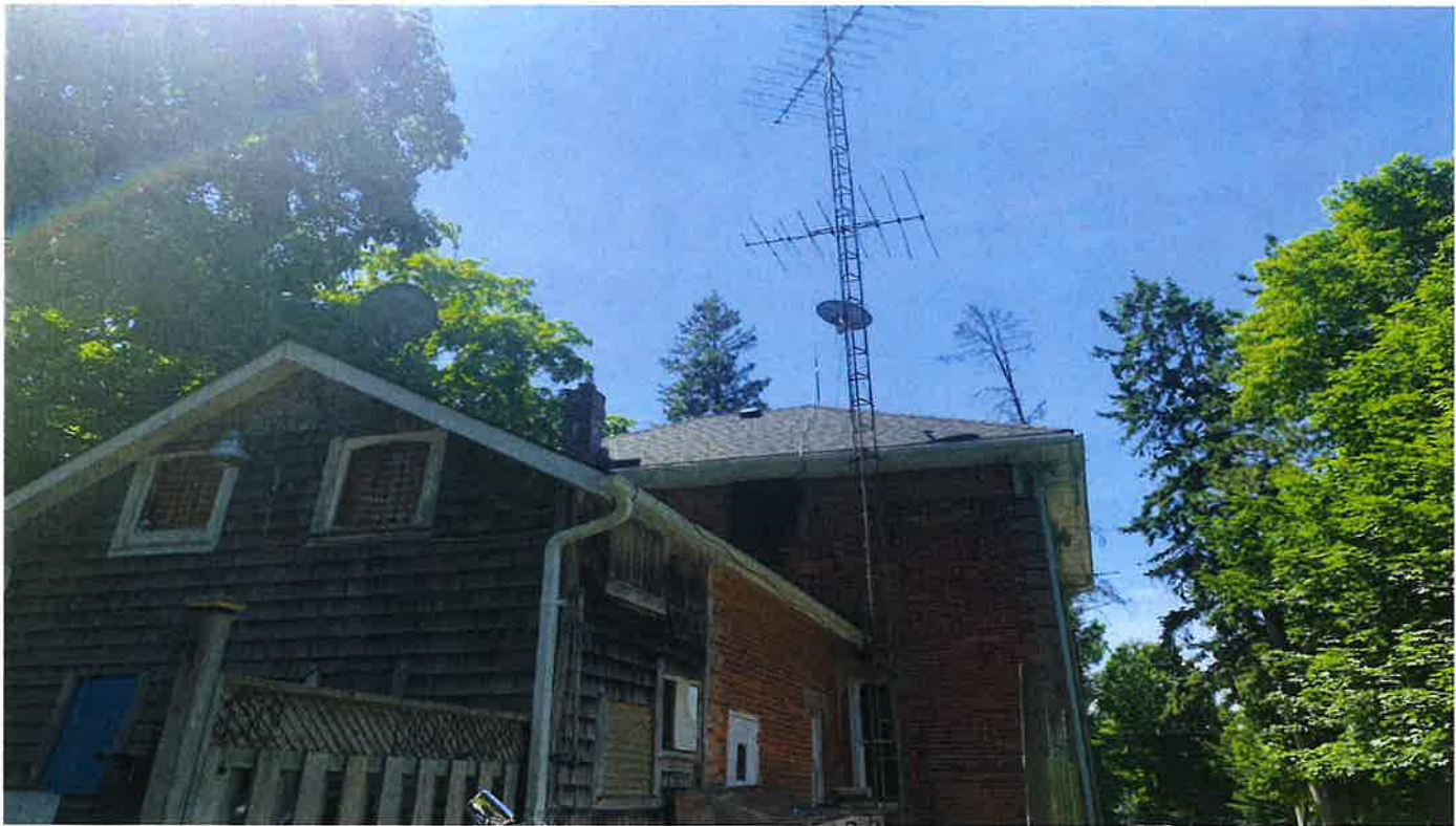
General view of residential building at 63 Trafalgar Road (looking south)
