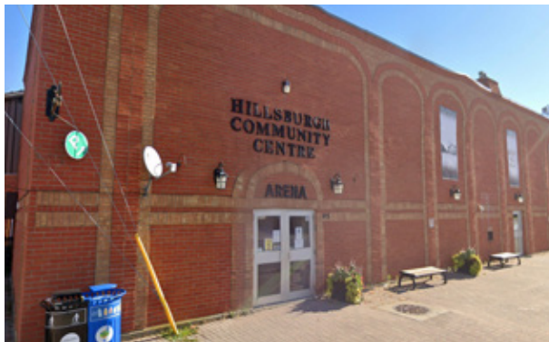
8 View of the Hillsburgh Community Centre Arena
