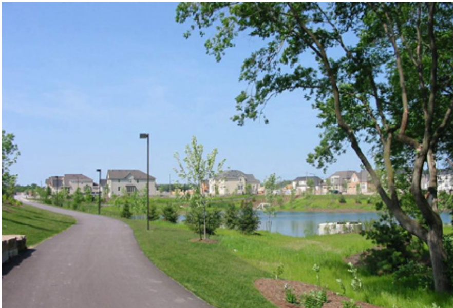
Figure 3.23: Image example of a trail integrated within the SWM pond area as a space for both ecological function and recreational activity.
