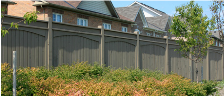
Figure 3.12: Image example of an acoustic fence between future commercial and residential developments.
