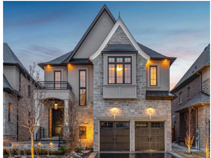
Figure 4.1: Image examples of single detached dwellings that have mix of architectural styles incorporated in the design.
