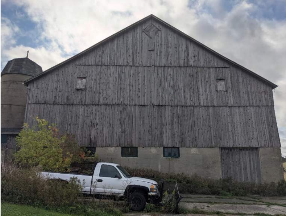
Figure 76: North elevation of large barn
