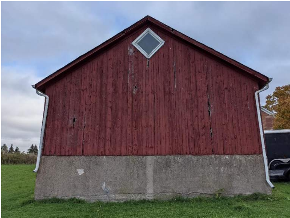
Figure 70: West elevation of the driveshed
