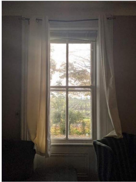
Figure 33: Wood window surround and paneling in south front room (also representative of paneling in north front room)
