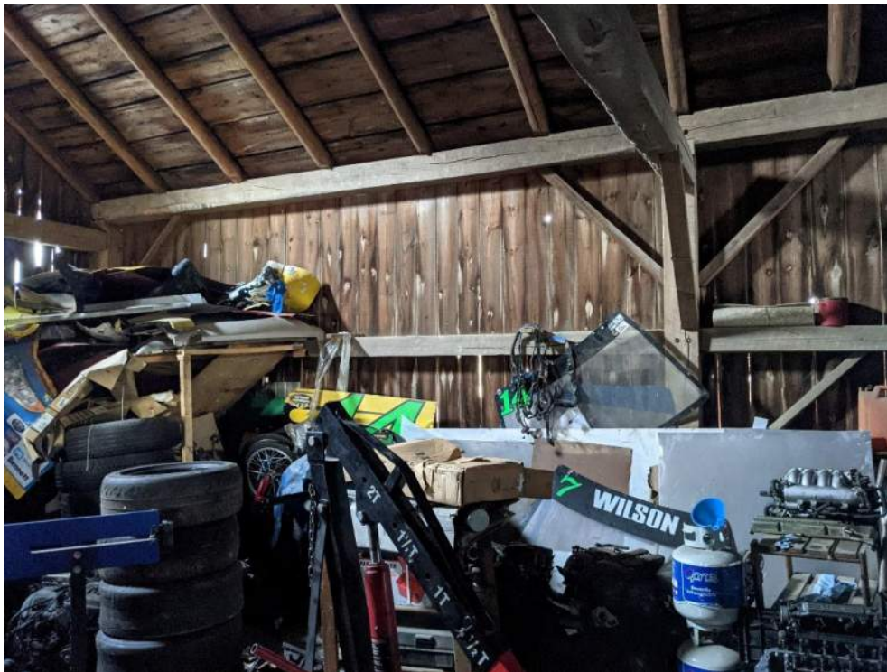
Figure 73: Interior of the driveshed with drop tie-beam, hand-hewn posts, and plates
