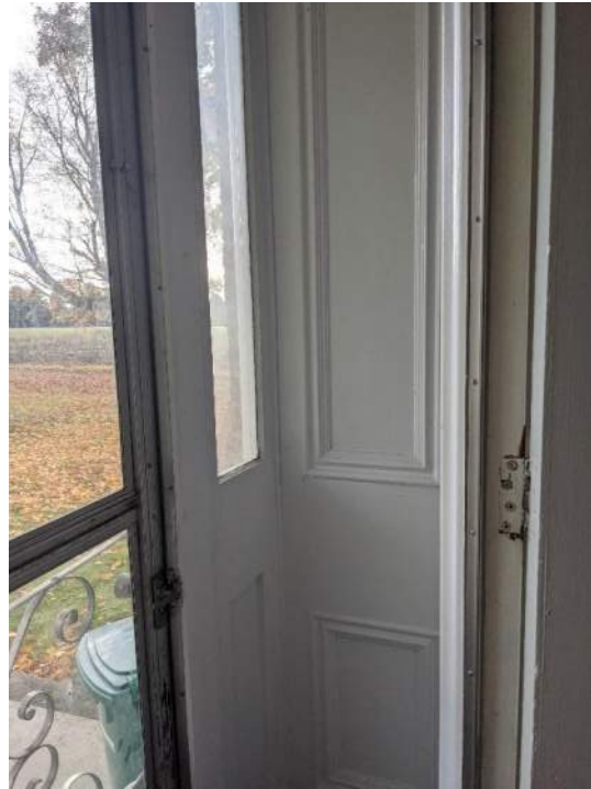
Figure 25: Wood paneling between exterior door and interior door.
