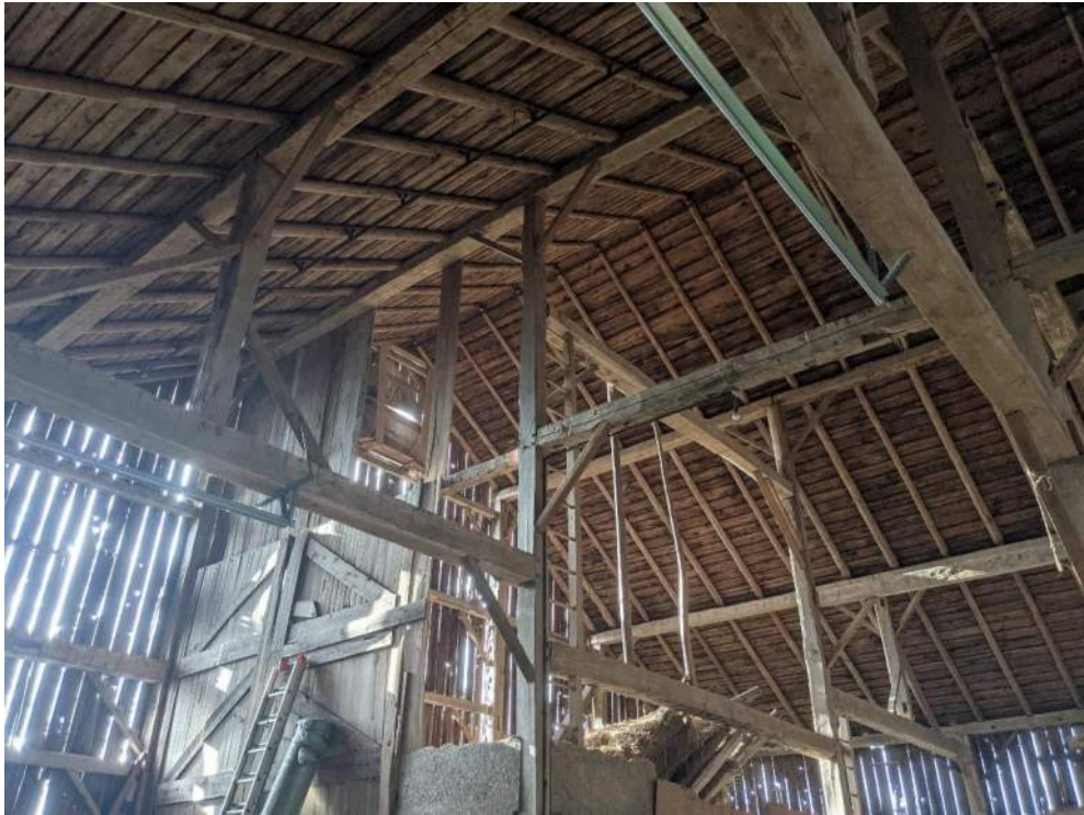
Figure 84: View of the roof rafters inside the large barn
