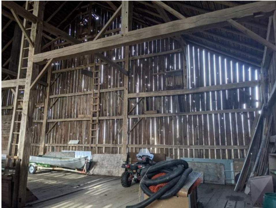
Figure 82: View of the timber frame construction
