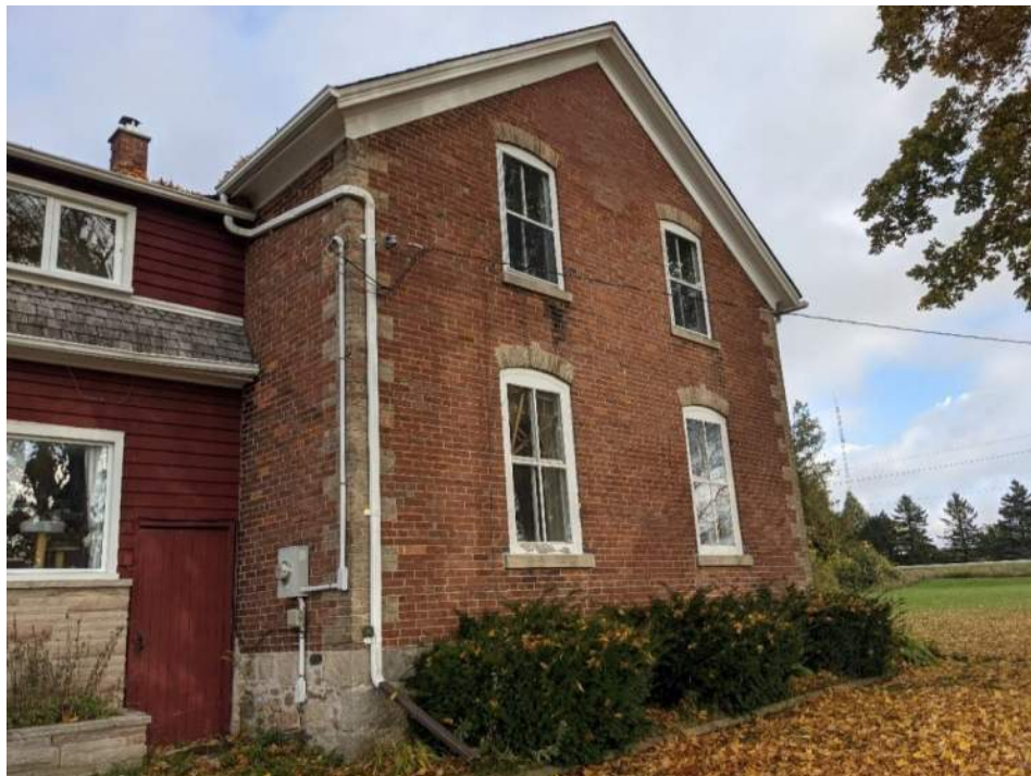
Figure 15: The south façade of the farmhouse main block
