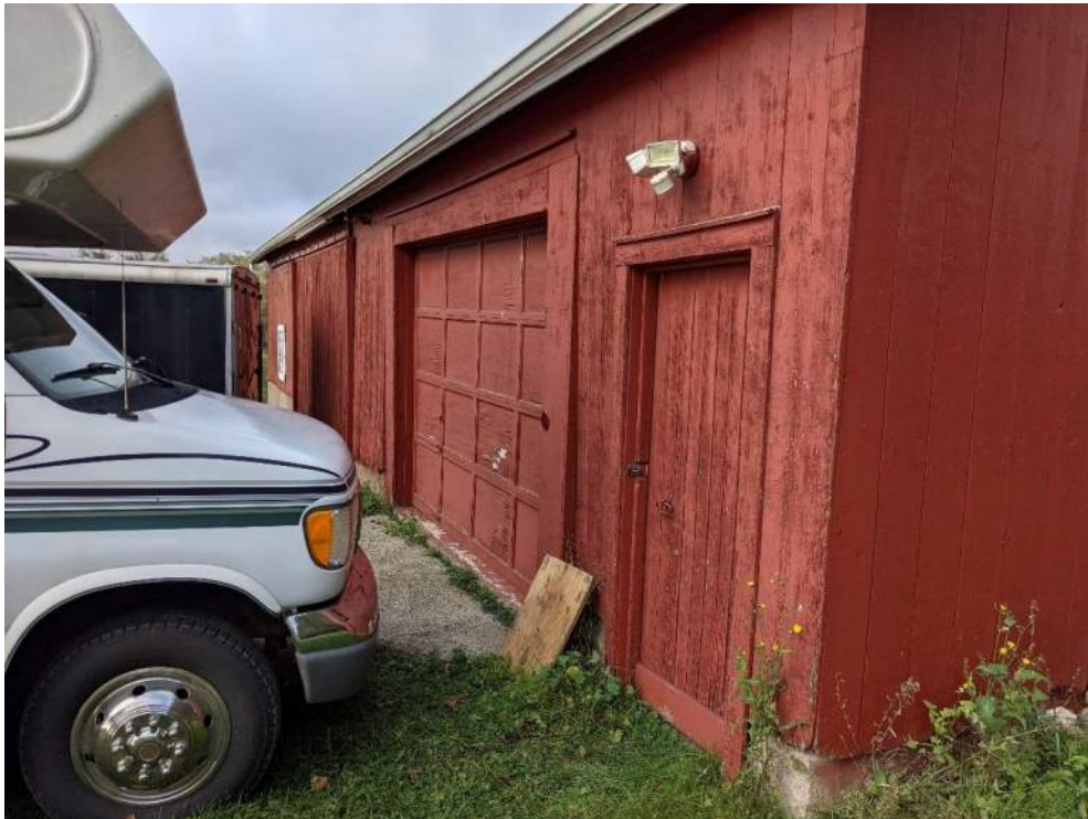
Figure 66: South façade of the driveshed
