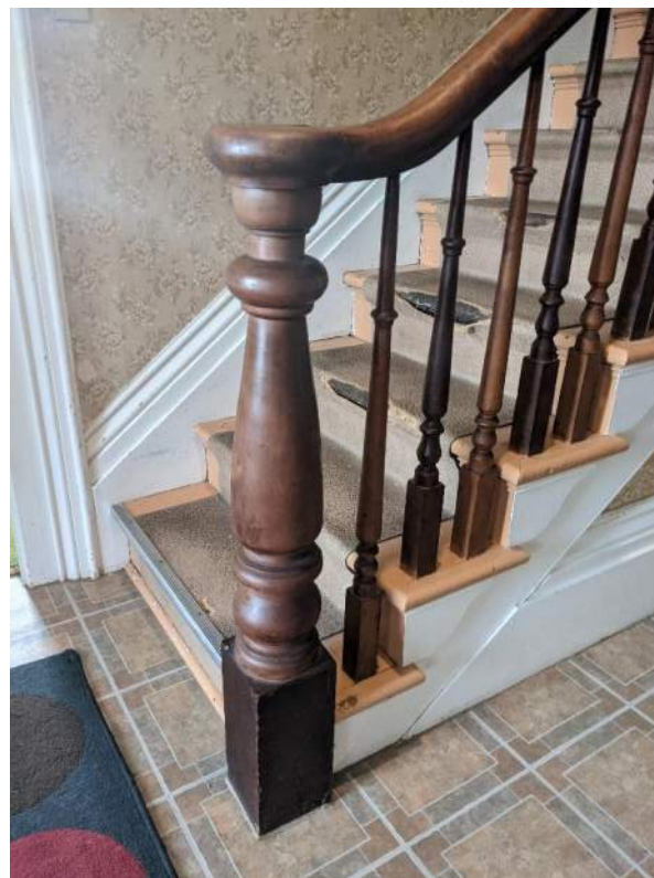
Figure 28: Staircase newel post and spindles
