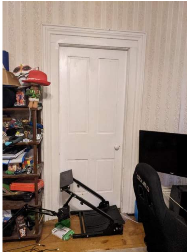
Figure 31: Four paneled door in north front room
