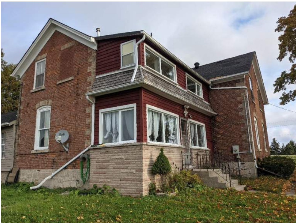
Figure 17: West façade of the rear wing and two-storey addition.
