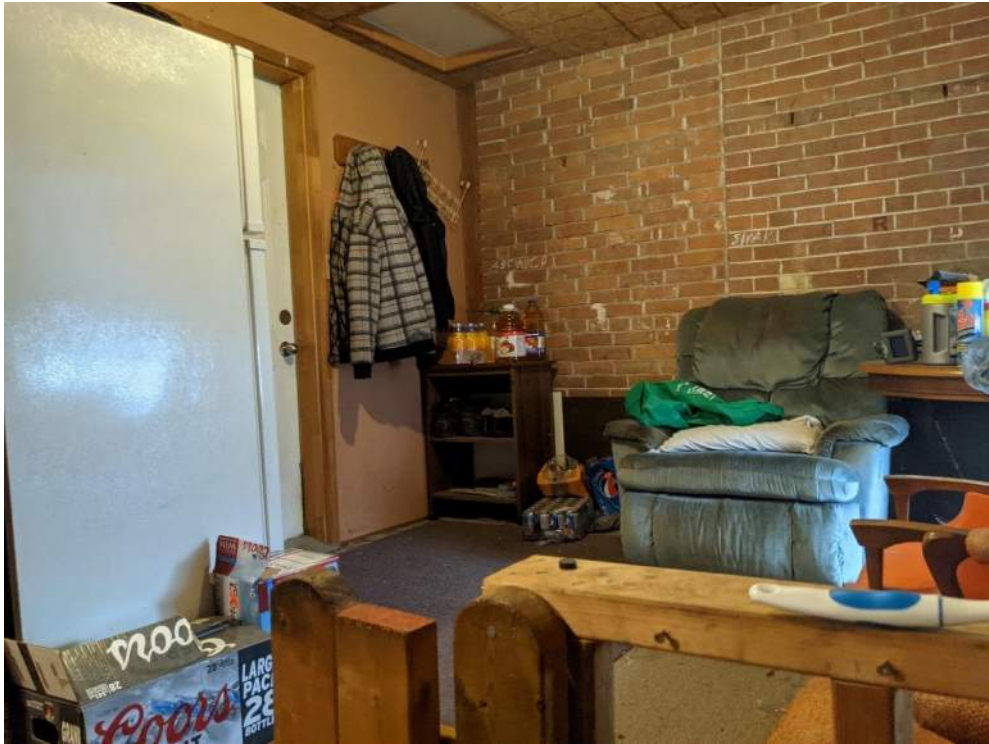
Figure 59: Interior of north addition, entrance to interior of farmhouse (left behind fridge)
