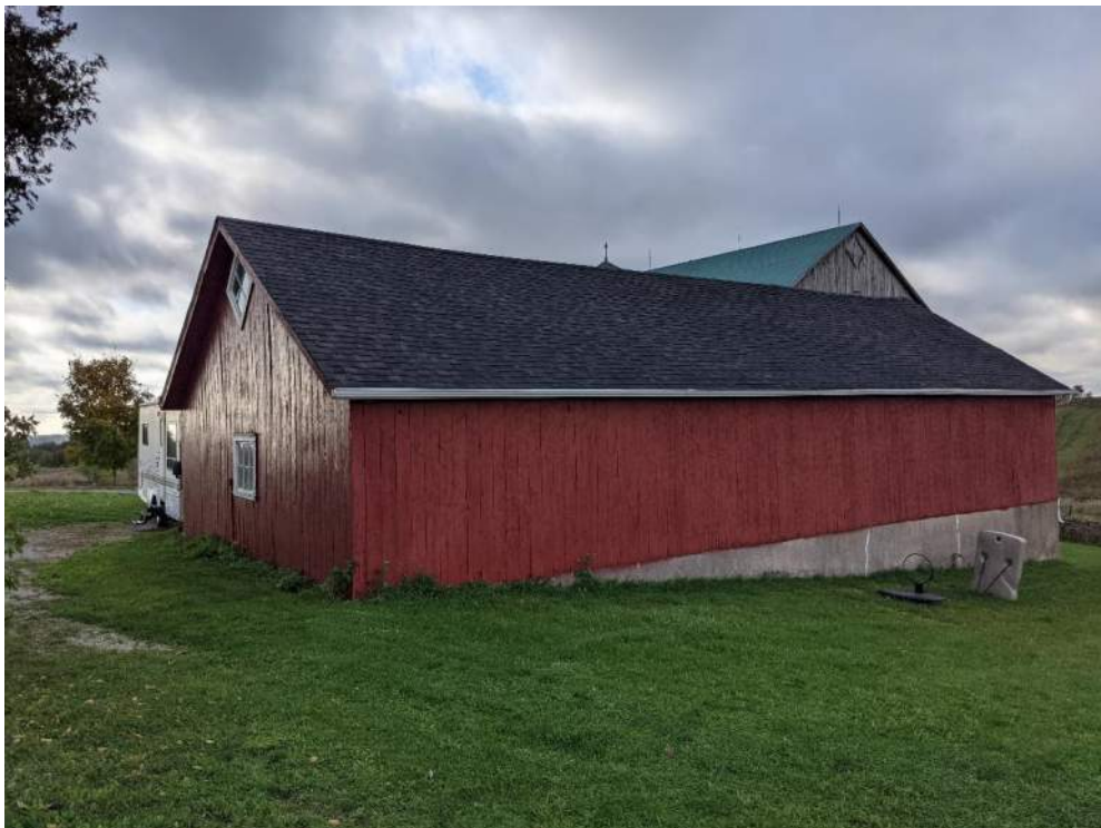
Figure 68: North façade of the driveshed
