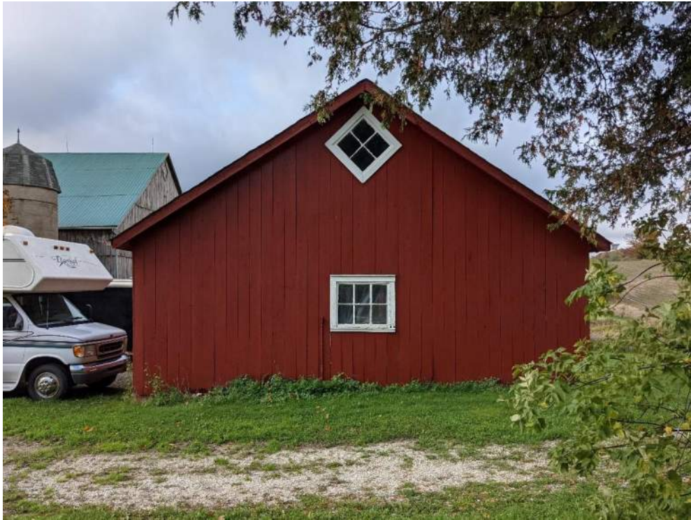
Figure 69: East elevation of the driveshed
