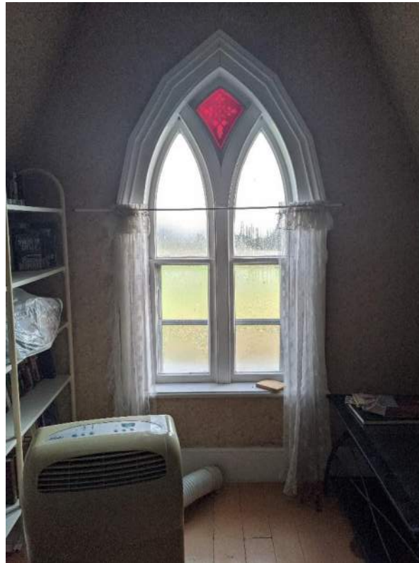
Figure 41: Interior of lancet window on east façade, not coloured and patterned glass in lancet peak
