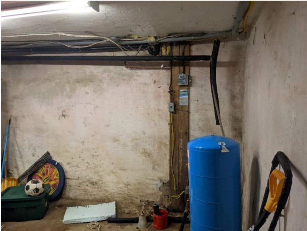
Figure 54: Wood support column
