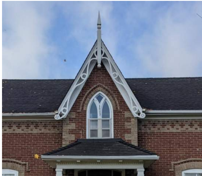
Figure 21: Gable peak on east façade
