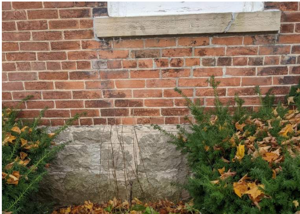
Figure 19: Stone foundation and common bond brick on south elevation.
