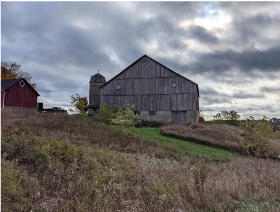
Figure 79: South façade of the large barn
