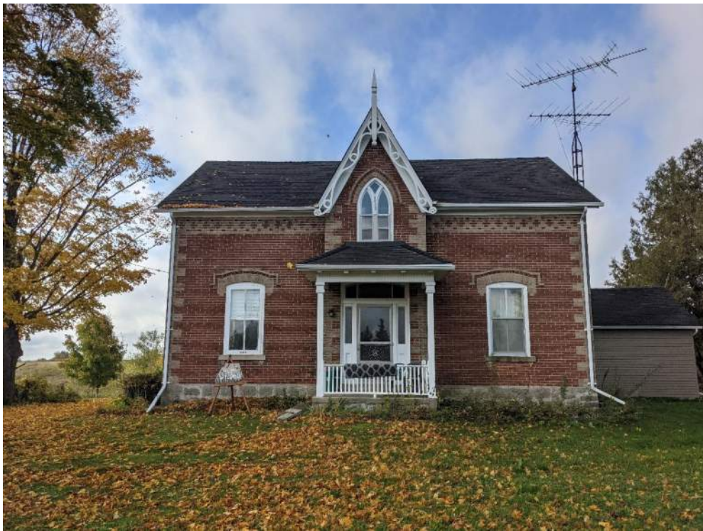
Figure 13: Front or east façade of the Farmhouse
