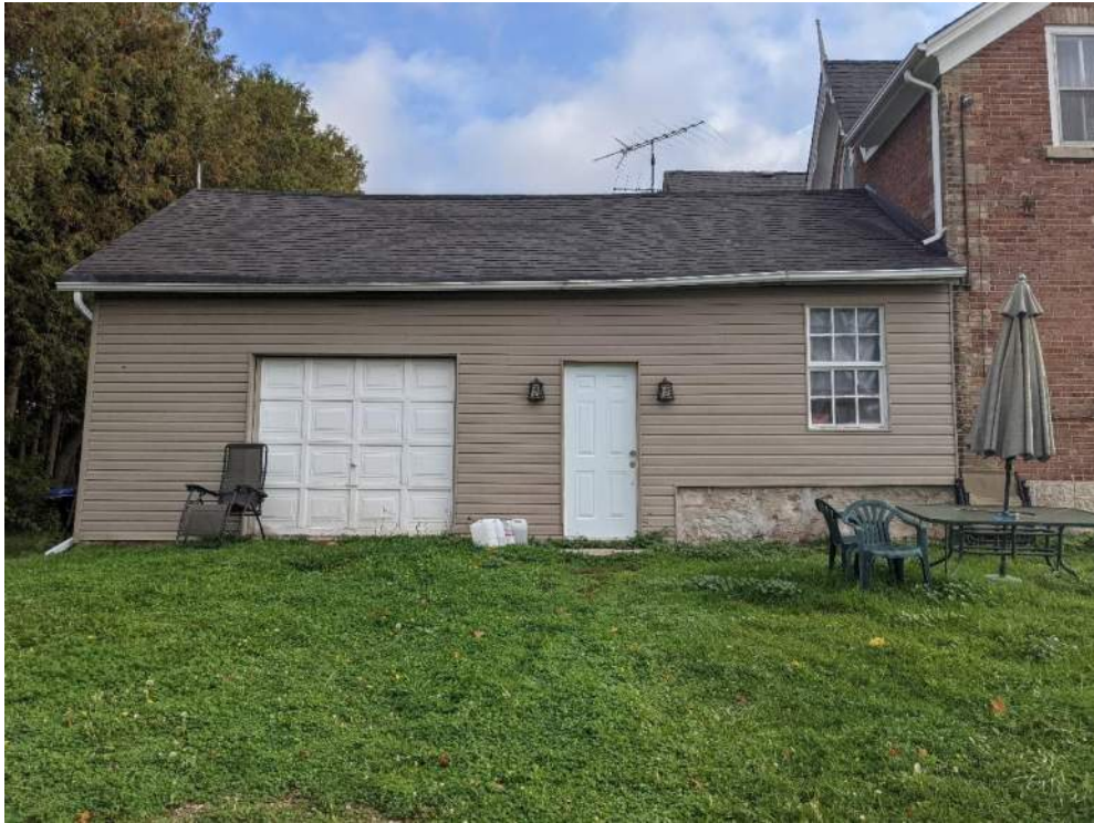
Figure 55: West elevation of the north addition
