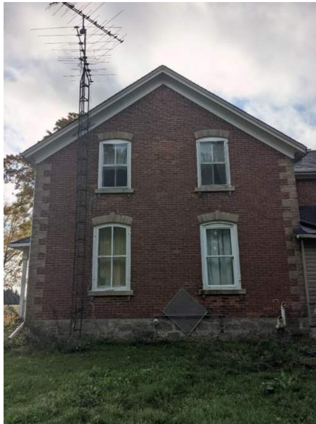
Figure 14: North façade of the Farmhouse's main block
