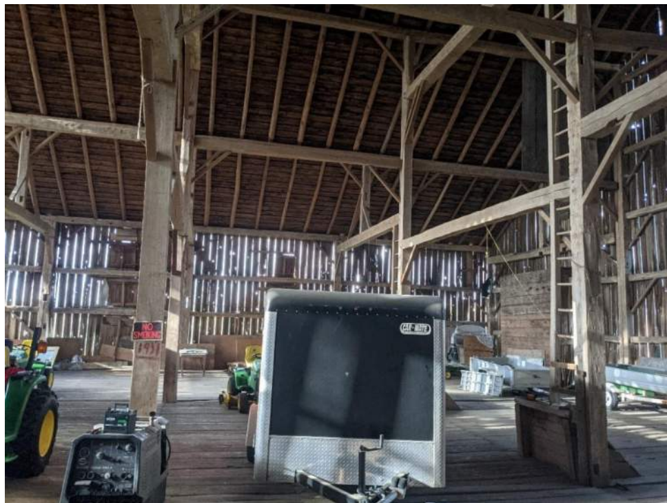
Figure 83: View of threshing floor inside the large barn
