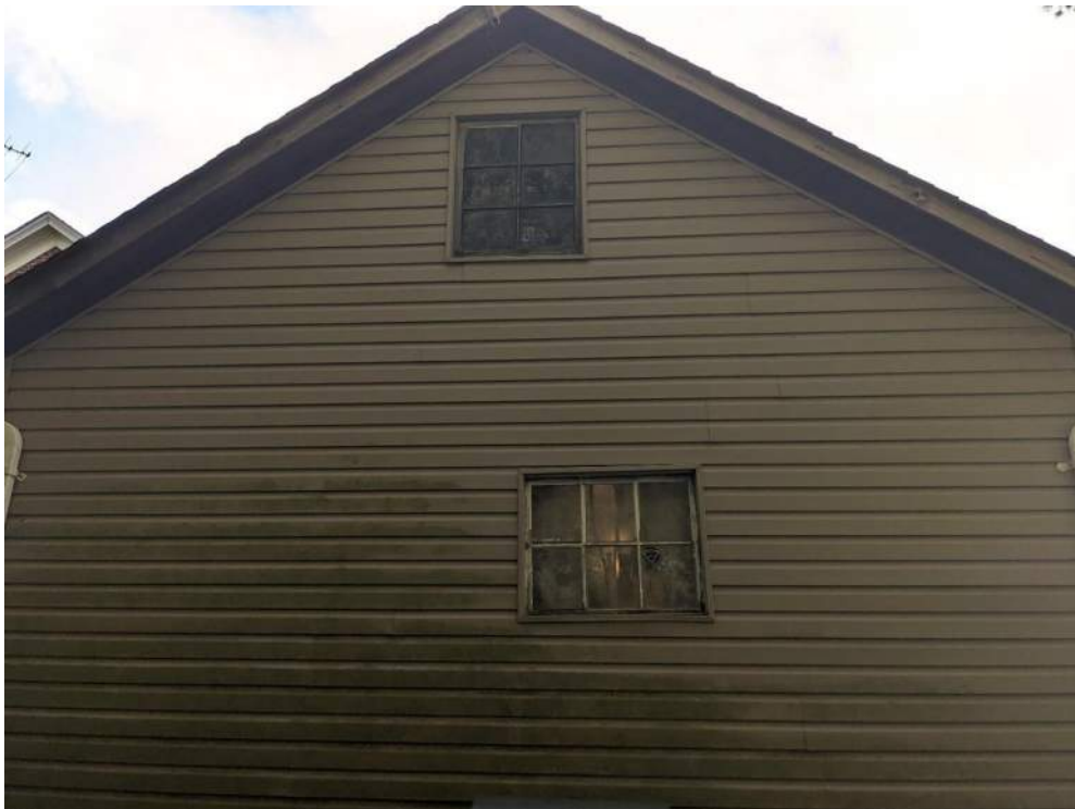
Figure 58: North elevation of the north addition
