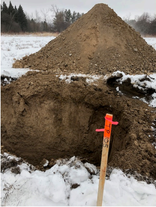
Photograph 5- Excavated soils from TP 105. After 4.0 hours, cave-in of sides and water level were observed at 3.0 m below existing grade.
