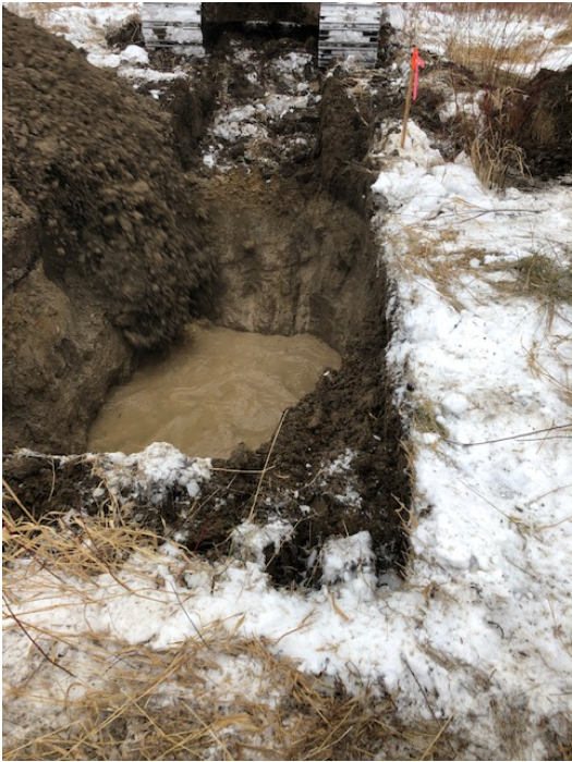
Photograph 12- View of TP 109 approximately 5 hours after completion.
