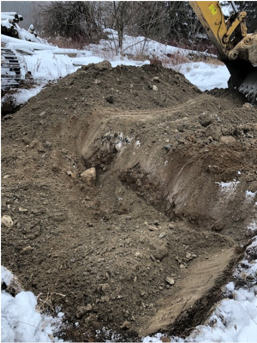
Photograph 14- View of excavated soil being used to backfill TP 110.
