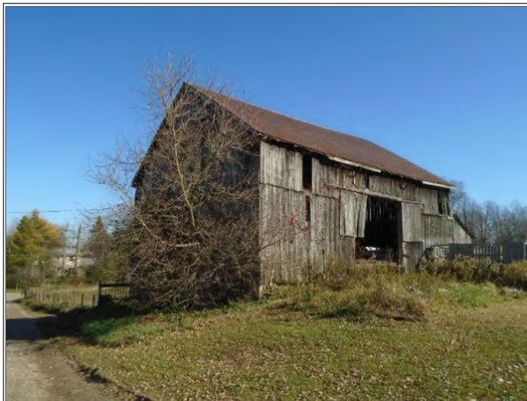
Photo 4 –Southwest elevation of Site Building B, looking northeast.
