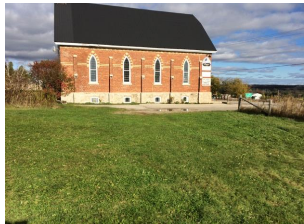
Plate 12. Grass Covered Church Parking Area (view northeast)
