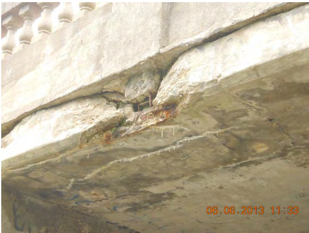
Spalls, exposed corroded rebar on fascia.
