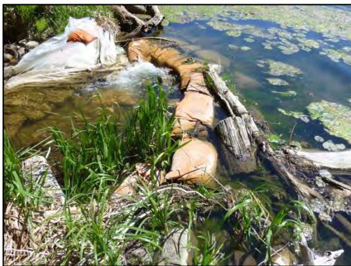
Image 5. Partial Fish Barrier, north upstream reach of segment 7.
