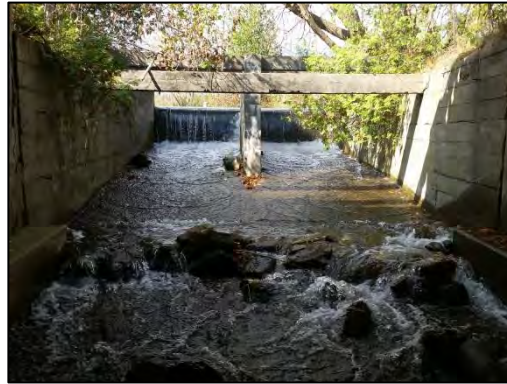
Image 4. Full Fish Barrier, upstream reach of segment 5.
