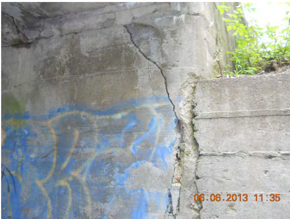
Wide crack on abutment.
