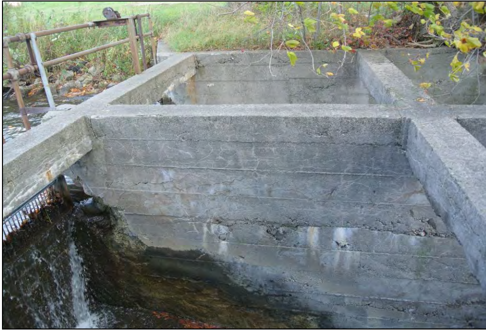
Plate 19: Detail of stop log control structure.
