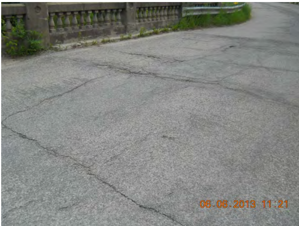
Narrow to wide cracks on wearing surface.
