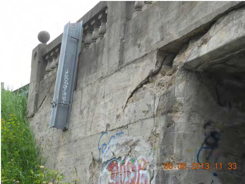
Spalls, delamination on wingwall and fascia.
