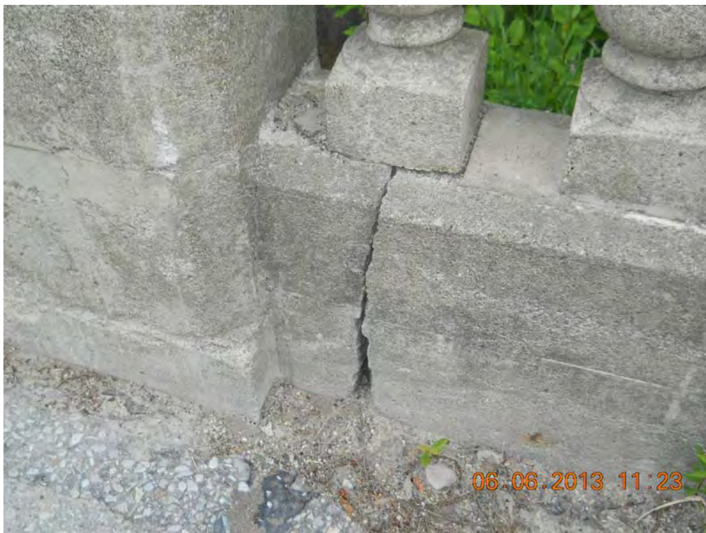
Wide crack on barrier.
