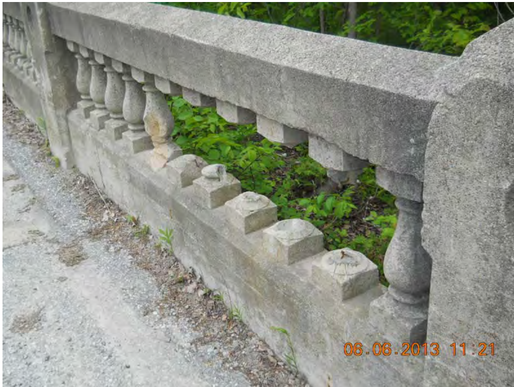
Missing spindles on barrier.
