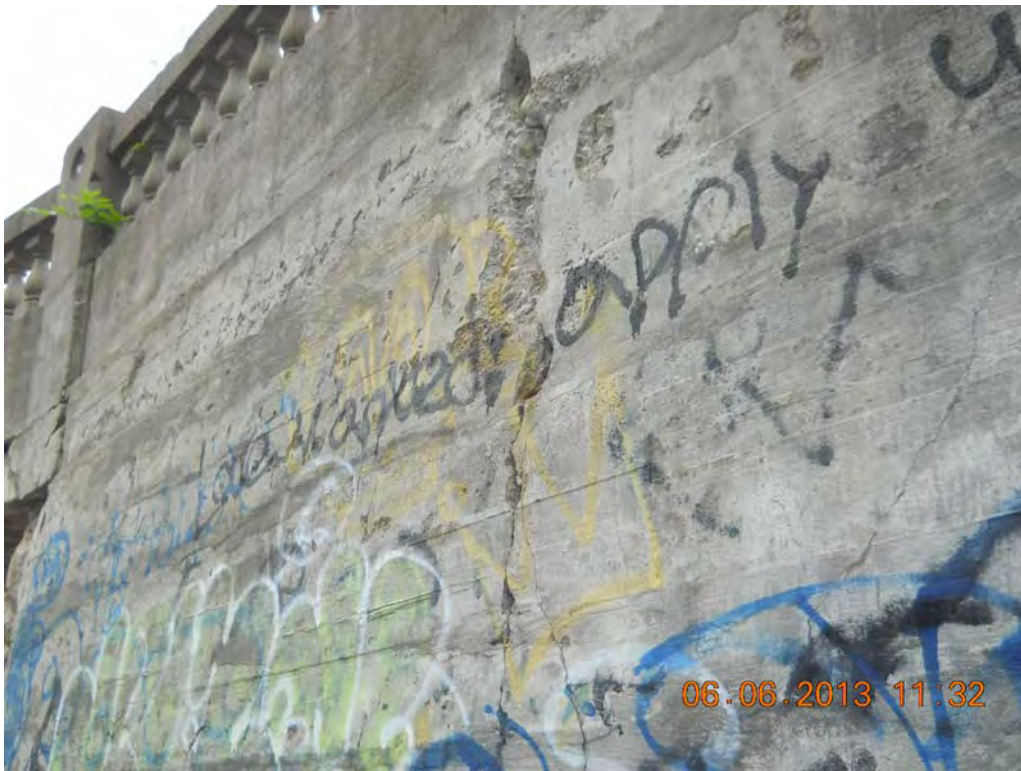
Spalls, wide crack on wingwall.
