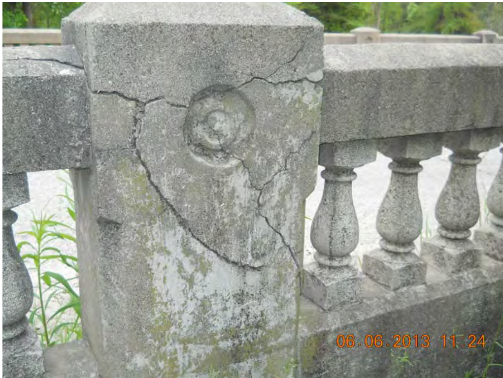
Delaminations, wide cracks on barrier post.
