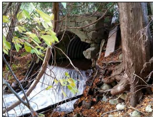
Image 6. Full Fish Barrier, south upstream reach of segment 7.
