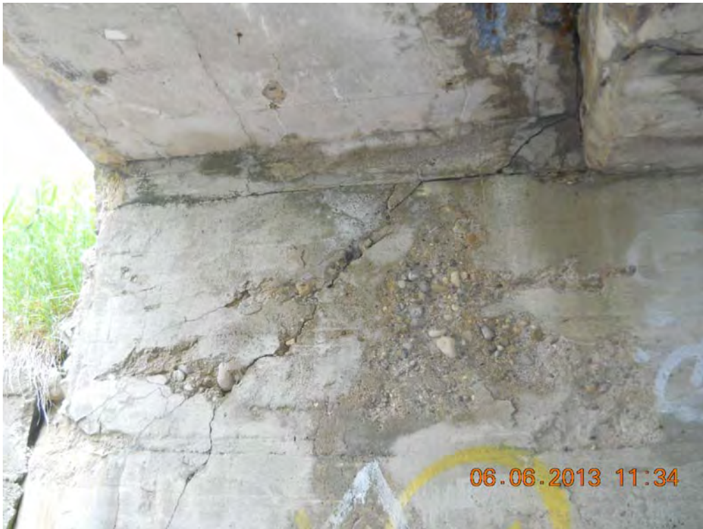
Delamination, spalling and scaling on abutment.
