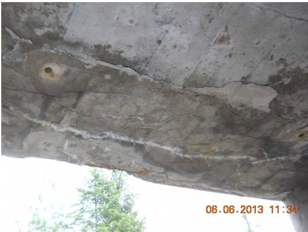
Delamination and efflorescence on soffit.
