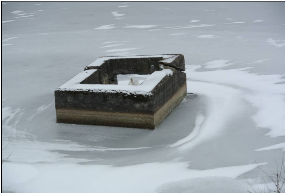
Plate 5: Detail of “Monk” culvert west of the Hillsburgh Dam, looking west.
