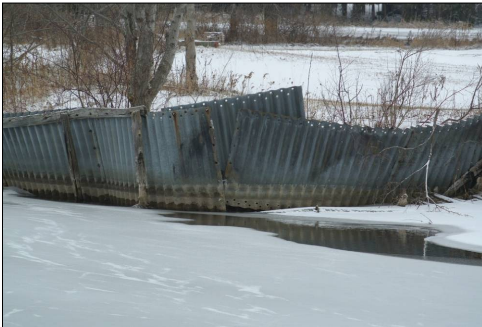
Plate 26: Detail of corrugated metal used in the bank protection on the northeast shore of the pond.
