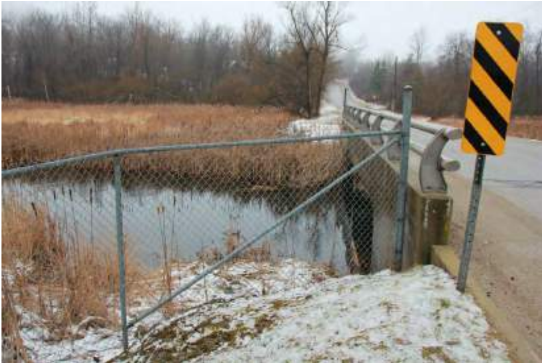
Figure 11 – West Credit River crossing with Dundas Street
