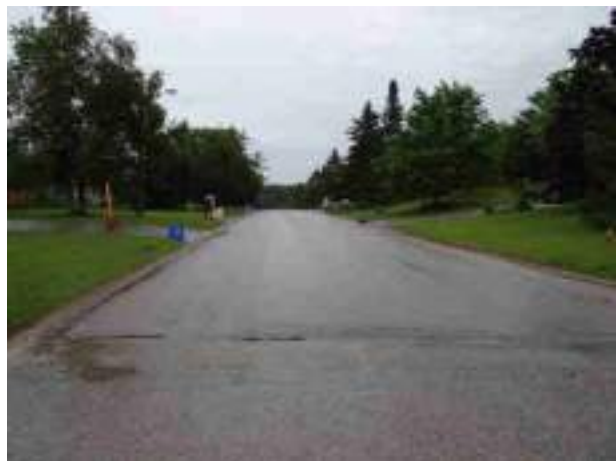
Plate 32: Northeast view of Erin Height Blvd, Erin; Proposed sewer route is within the disturbed road, no Stage 2 required.
