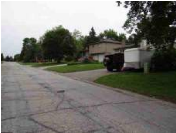
Plate 23: North view of SPS site #7, Erin; sewer route, and forcemain are within the disturbed road, if proposed SPS site #7 will impact the lawn, Stage 2 test pit survey is required
