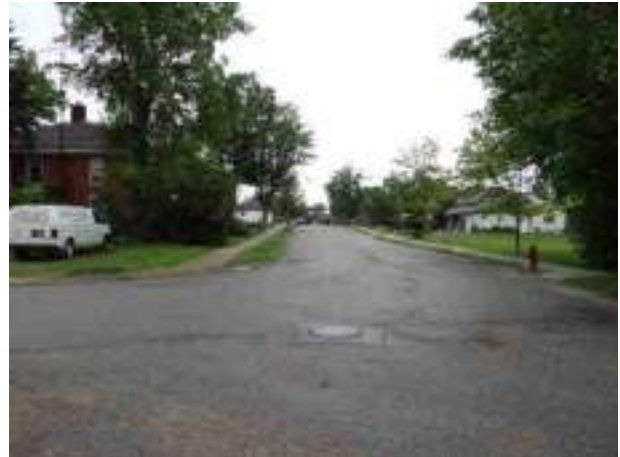
Plate 26: Northeast view of Church St and Church Blvd, Erin; Proposed sewer route is within the disturbed road, no Stage 2 required
