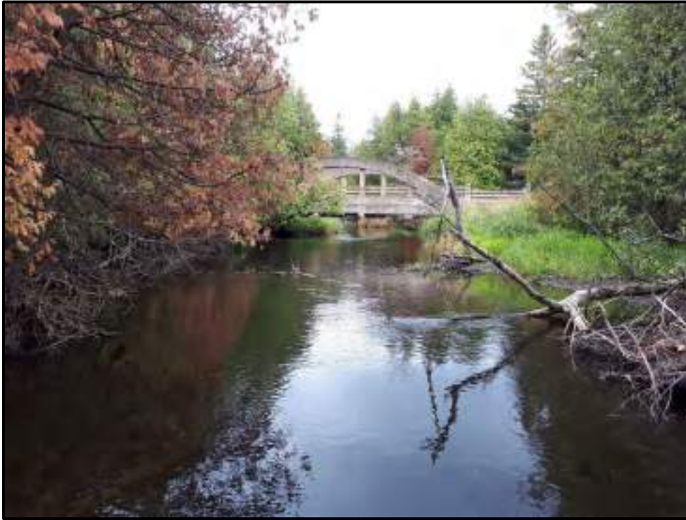
Photograph 5. A view of the West Credit River facing the 10 th Line from approximately 20 m downstream.
