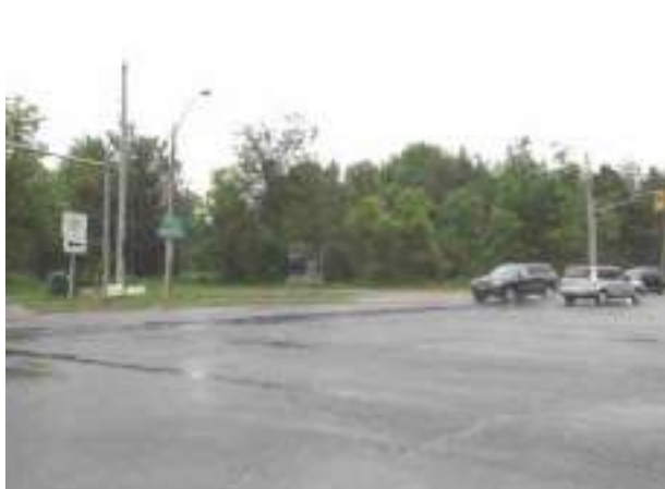
Plate 37: East view of SPS site #1A; Area surrounding the disturbed parking lot retains potential, requires Stage 2 test pit survey
