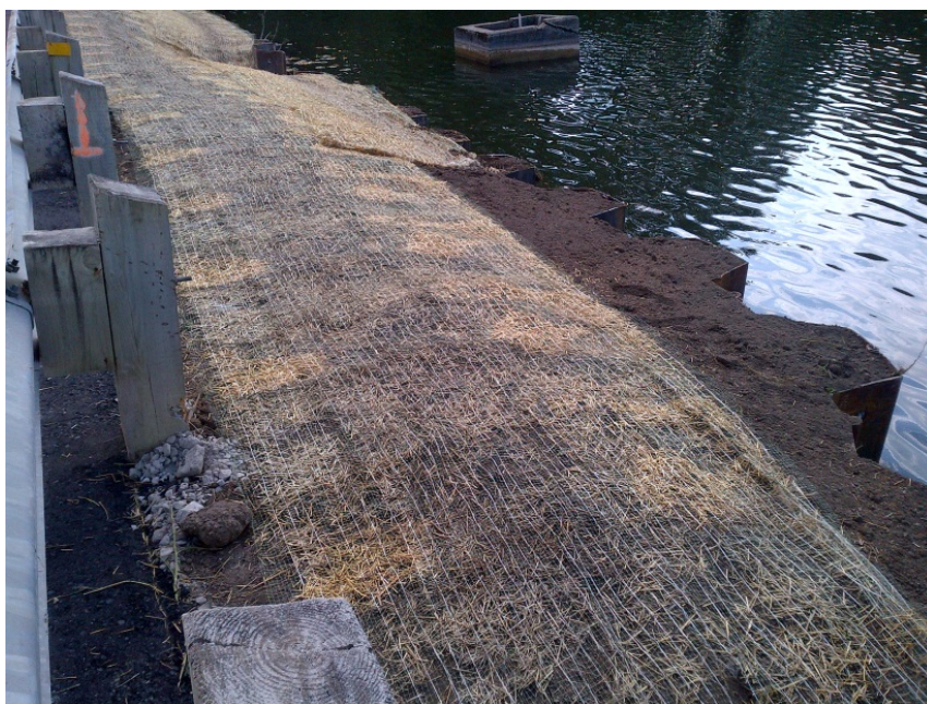
Photo 7 – Corrugated Metal Sheet Piles – Installed along the upstream side of the Hillsburgh Dam within repaired area as part of the Non-Application Emergency Repairs.
