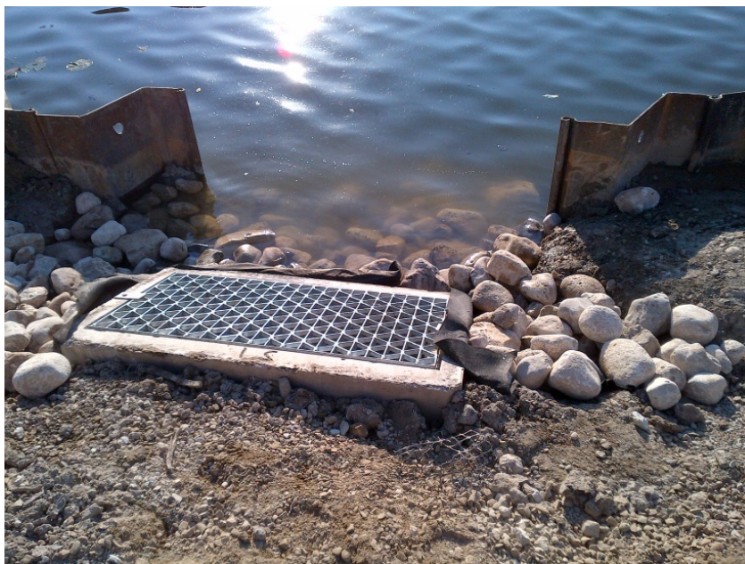
Photo 6 – New Ditch Inlet – Within Town road right-of-way installed as part of the Non-Application Emergency Repairs
