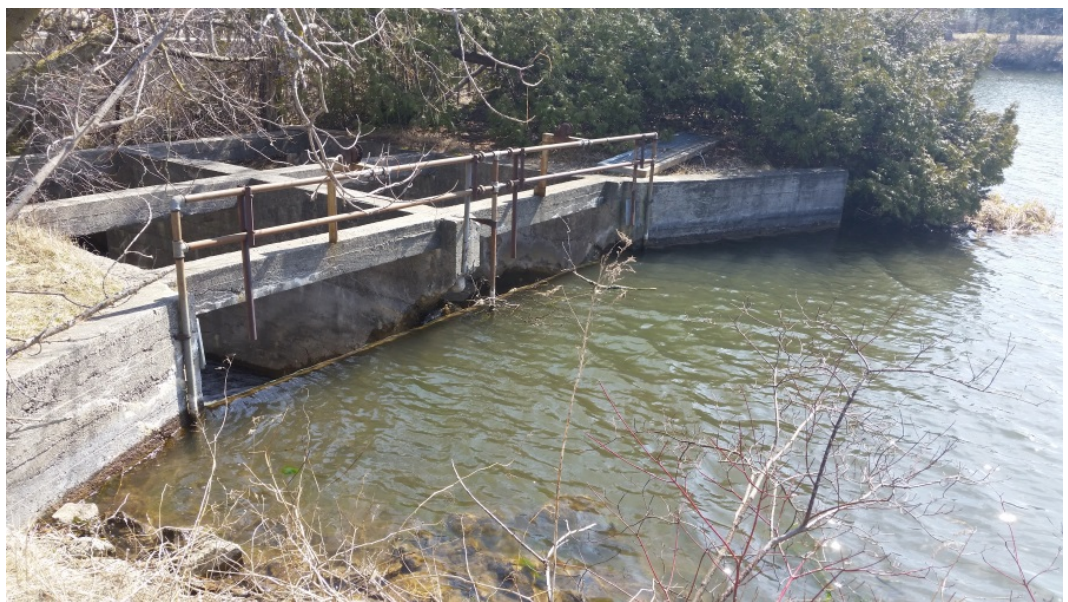
Photo 4 – Stop Log Control Structure – Looking downstream from east shoreline
