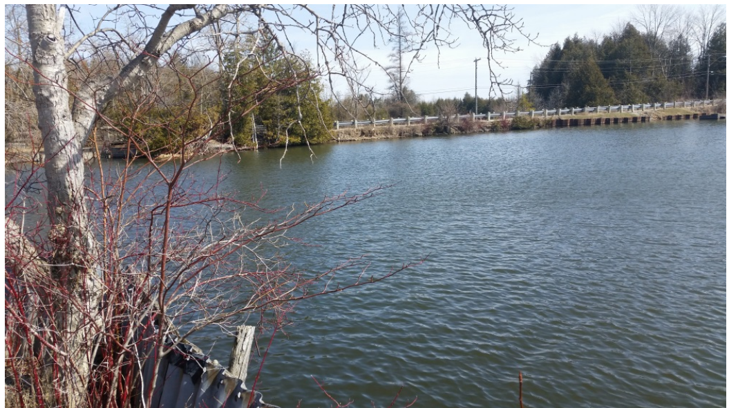
Photo 2 - Hillsburgh Dam – Looking south from east shoreline
