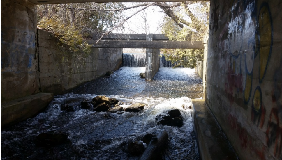
Photo 3 – Stop Log Control Structure and Spillway– Looking upstream under Bridge
