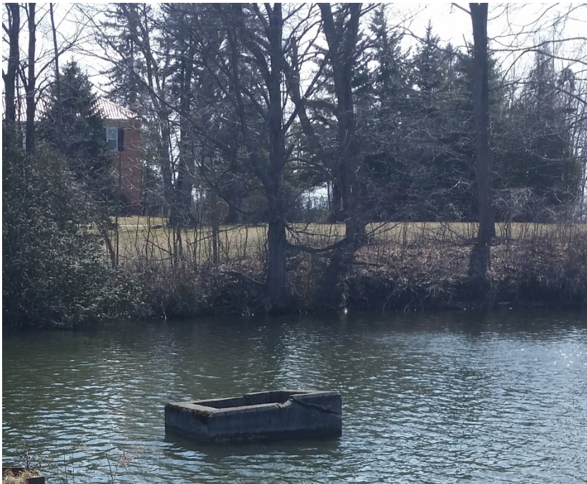
Photo 5 – Monk Riser Structure – Looking upstream from Station Street
