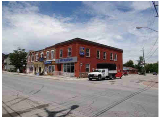
Plate 6: North view of Main St and Mill St, Hillsburgh; Proposed sewer route and forcemain are within the disturbed ROW, no Stage 2 required
