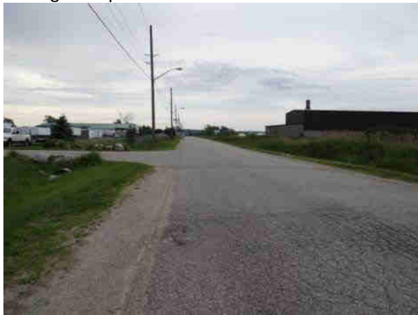
Plate 13: Southeast view of Erin Park Dr, Erin; Proposed sewer route is within the disturbed ROW, no Stage 2 required
