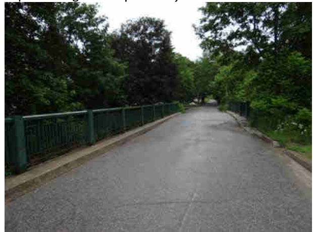
Plate 36: South view of Charles St and bridge, Erin; Proposed sewer route is within the disturbed road, no Stage 2 required.
