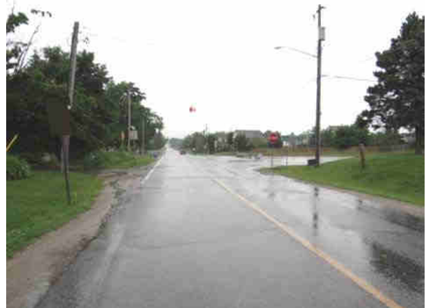
Plate 38: Northwest view of 9 th Line and Wellington Rd 52, Erin; Proposed sewer route and forcemain are within the disturbed road, no Stage 2 required.
