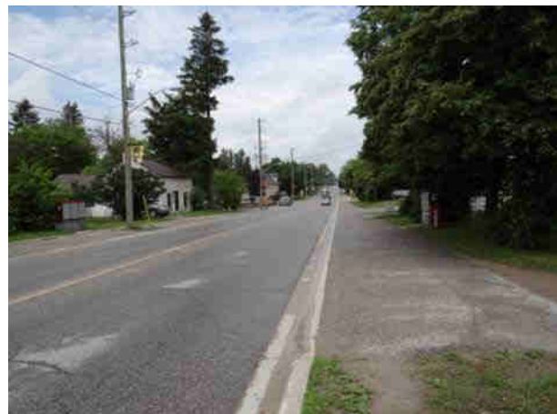
Plate 4: Northwest view of Main St, Hillsburgh; Proposed sewer route is within the disturbed ROW, no Stage 2 required
