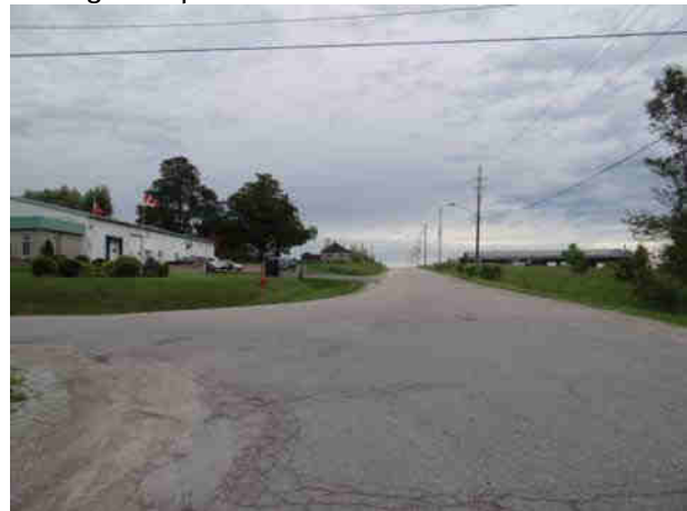
Plate 14: Northeast view of Erinville Dr, Erin; Proposed sewer route is within the disturbed ROW, no Stage 2 required
