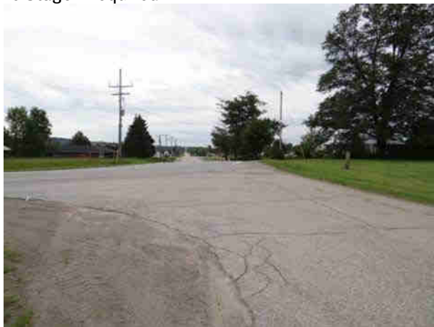
Plate 15: South view of Wellington 23 Rd, Erin; Proposed sewer route is within the disturbed ROW, no Stage 2 required
