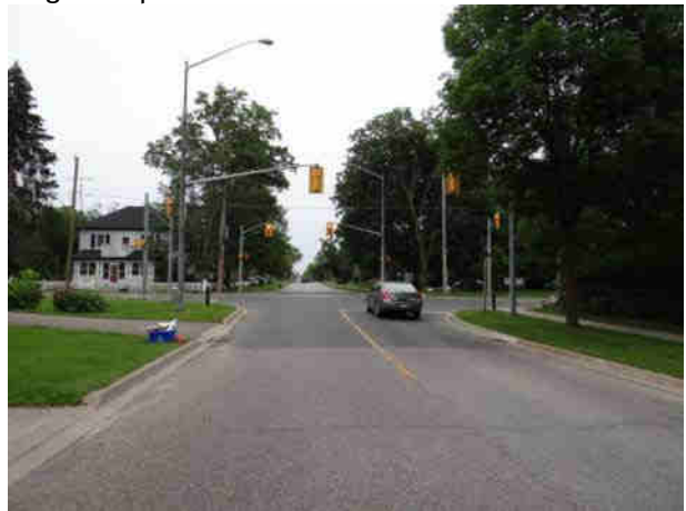
Plate 20: Northeast view of Dundas St W at Main St, Erin; Proposed sewer route and forcemain are within the disturbed road, no Stage 2 required
