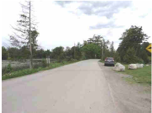
Plate 18: Northeast view of Overland Dr, Erin; Proposed sewer route is within the disturbed road, no Stage 2 required
