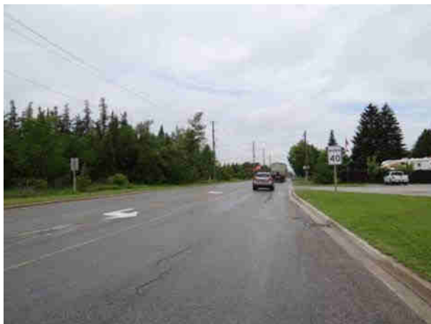
Plate 3: Northwest view of Main St, Hillsburgh; Proposed sewer route is within the disturbed ROW, no Stage 2 required
