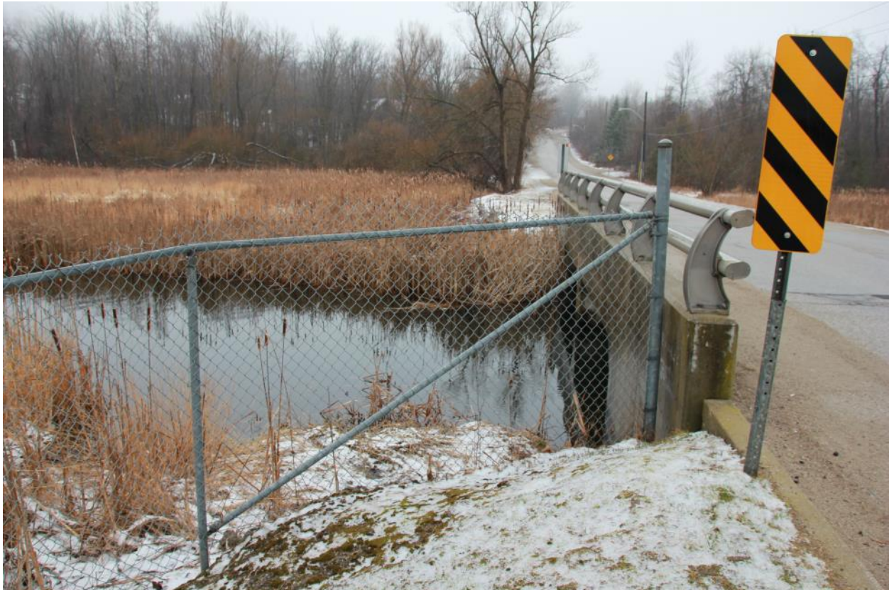
Figure 11 – West Credit River crossing with Dundas Street
