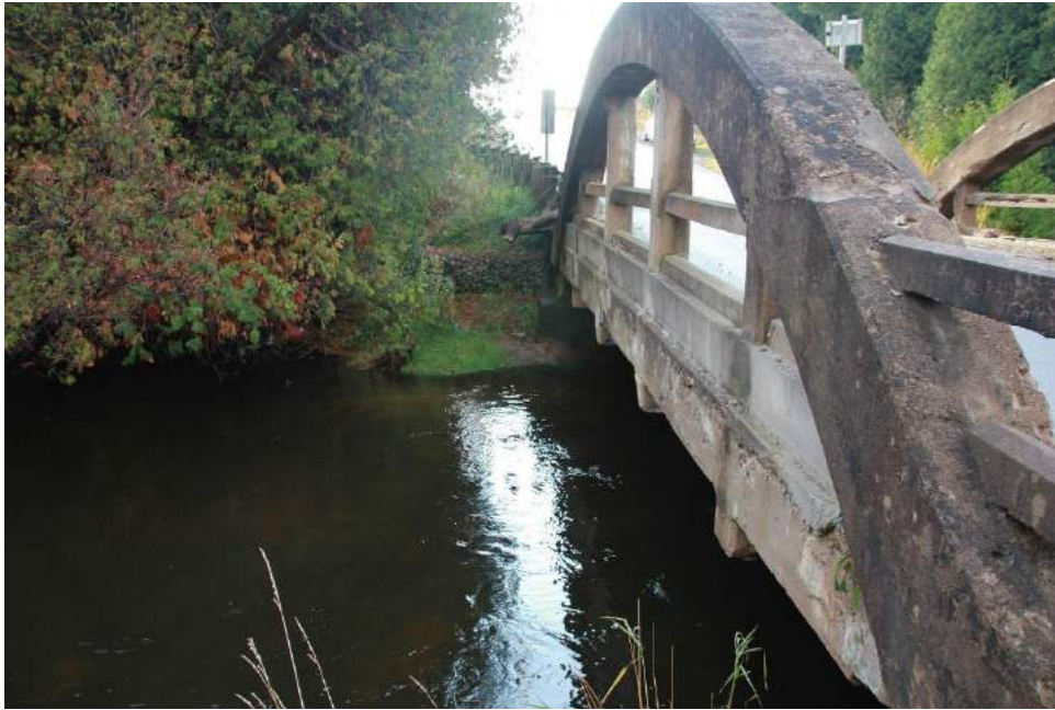
Figure 9 - Alternative 1B Discharge Sewer Outfall Location (Facing South)
