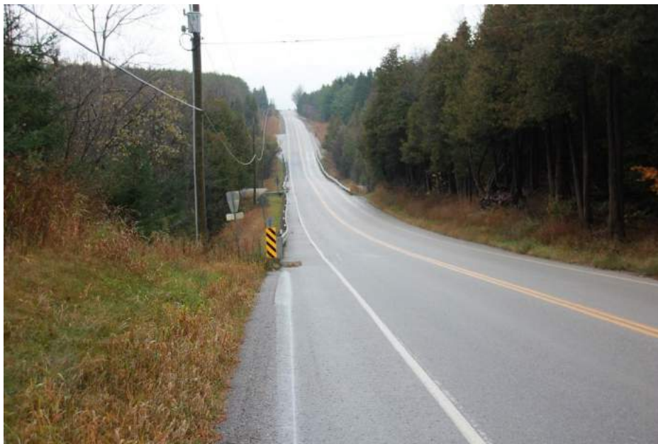
Figure 13 - Facing North on Winston Churchill Blvd towards West Credit River
