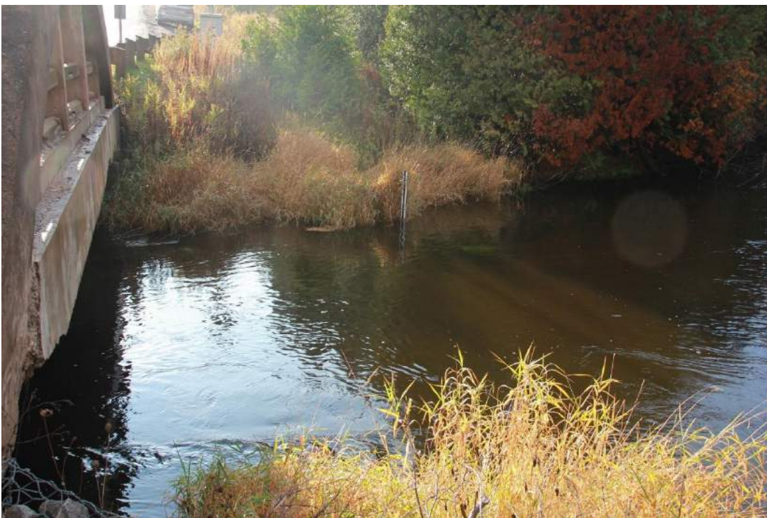
Figure 7 - Outfall Alternative 1A Discharge Location (Facing South)
