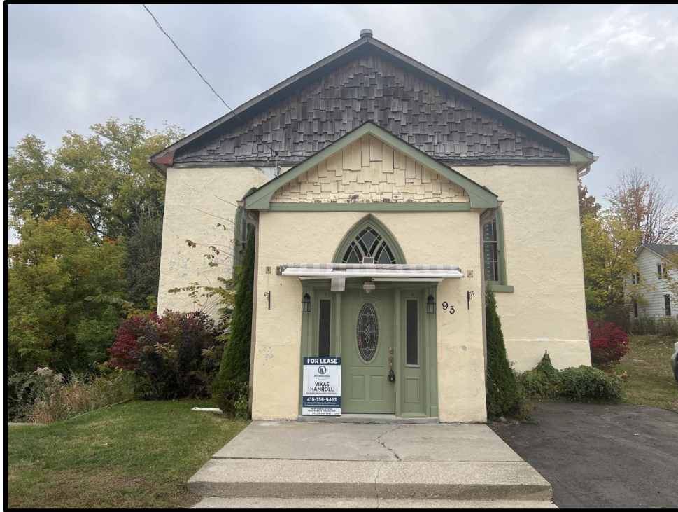
Image 1: Façade of 93 Trafalgar Road (Photo taken October 19, 2023; Facing Northeast)
