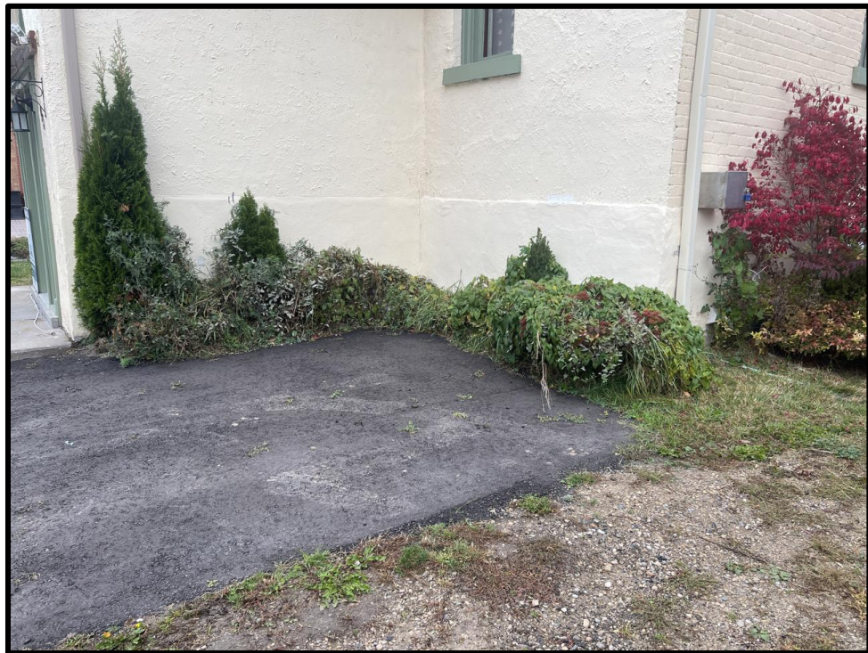
Image 10: Detail of Foundation of 93 Trafalgar Road (Photo taken October 19, 2023; Facing North)
