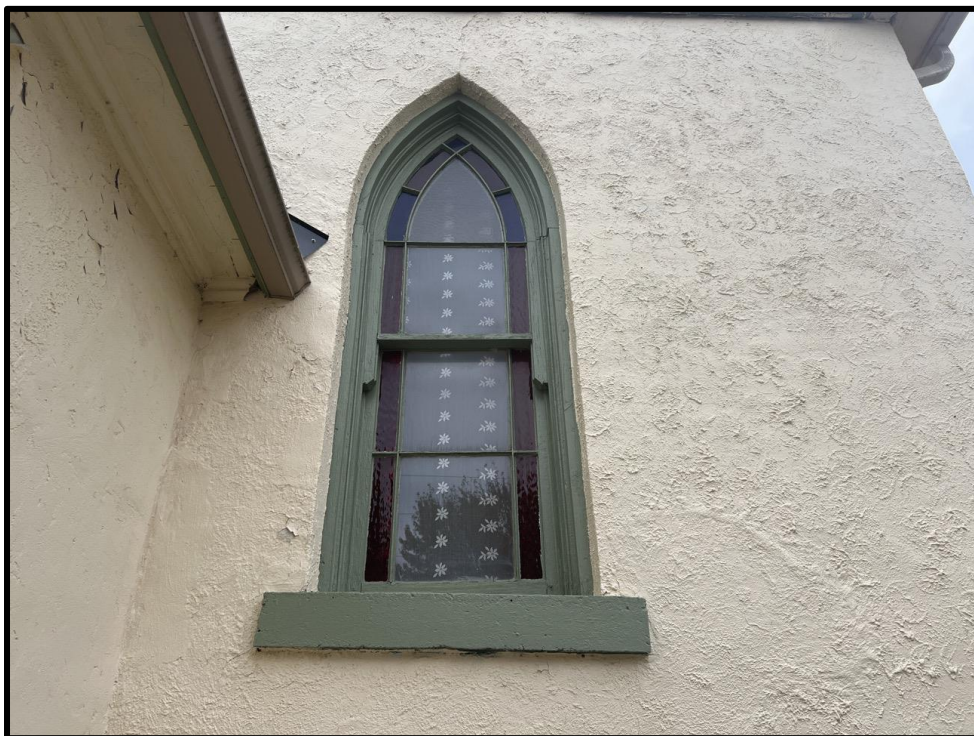
Image 4: Detail of Lancet Window Opening of 93 Trafalgar Road (Photo taken October 19, 2023; Facing Northeast)
