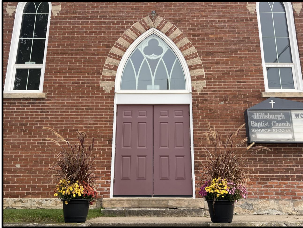
Image 3: Detail of Original Front Door of 21 Trafalgar Road (Photo taken October 19, 2023; Facing Northeast)
