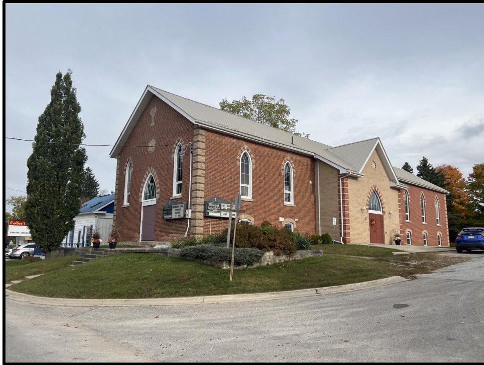
Image 9: South Elevation of 21 Trafalgar Road (Photo taken October 19, 2023; Facing North)
