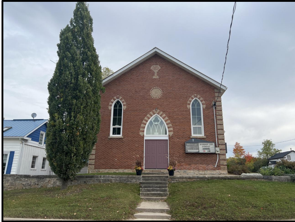
Image 1: Façade of 21 Trafalgar Road (Photo taken October 19, 2023; Facing Northeast)
