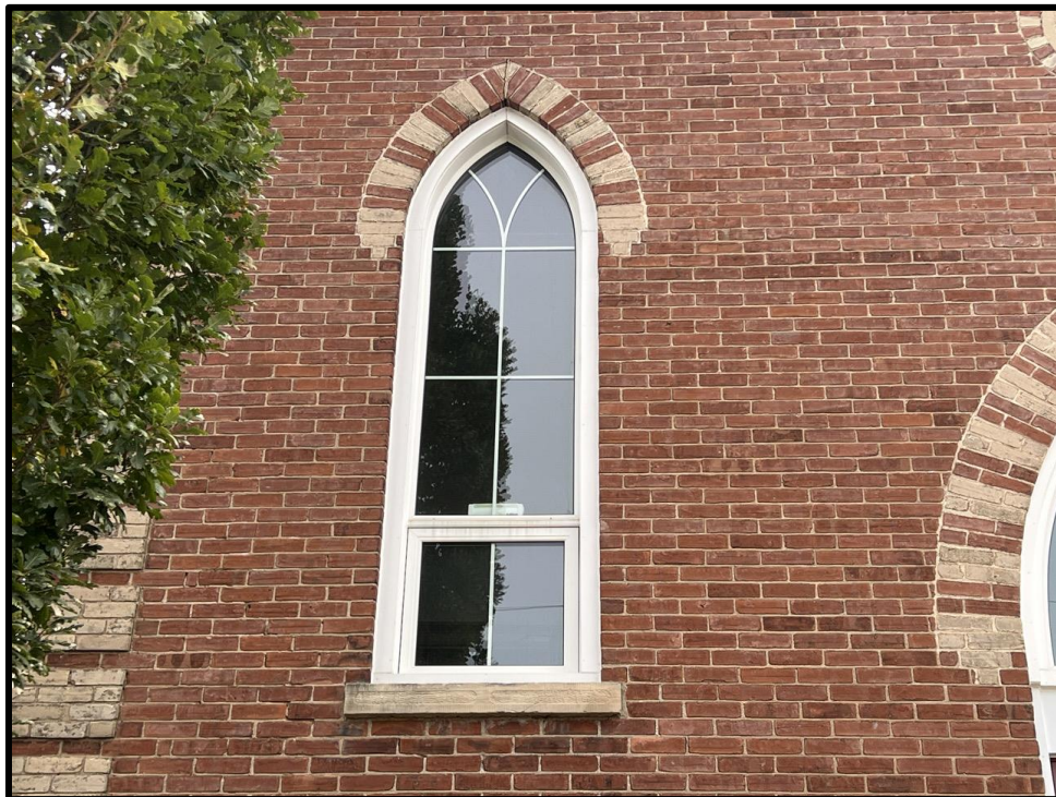
Image 4: Detail of Lancet Window Opening of 21 Trafalgar Road on Original Portion (Photo taken October 19, 2023; Facing Northeast)
