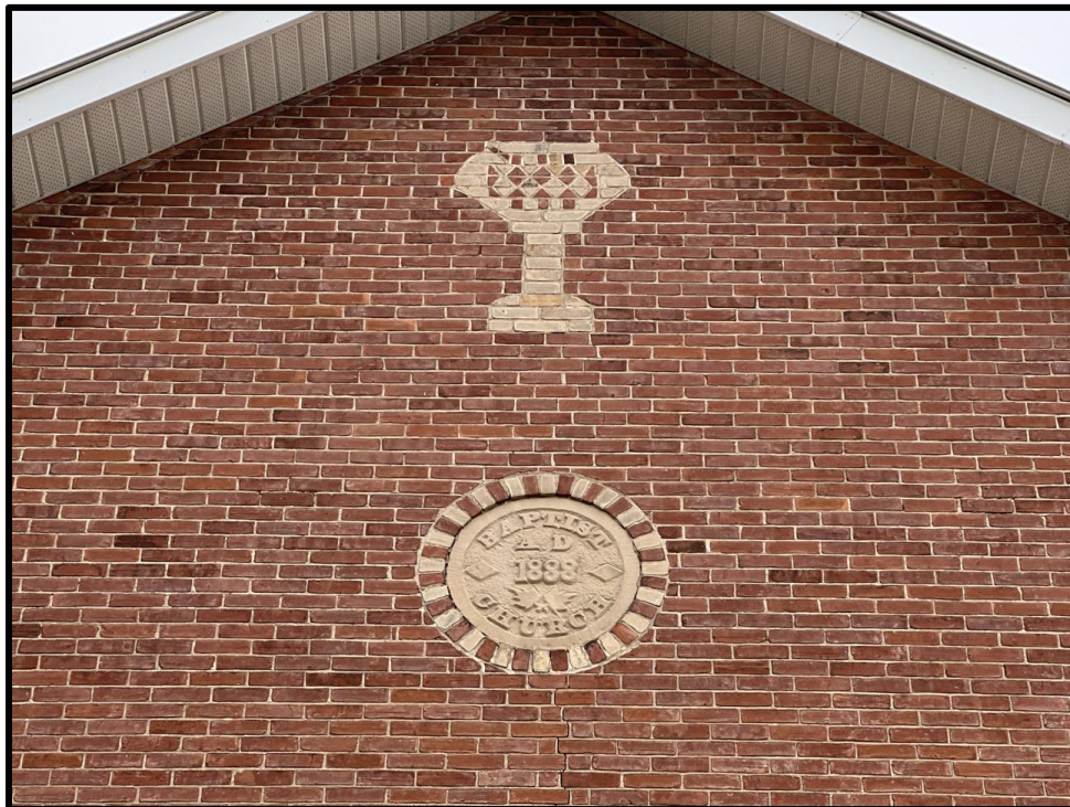
Image 2: Detail of Date Stone and Brick Chalice on Façade of 21 Trafalgar Road (Photo taken October 19, 2023; Facing Northeast)
