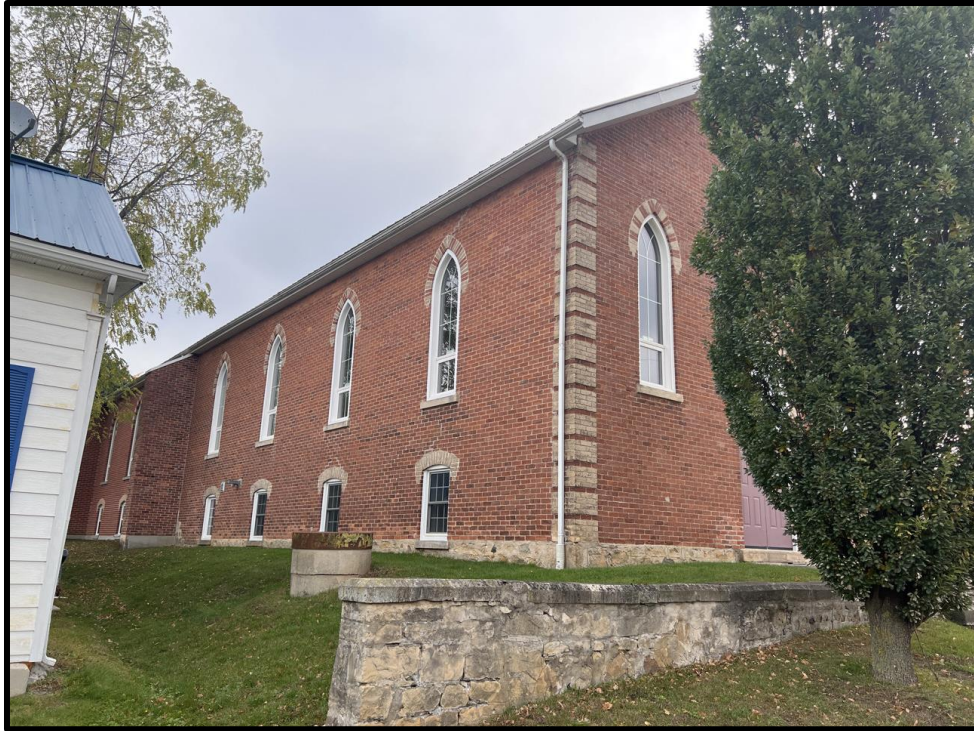
Image 7: Northwest Corner and Retaining Wall of 21 Trafalgar Road (Photo taken on October 19, 2023; Facing Southeast)
