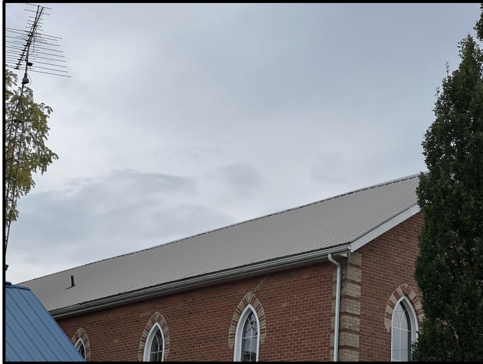
Image 11: Detail of Steel Roof of 21 Trafalgar Road (Photo taken on October 19, 2023; Facing Southeast)
