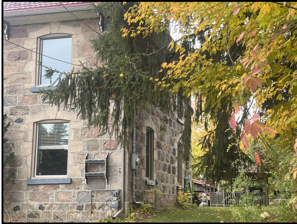
Image 3: Window Detail and North Elevation of 18 Anne Street (Photo taken October 19, 2023; Facing Southwest)
