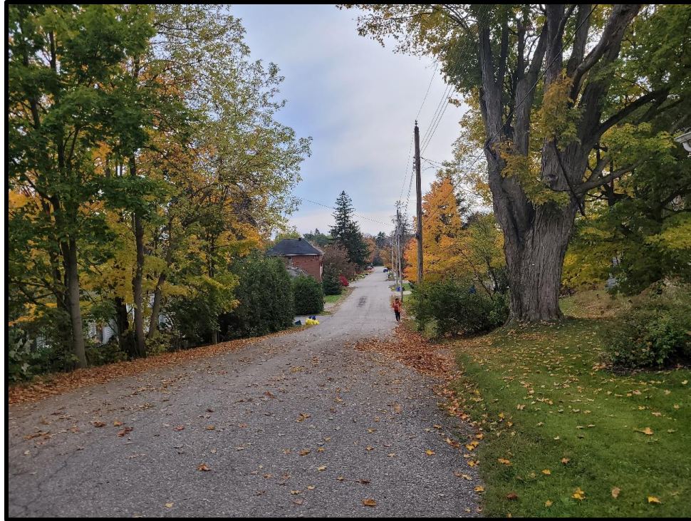
Image 9: Context View of Anne Street Looking South (Photo taken October 19, 2023; Facing Southeast)
