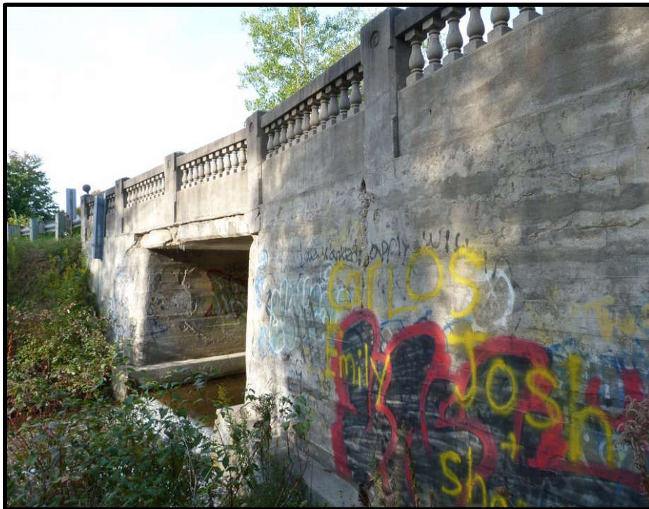
Figure 5: Station Bridge Constructed in 1917 – Replaced in 2020 (Nathan Holth 2022)
