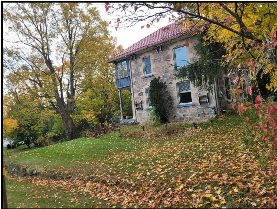
Image 6: View Stone Retaining Wall of 18 Anne Street (Photo taken on October 19, 2023; Facing South)
