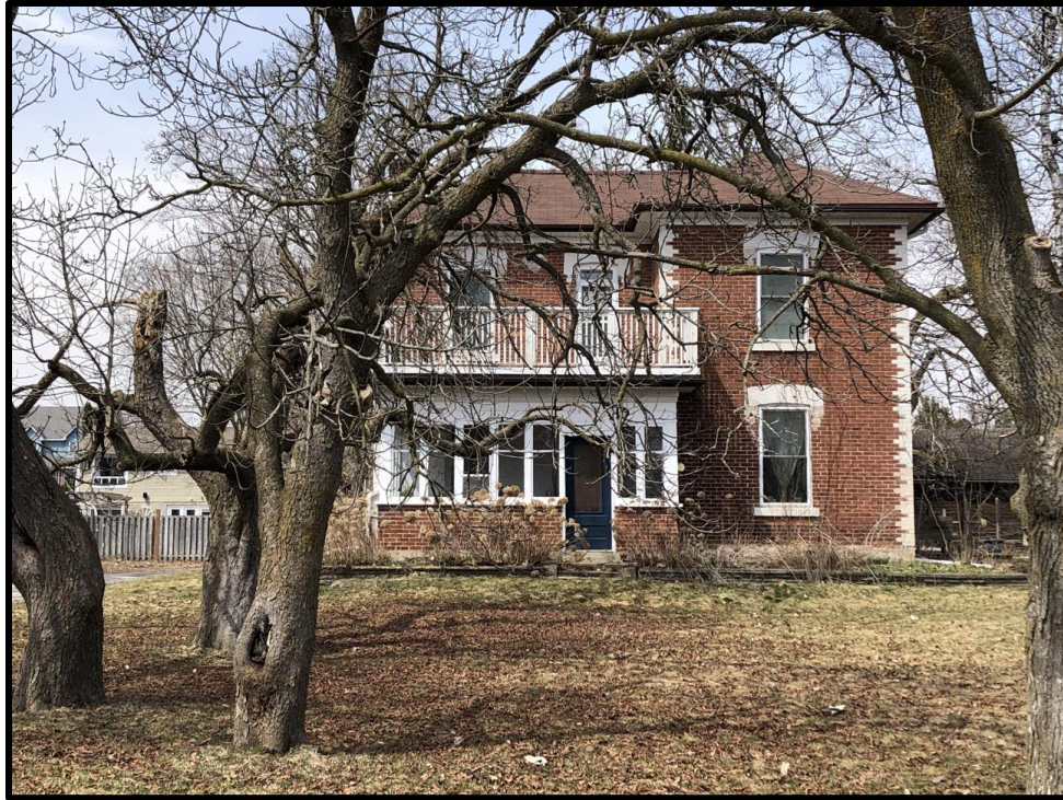
Image 1: Façade of 12 Orangeville Street (Photo taken April 11, 2023; Facing Northwest)
