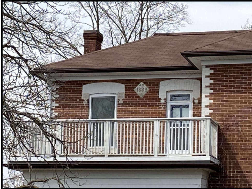
Image 8: Date Stone and Upper Storey Balcony of 12 Orangeville Street (Photo taken on October 19, 2023; Facing North)
