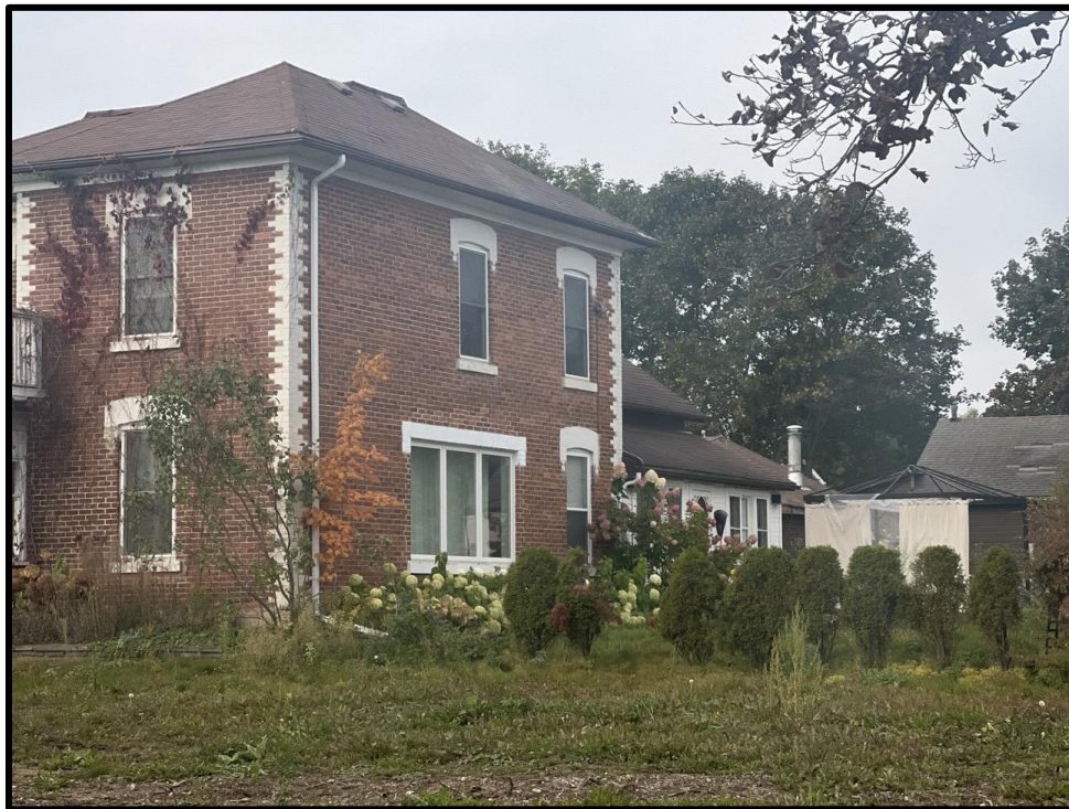
Image 4: View of East Elevation and Rear Addition of 12 Orangeville Street (Photo taken October 19, 2023; Facing Northwest)
