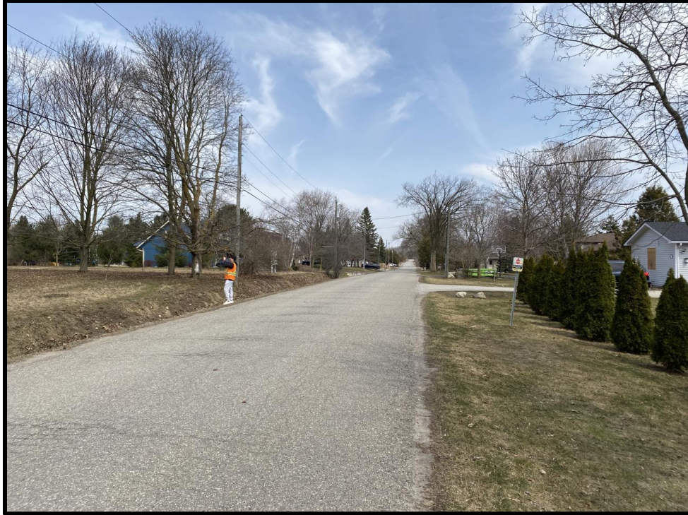
Image 11: View of Orangeville Street (Photo taken on April 11, 2023; Facing Northeast)
