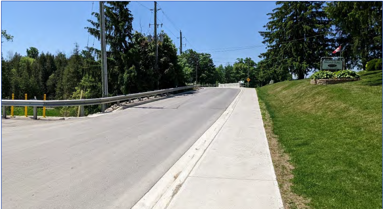
Figure 21: View southwest along Station Street from the sidewalk on the west side of Station Street
