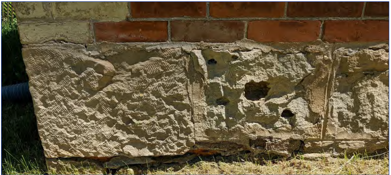
Figure 34: View of the foundation
