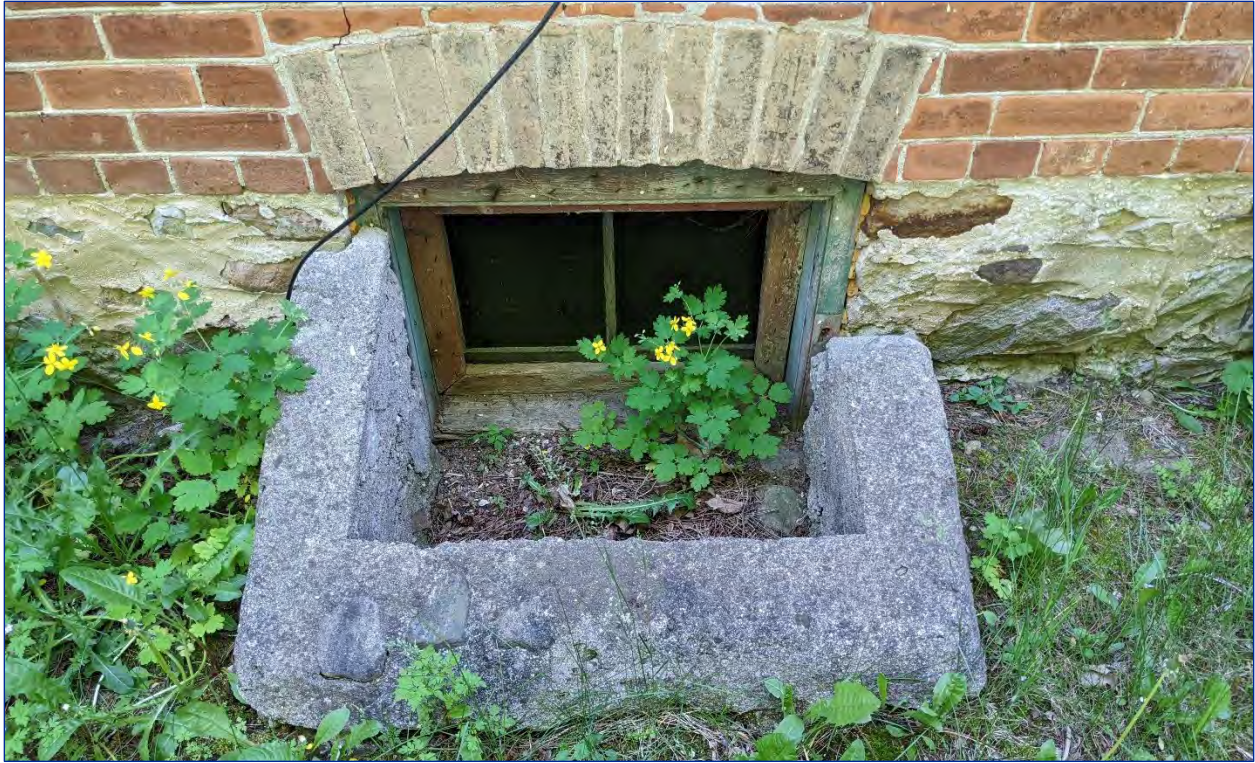
Figure 37: Detail image of the basement windows
