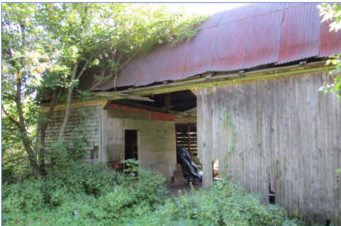
Figure 5: Image of the former drive shed 76
