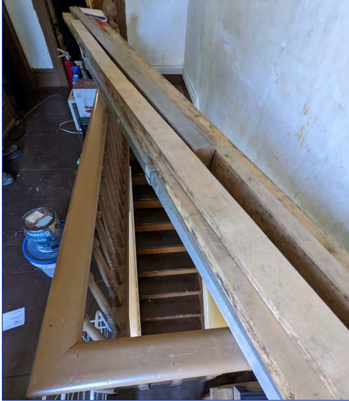
Figure 47: View of the second storey landing
