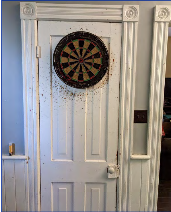
Figure 43: View of the basement door
