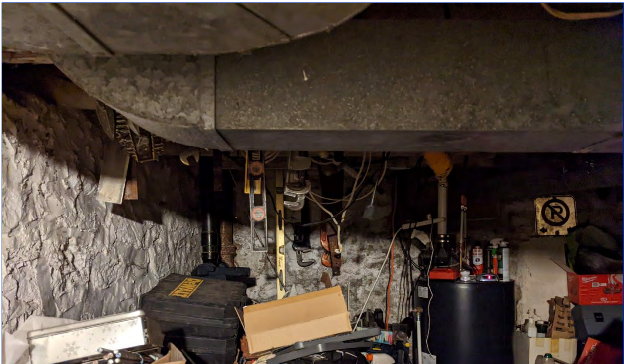
Figure 46: View of the north half of the basement
