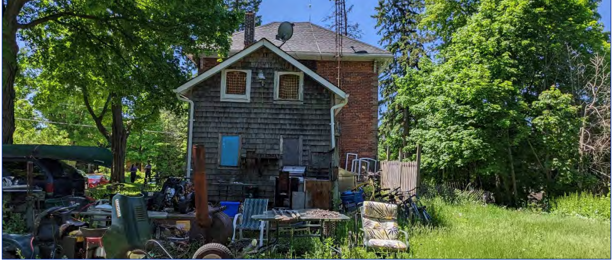
Figure 31: View of the north elevation
