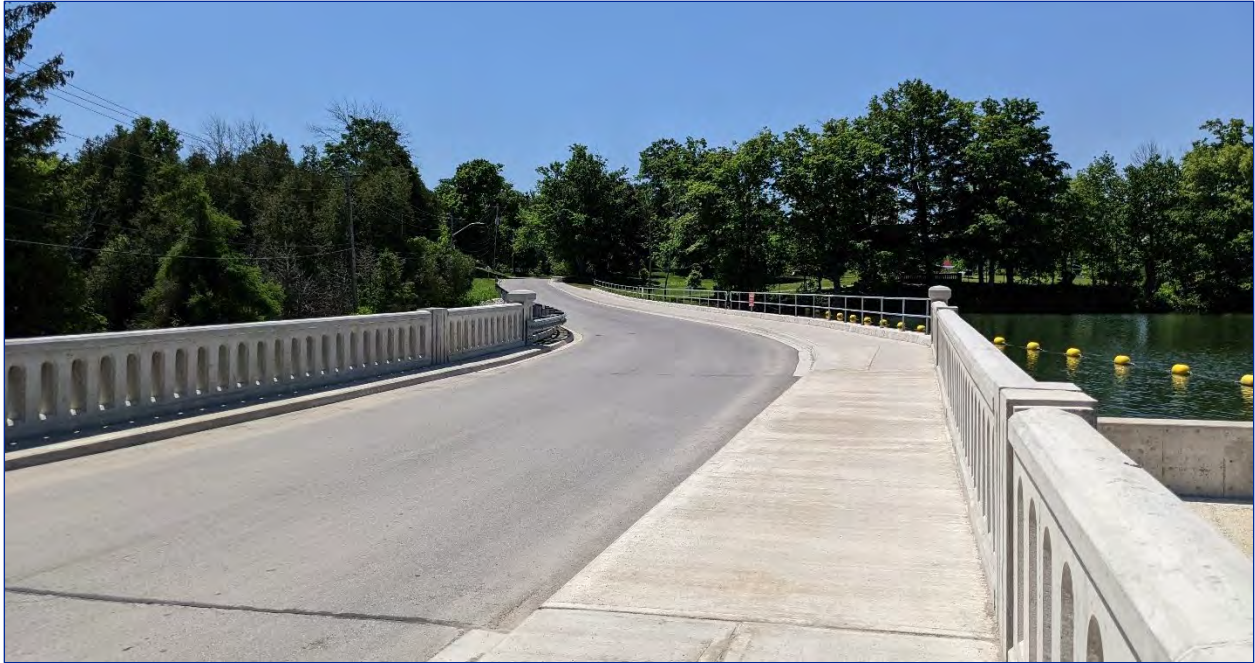
Figure 22: View south along Station Street from the Station Street bridge
