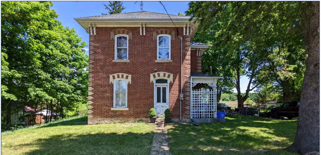
Figure 28: View of the south elevation
