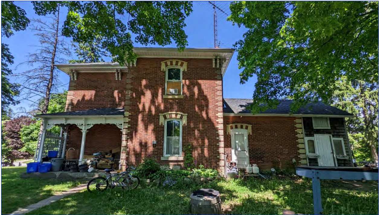
Figure 32: View of the east elevation
