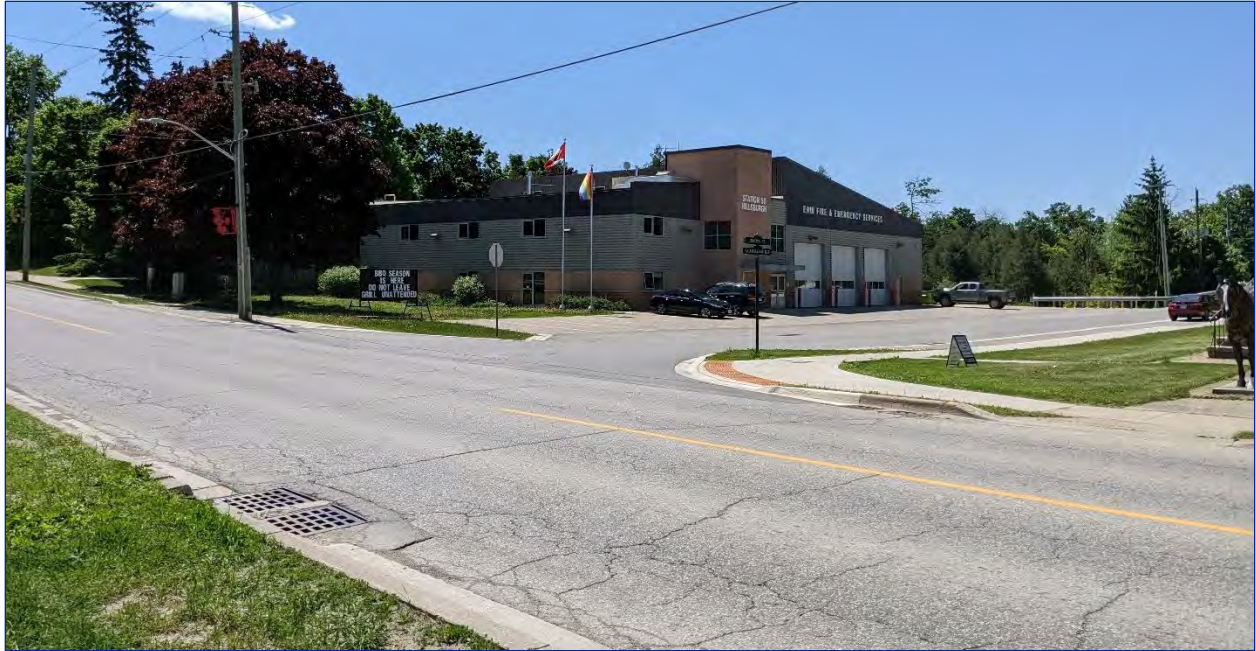
Figure 20: View south of the intersection of Trafalgar Road and Station Street from in front of 71 Trafalgar Road
