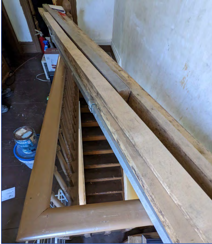
Figure 47: View of the second storey landing
