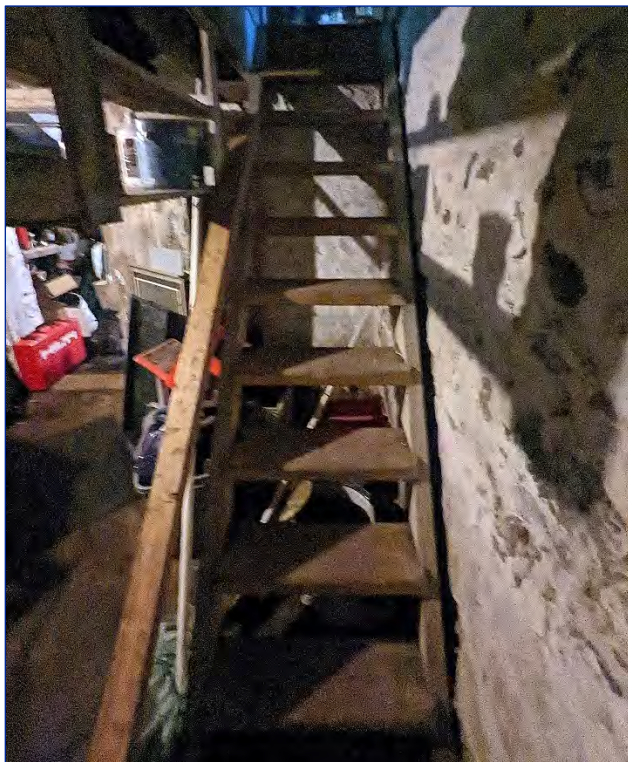
Figure 44: View of the basement stairs
