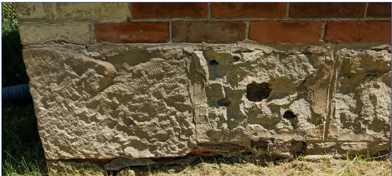
Figure 34: View of the foundation
