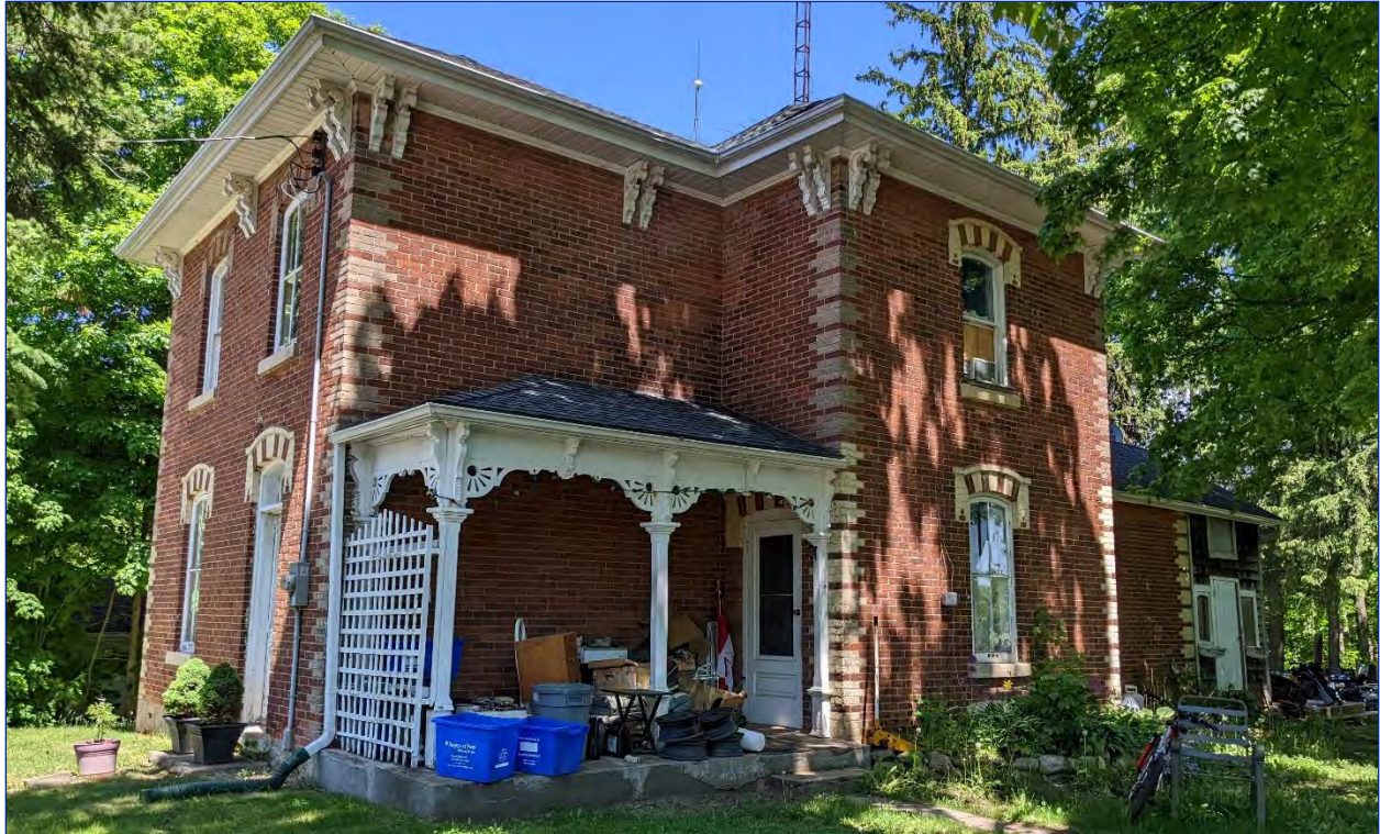
Figure 33: View of the south and east elevations
