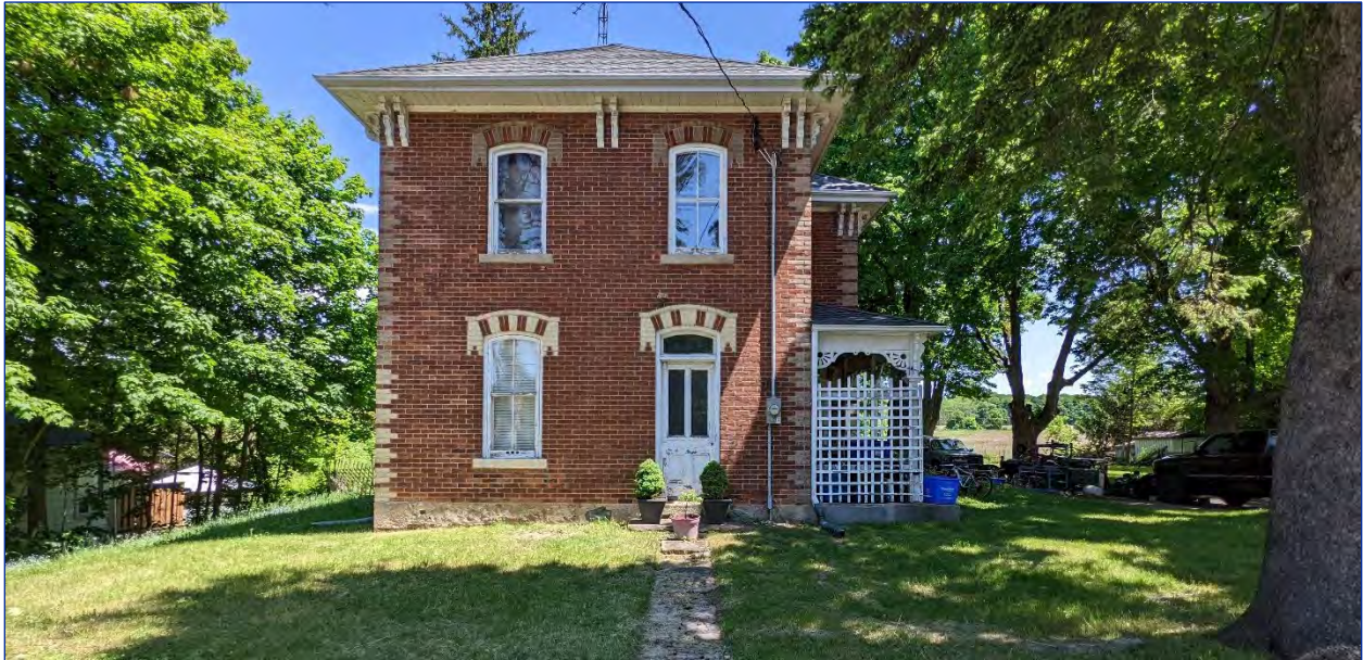
Figure 28: View of the south elevation
