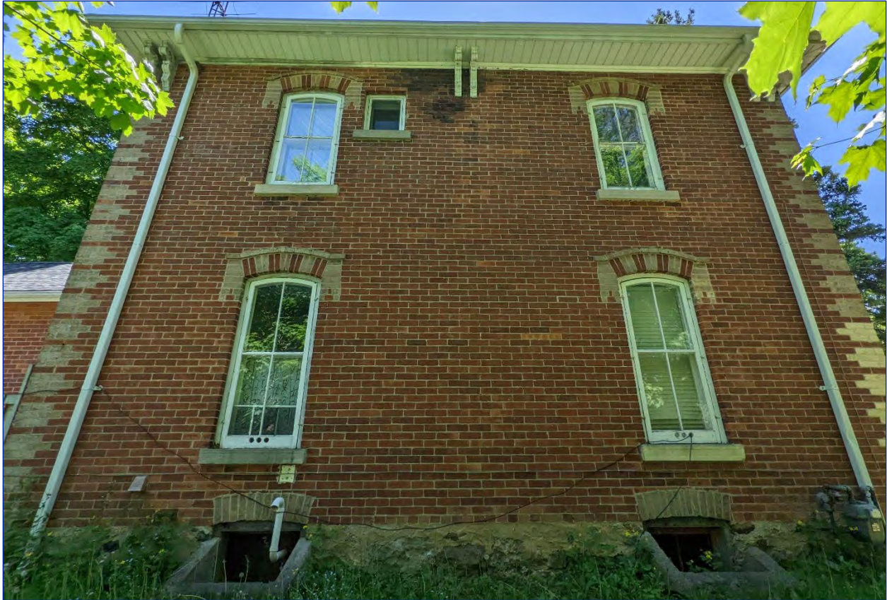
Figure 29: View of the west elevation of the main building
