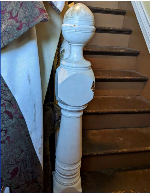
Figure 39: Detailed view of the staircase to the second storey
