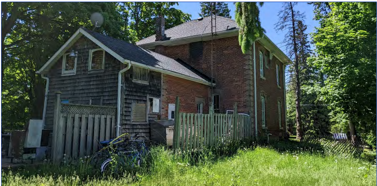
Figure 30: View of the west and north elevations
