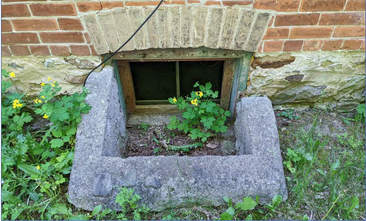
Figure 37: Detail image of the basement windows
