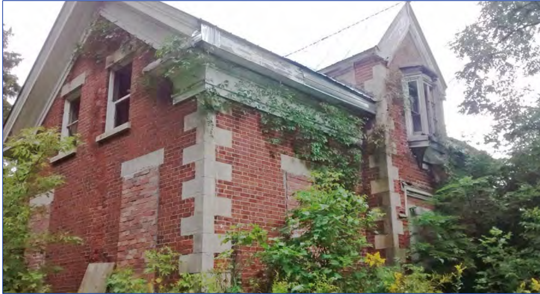
Figure 4: Image of the 1860s Nodwell House before its demolition in 2019 75
