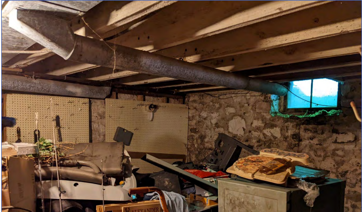
Figure 45: View of the south half of the basement
