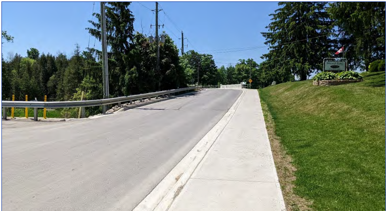
Figure 21: View southwest along Station Street from the sidewalk on the west side of Station Street
