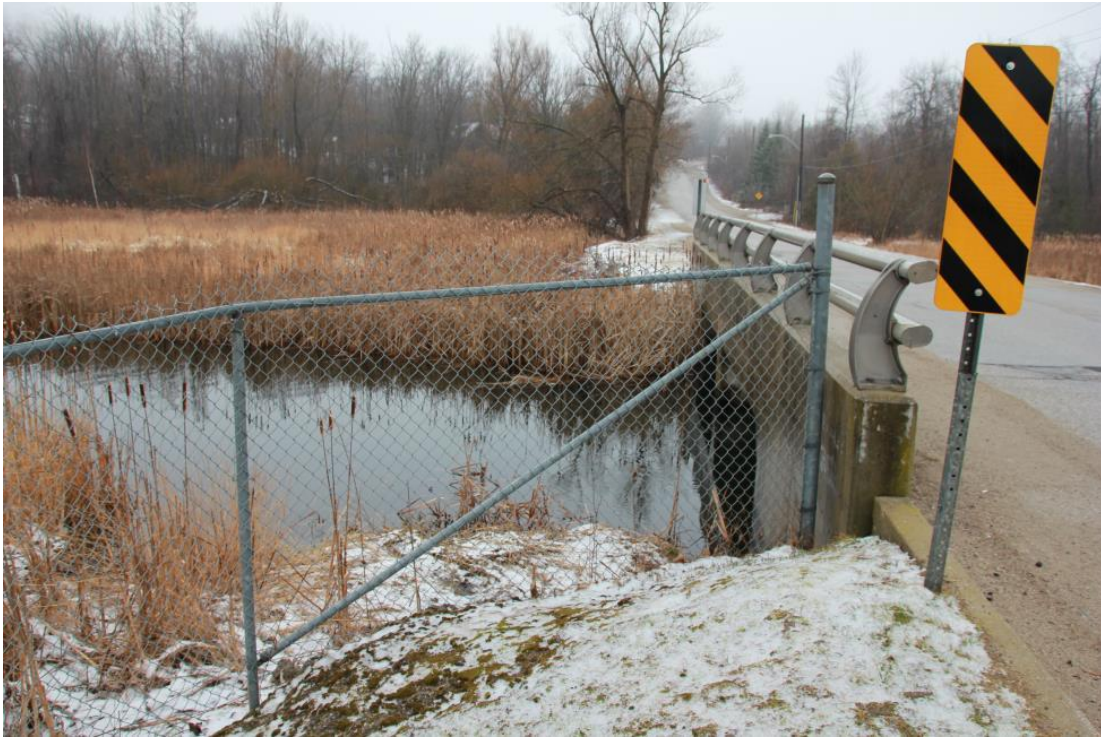
Figure 11 – West Credit River crossing with Dundas Street
