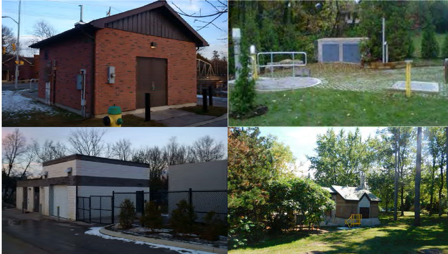
The architecture of a pumping station can be designed to suit the surrounding area.
