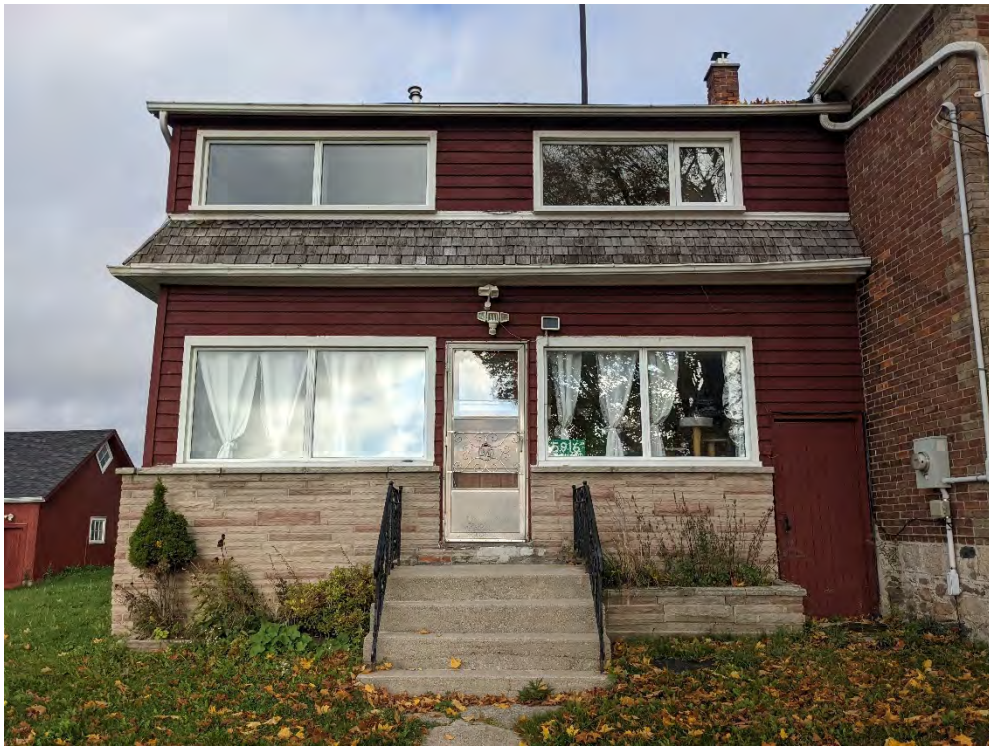
Figure 61: The south elevation of the south addition, note entrance to basement (Right)
