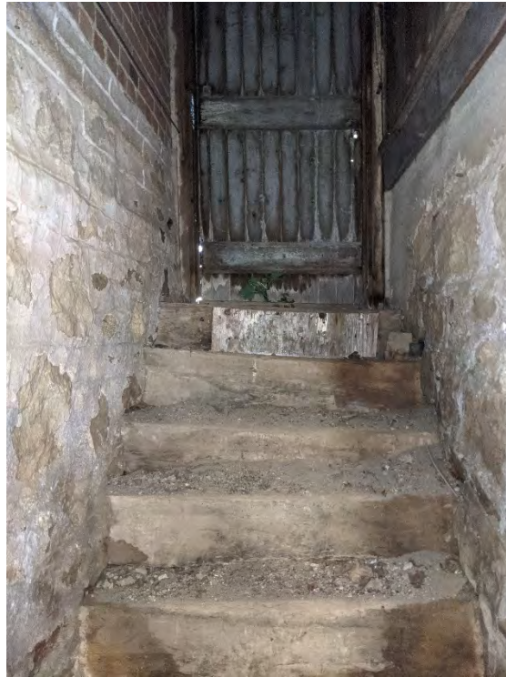
Figure 52: Stone steps from the entrance off the south addition
