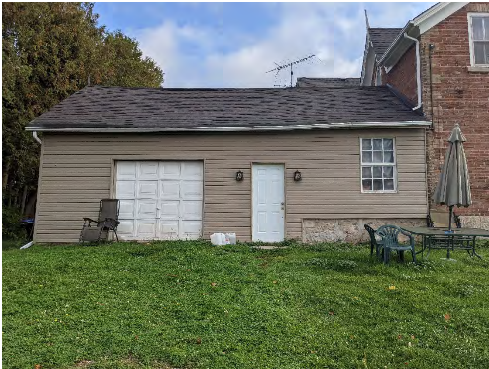
Figure 55: West elevation of the north addition
