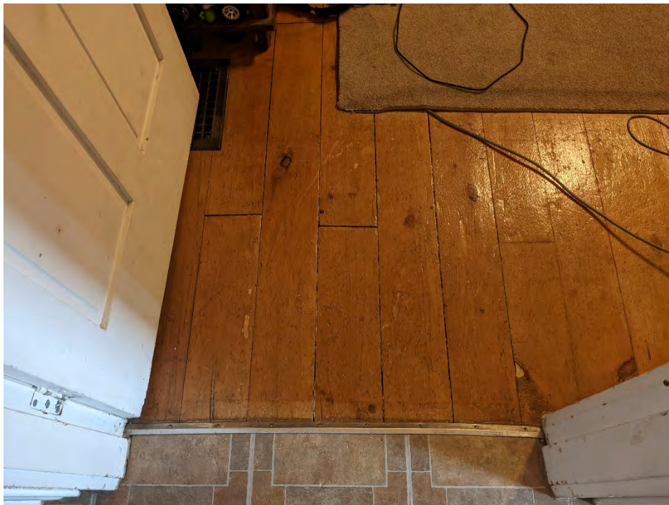
Figure 30: Pine wood floors in north front room
