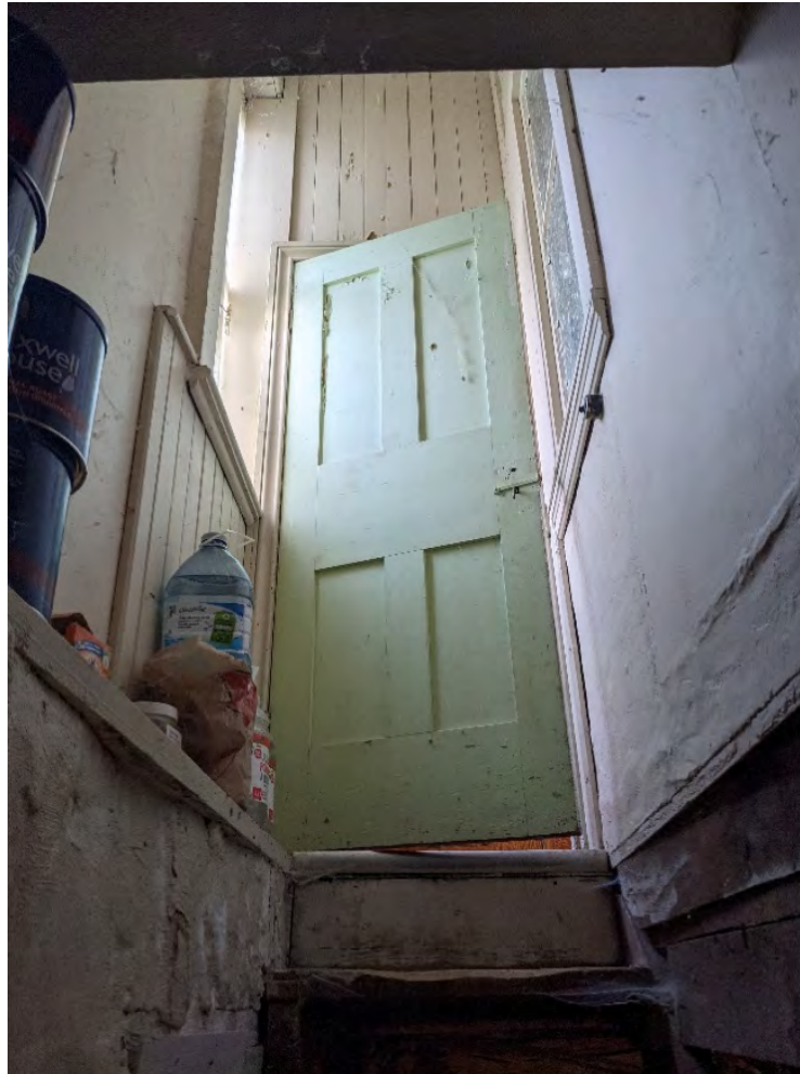
Figure 51: The door from the kitchen, view from the basement stairs
