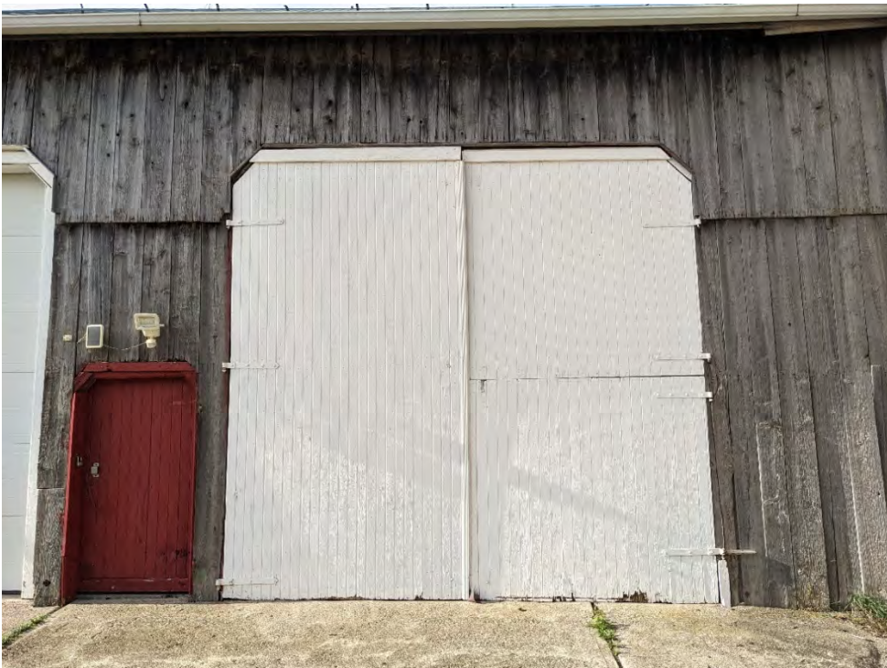
Figure 75: Large door on east elevation of the large barn
