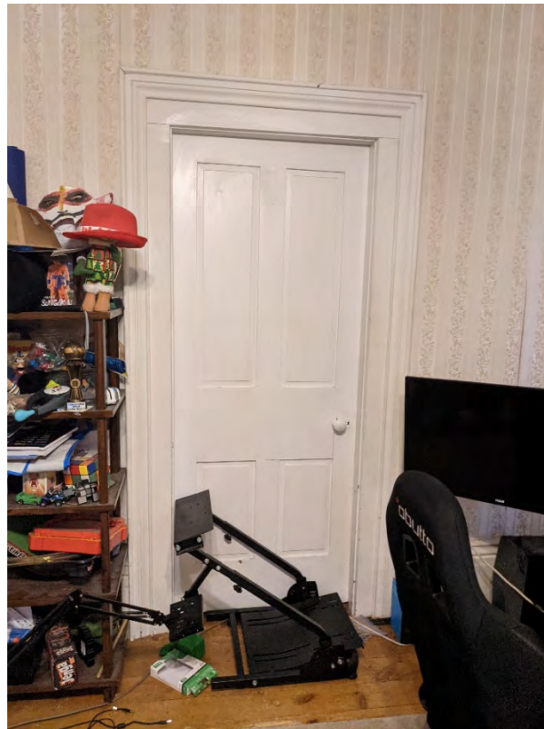
Figure 31: Four paneled door in north front room
