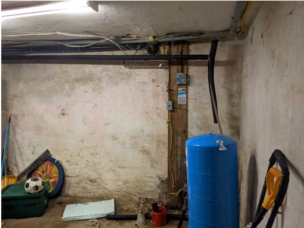
Figure 54: Wood support column
