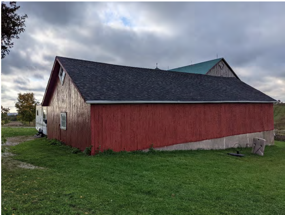
Figure 68: North façade of the driveshed
