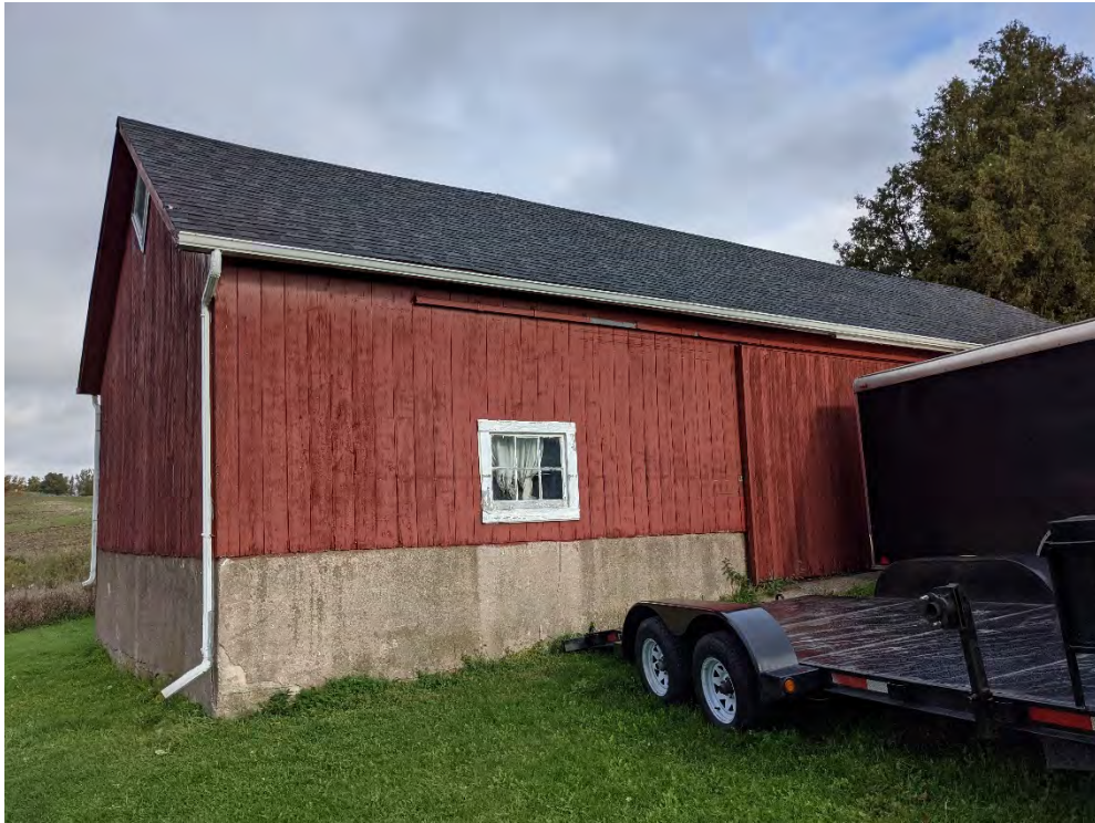
Figure 67: The sliding door entrance on the south façade of the driveshed
