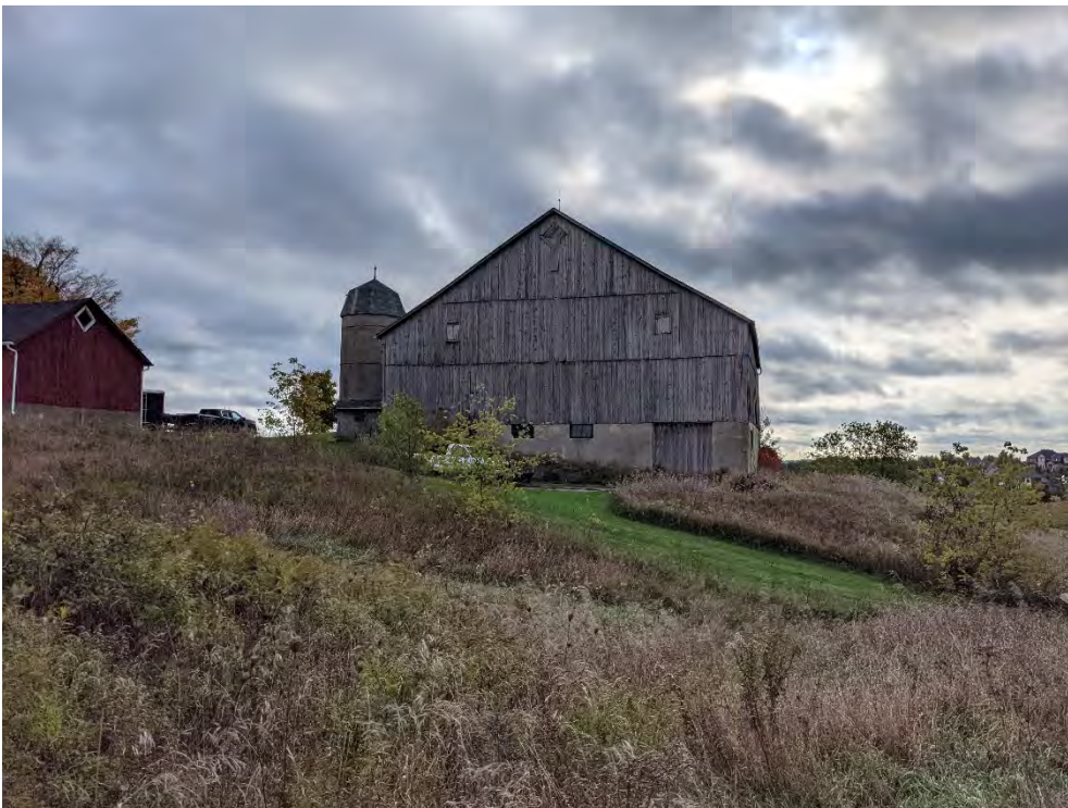
Figure 79: South façade of the large barn
