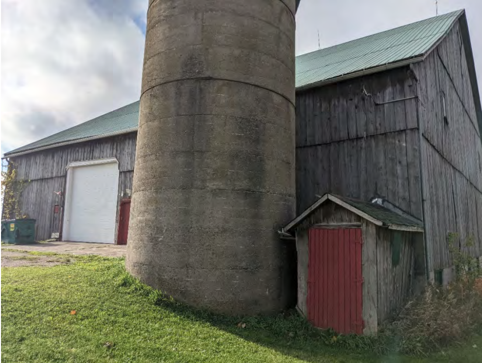
Figure 74: East elevation of the large barn
