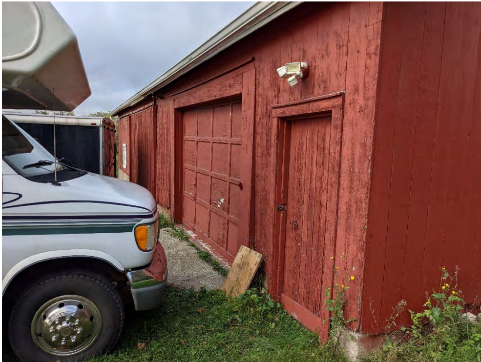
Figure 66: South façade of the driveshed
