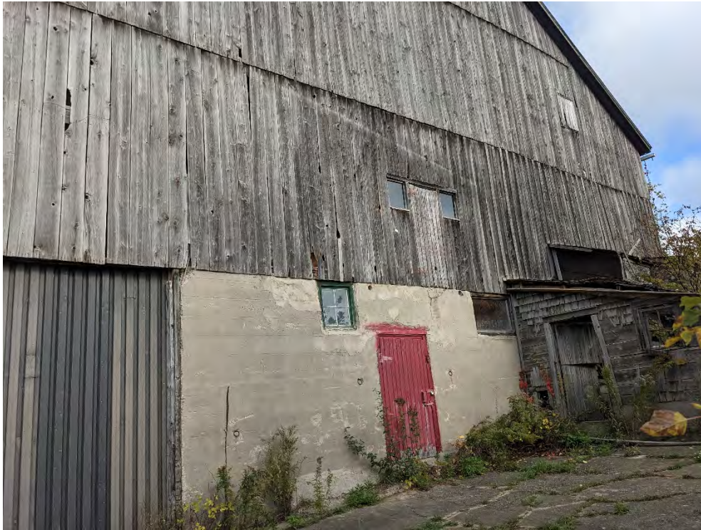
Figure 80: Lower level of the south façade of the large barn
