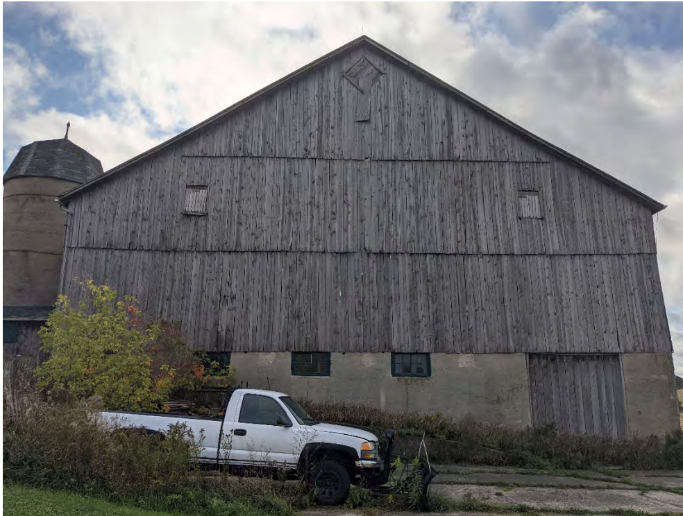
Figure 76: North elevation of large barn
