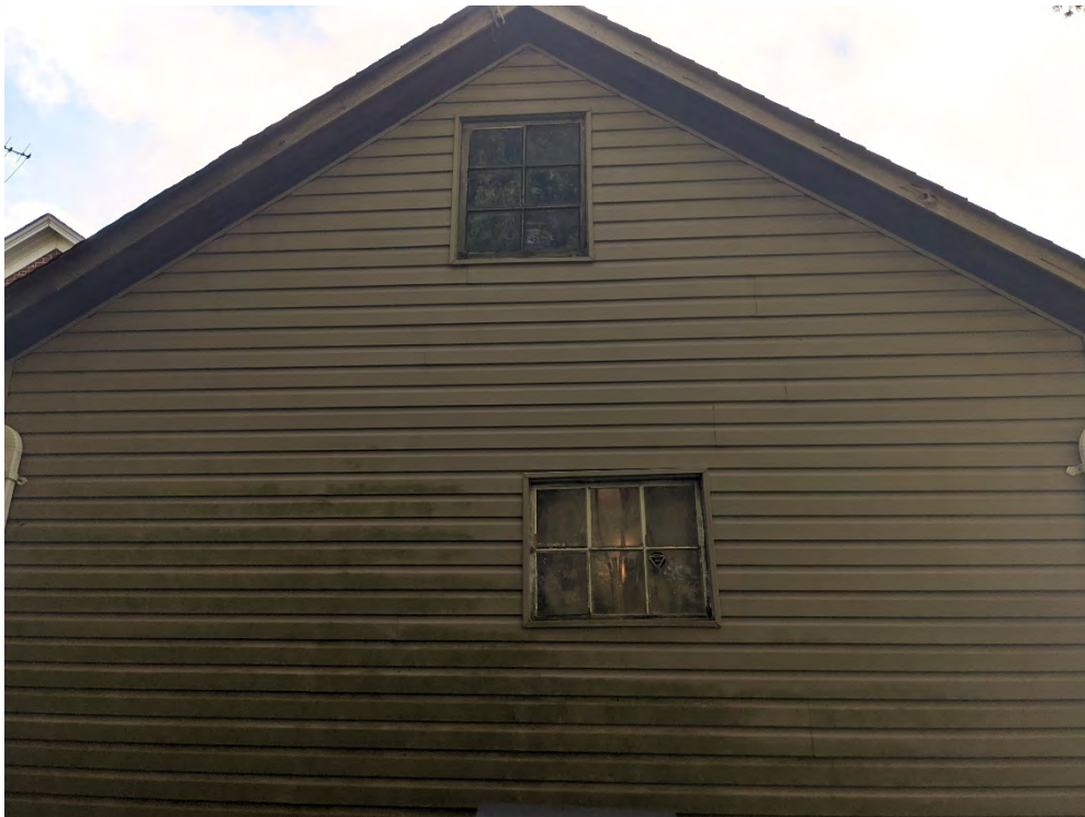
Figure 58: North elevation of the north addition
