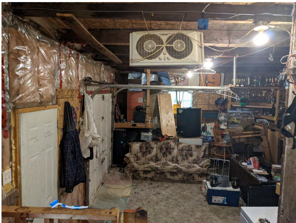
Figure 60: Interior of north addition, facing north
