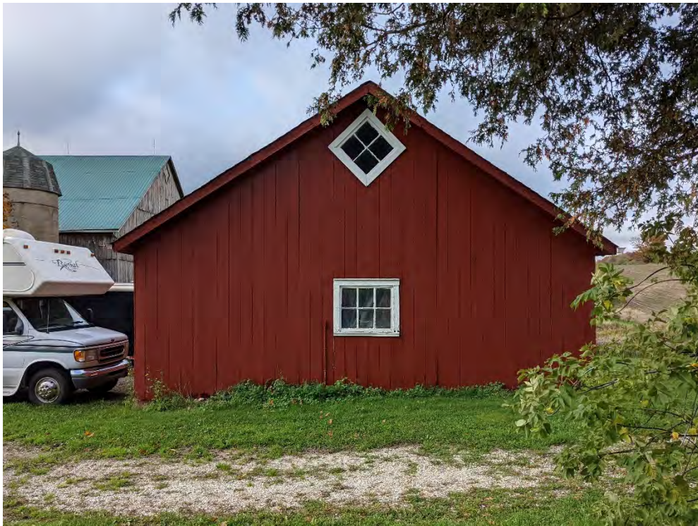
Figure 69: East elevation of the driveshed
