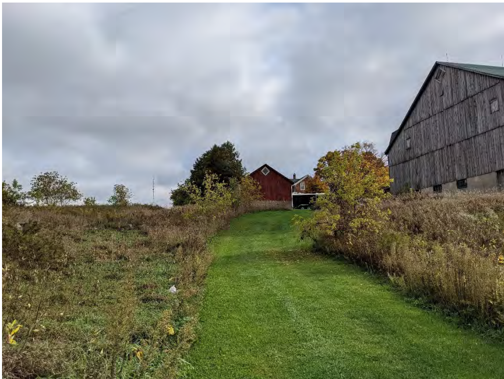
Figure 12: View looking east towards a circulation path behind the driveshed.
