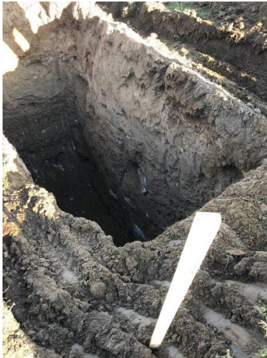
Photograph 11- View of excavation for TP11.
