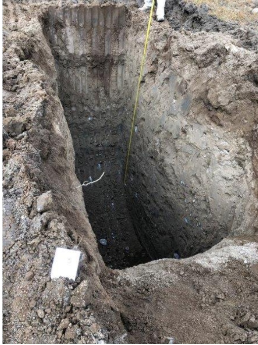
Photograph 3- View of excavation for TP3.
