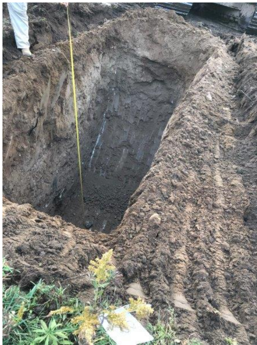
Photograph 8- View of excavation for TP8.
