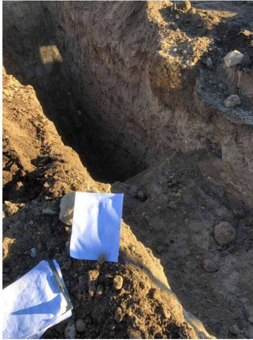
Photograph 9- View of excavation for TP9.
