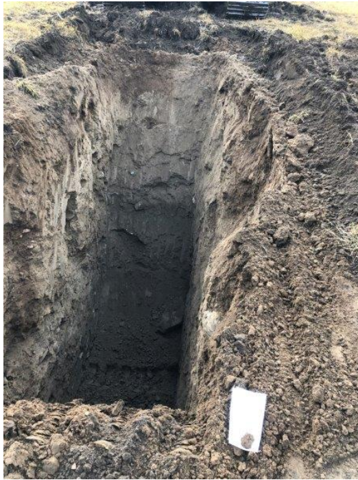
Photograph 6- View of excavation for TP6.
