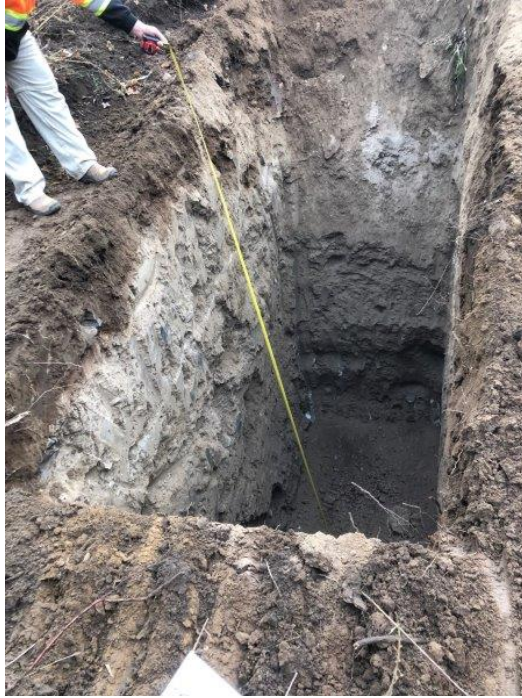
Photograph 7- View of excavation for TP7.
