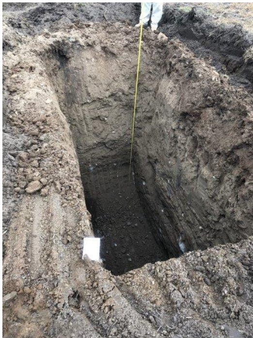
Photograph 2 – View of excavation for TP2.
