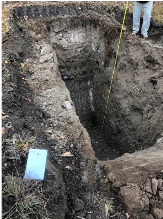
Photograph 4 – View of excavation for TP4.
