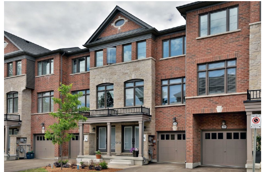
Townhouse block composition should provide massing and design continuity while achieving variety in architectural details.
