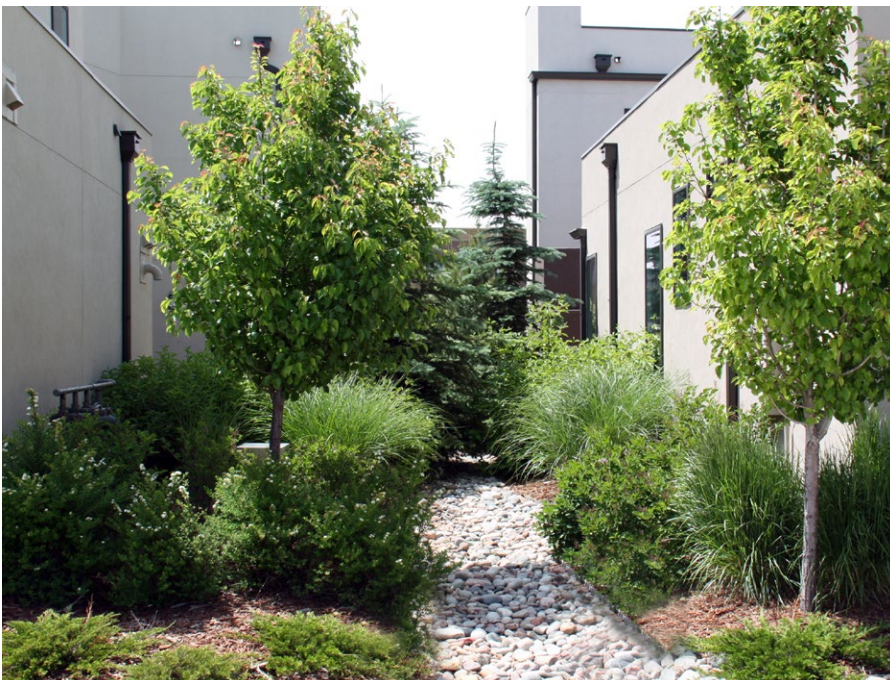
Roof downspouts help direct excess water into soakaway pits. Paired with xeriscape planting, the combination performs well in urban environments due to low-maintenance requirements.
