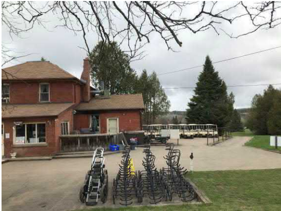
Picture 1: View of the south side of the clubhouse, facing north
