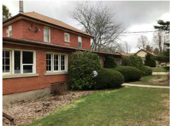
Picture 2: View of the west side of the clubhouse, facing southwest
