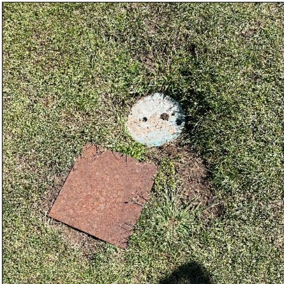
Image 19: Example of in-ground utility.
