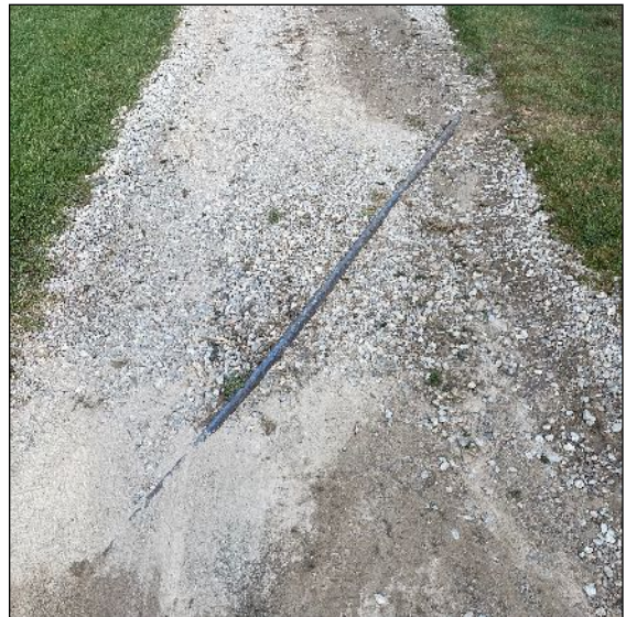
Image 20: Example of in-ground utility.
