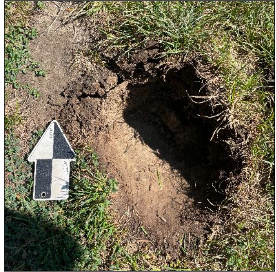
Image 22: Example of disturbed soil conditions.
