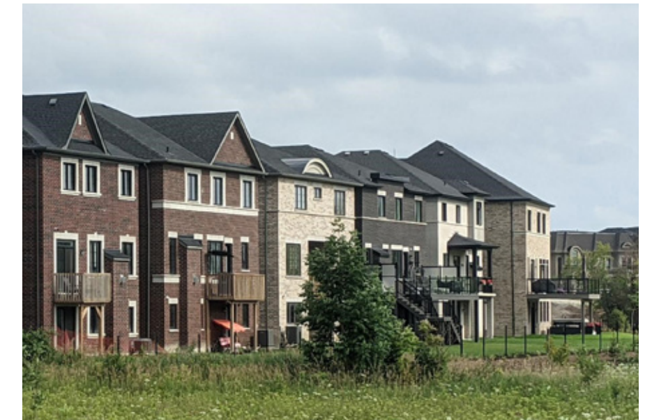
Figure 4.15: Image example of residential dwellings with rear upgrades.
