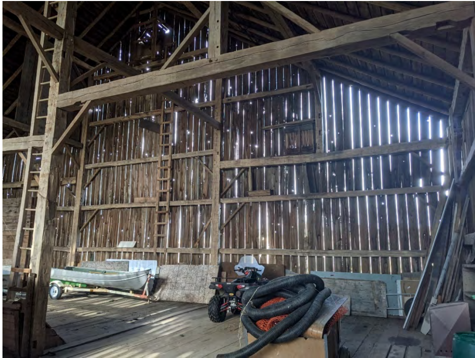
Figure 79: View of the timber frame construction
