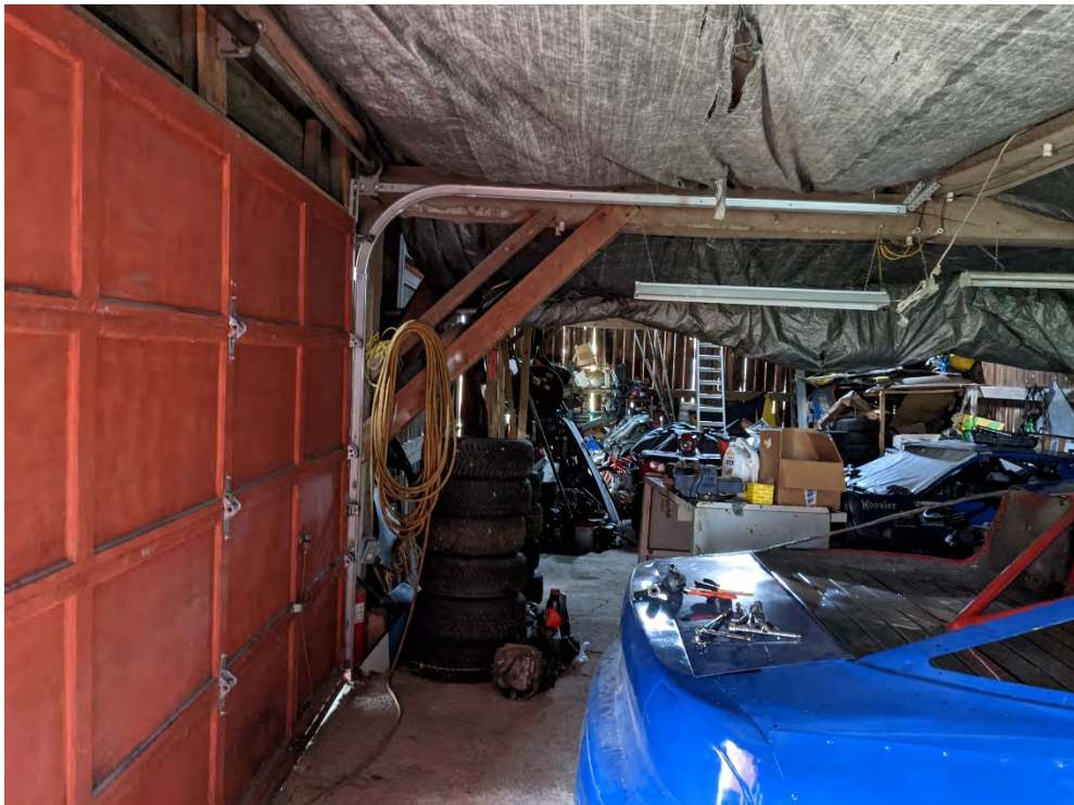
Figure 68: Interior of driveshed, facing west
