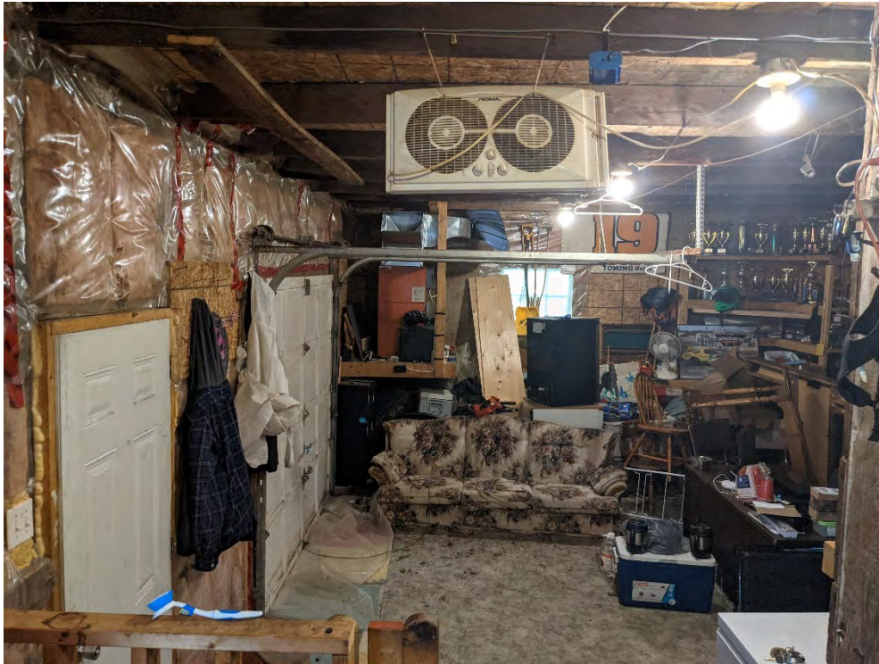
Figure 57: Interior of north addition, facing north
