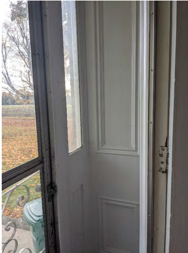
Figure 22: Wood paneling between exterior door and interior door.
