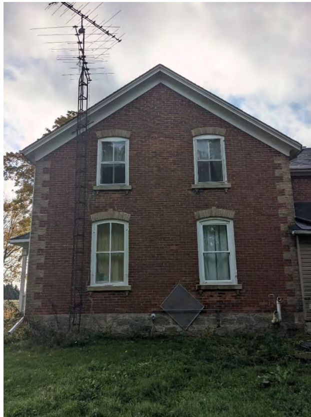
Figure 11: North façade of the Farmhouse's main block
