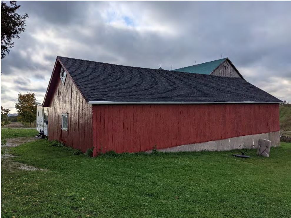
Figure 65: North façade of the driveshed
