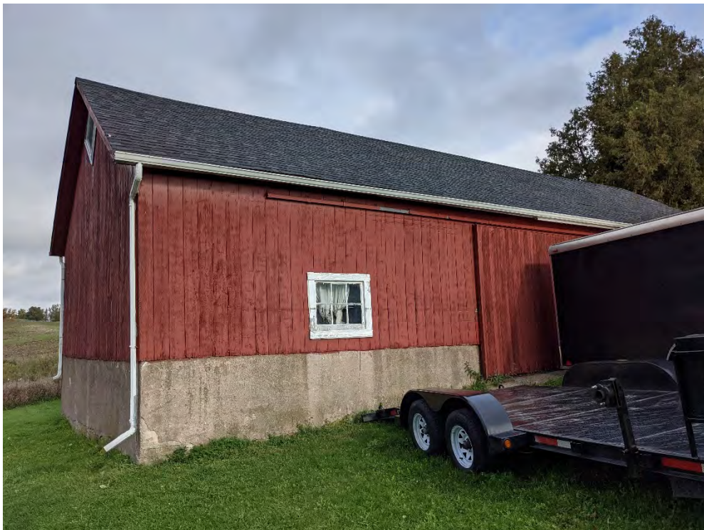
Figure 64: The sliding door entrance on the south façade of the driveshed
