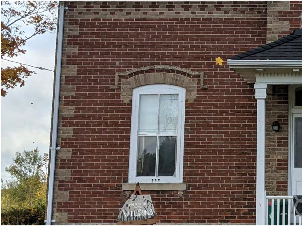
Figure 19: Two-over-two double hung sash window with wood storm door on east façade
