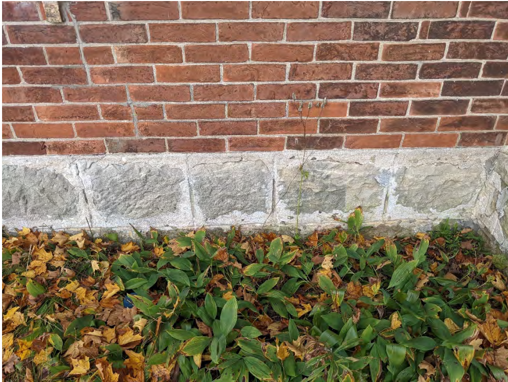
Figure 15: Tooled stone foundation and running bond brick on the east façade
