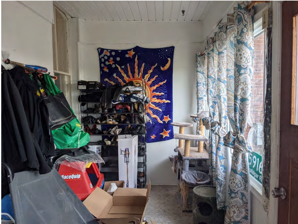
Figure 60: View of the first floor inside the south addition, facing east from the door
