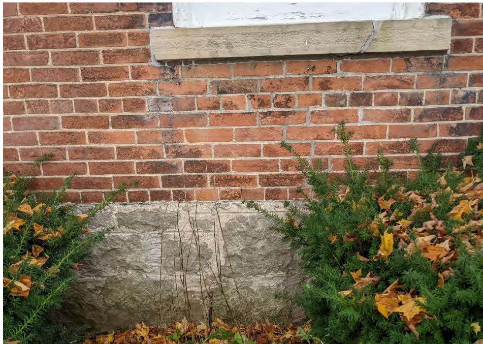
Figure 16: Stone foundation and common bond brick on south elevation.
