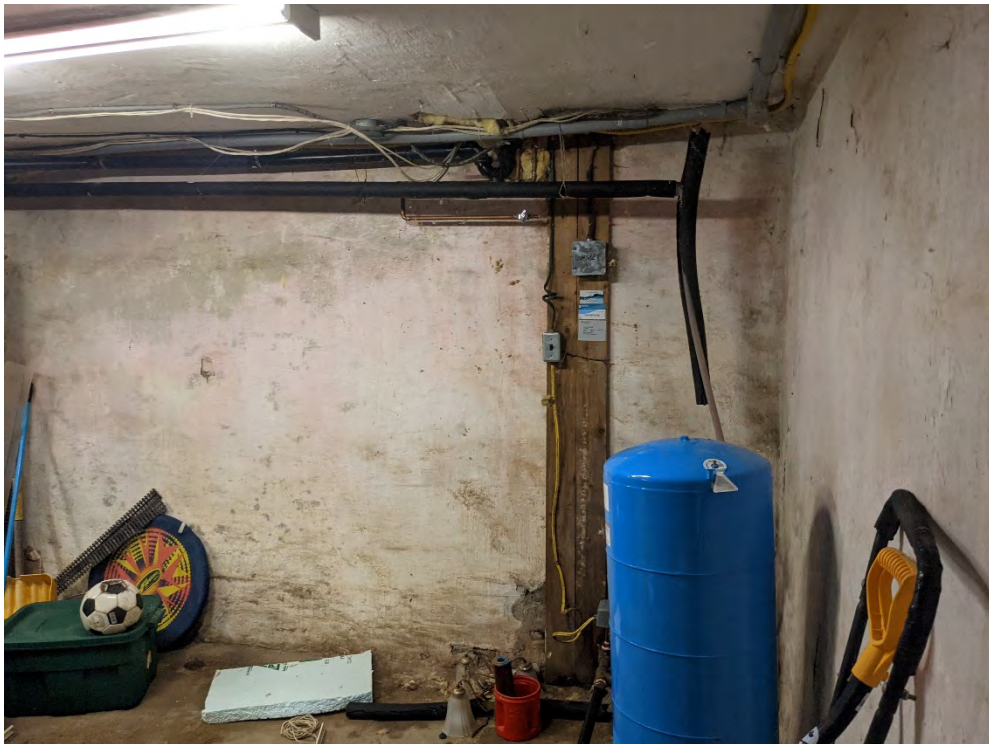
Figure 51: Wood support column
