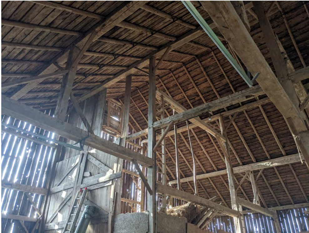
Figure 81: View of the roof rafters inside the large barn
