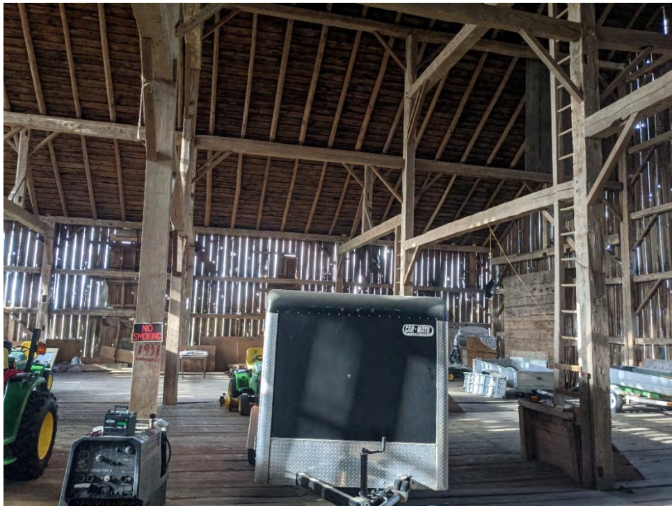
Figure 80: View of threshing floor inside the large barn
