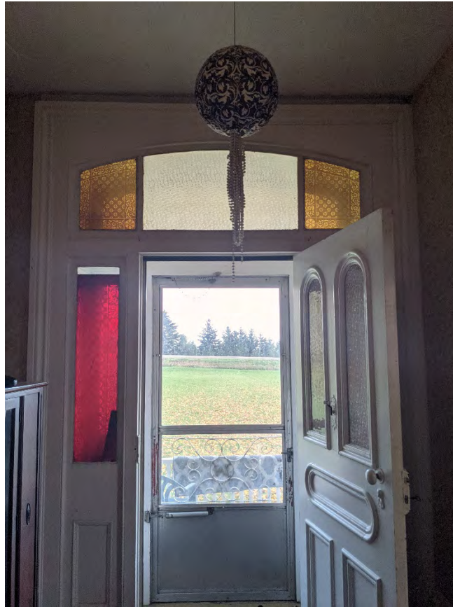
Figure 23: View of the front entrance including wood paneled door and interior transom and sidelights with coloured and patterned glass
