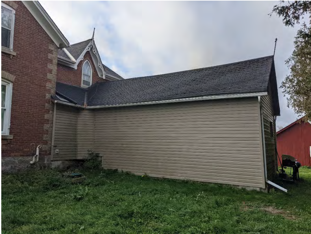
Figure 13: East wall of the one-storey addition
