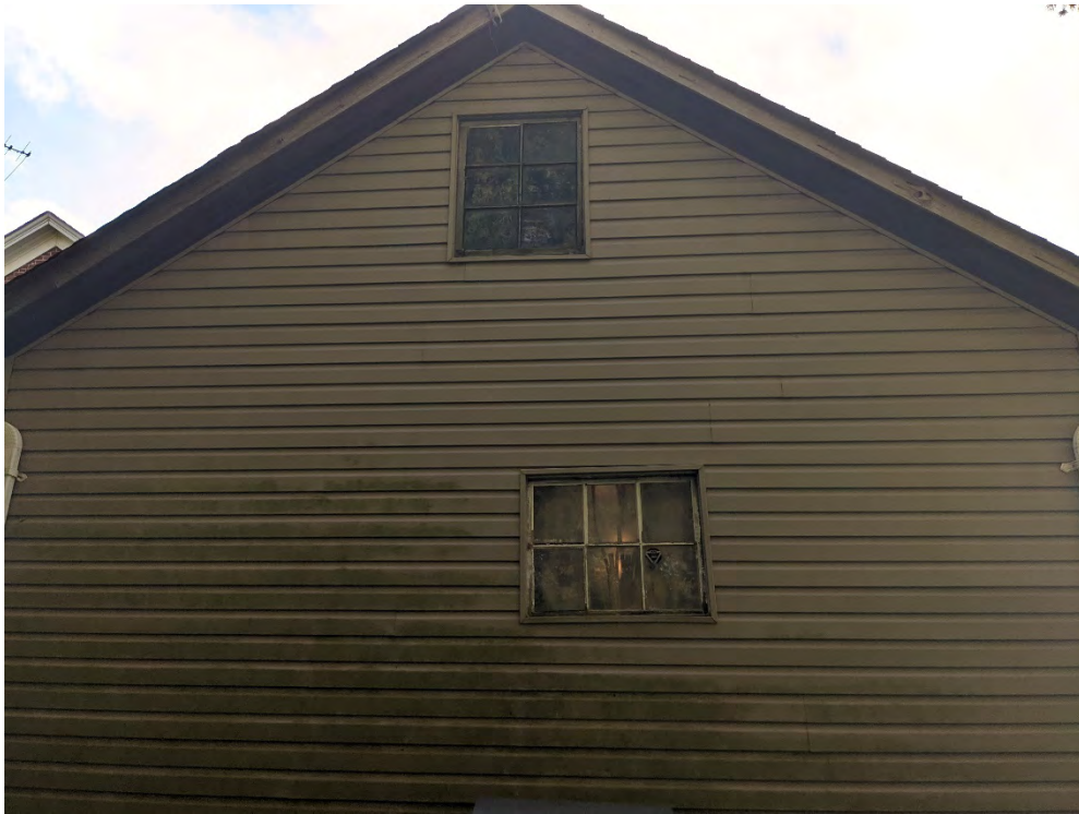
Figure 55: North elevation of the north addition
