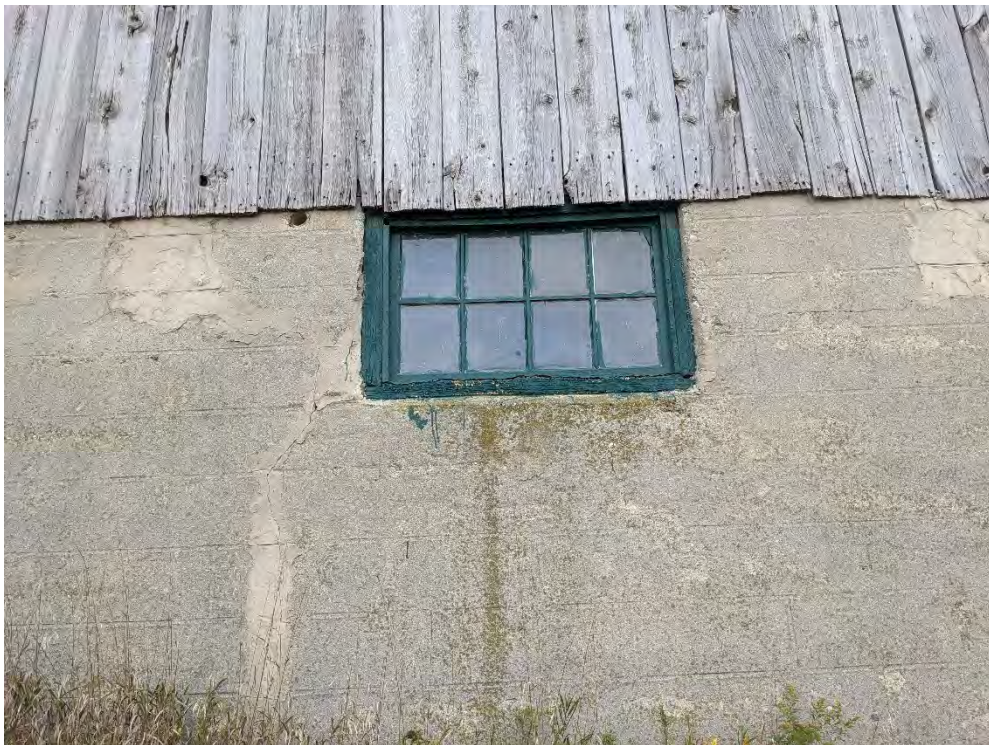
Figure 74: Typical window on the north elevation of the large barn
