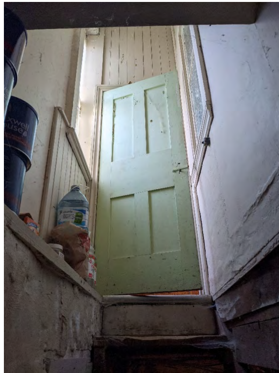
Figure 48: The door from the kitchen, view from the basement stairs
