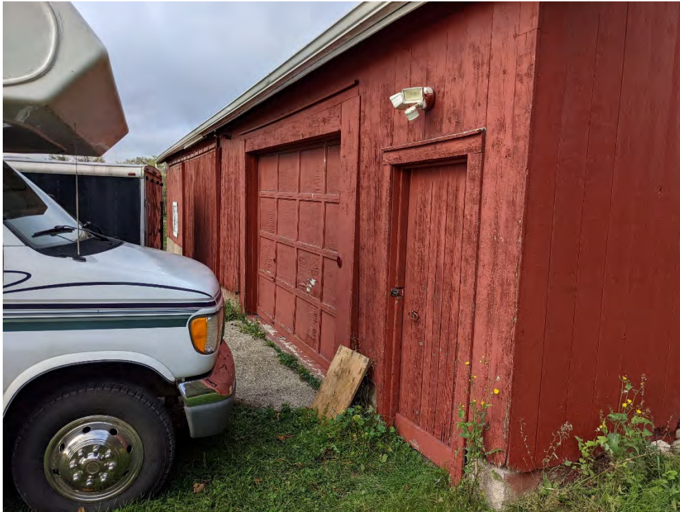
Figure 63: South façade of the driveshed
