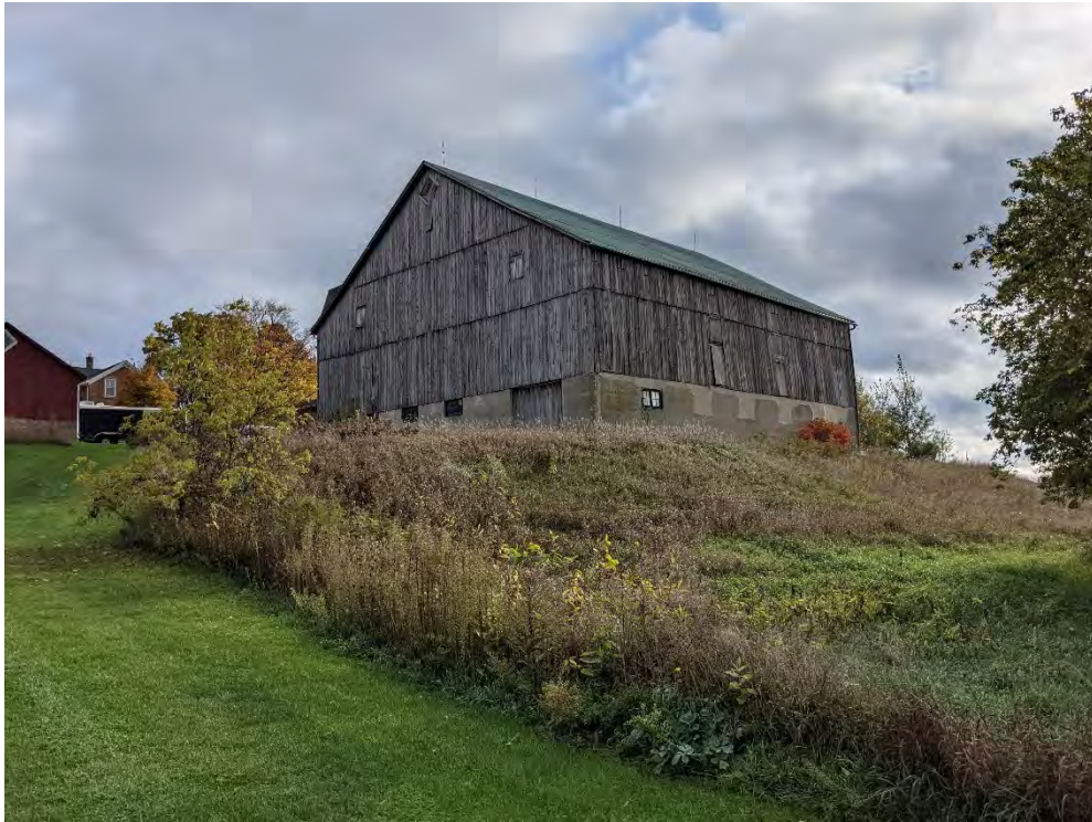
Figure 75: West and south façades of the large barn
