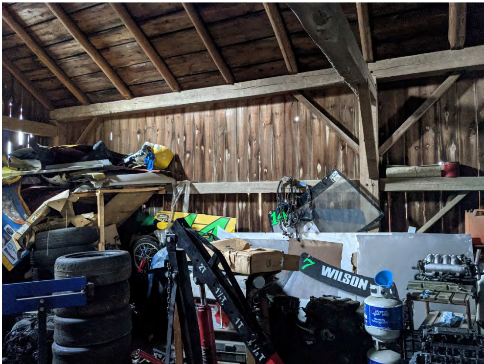
Figure 70: Interior of the driveshed with drop tie-beam, hand-hewn posts, and plates
