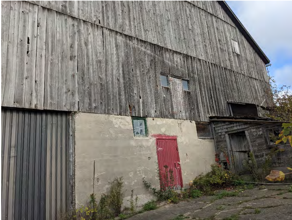
Figure 77: Lower level of the south façade of the large barn
