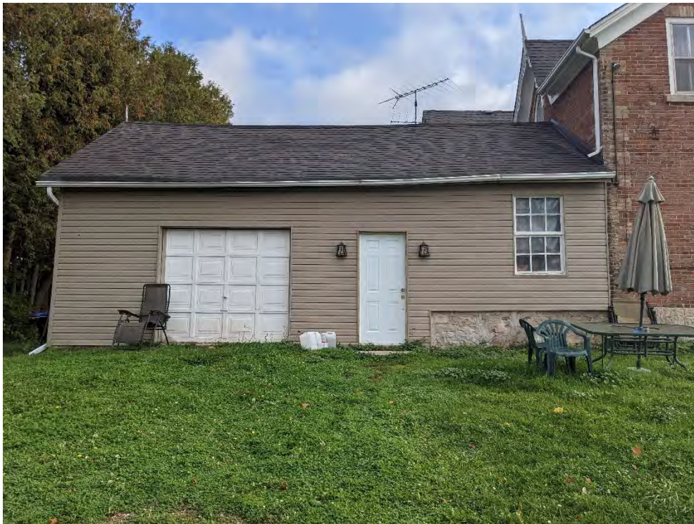
Figure 52: West elevation of the north addition
