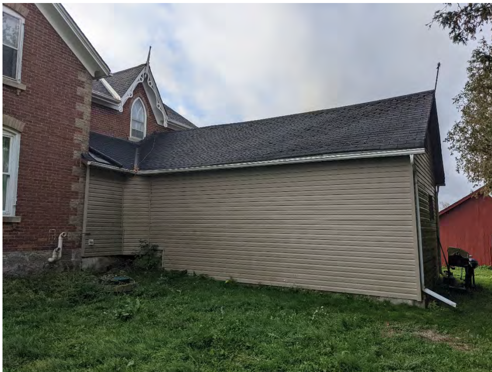
Figure 54: West elevation of the north addition
