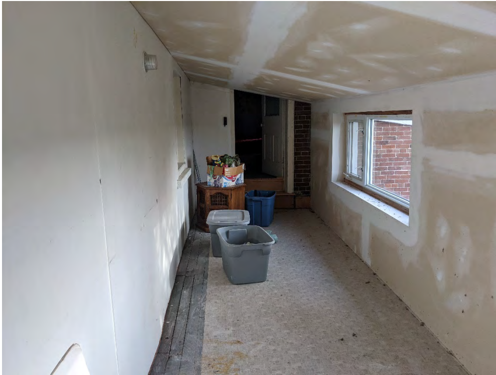
Figure 62: View of the second floor, inside the south addition, facing east
