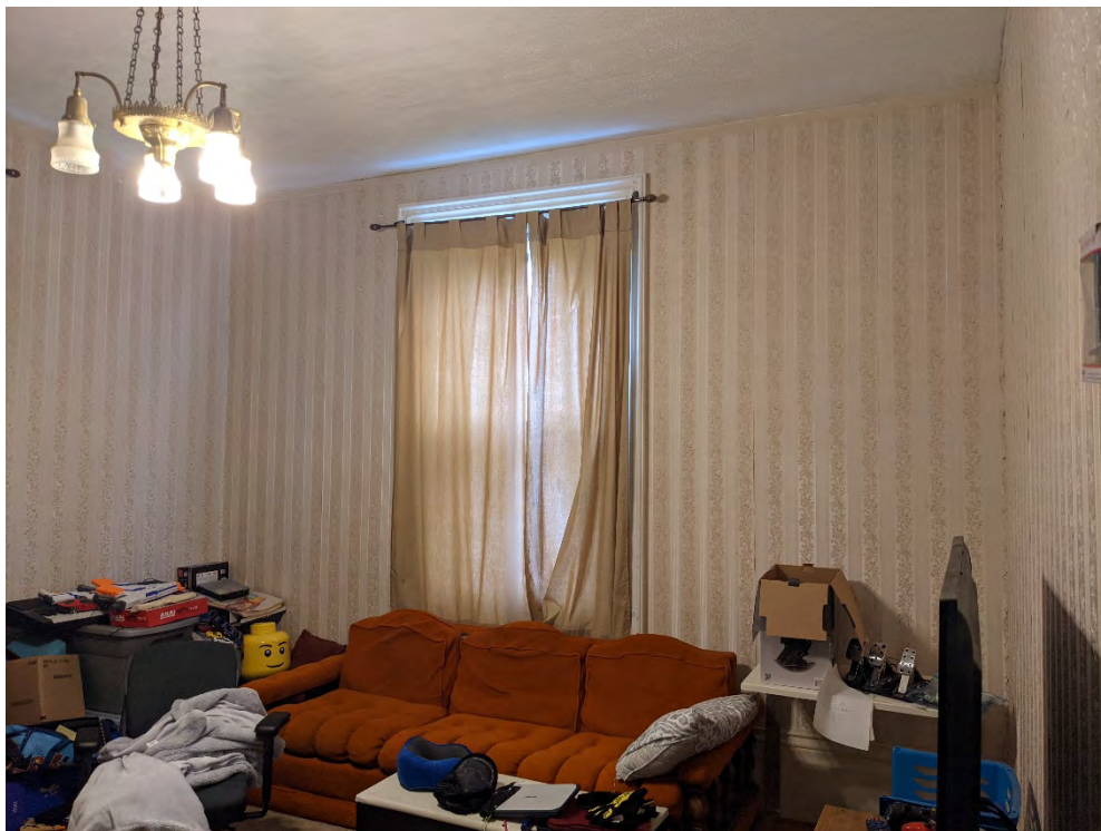
Figure 26: North front room, looking north
