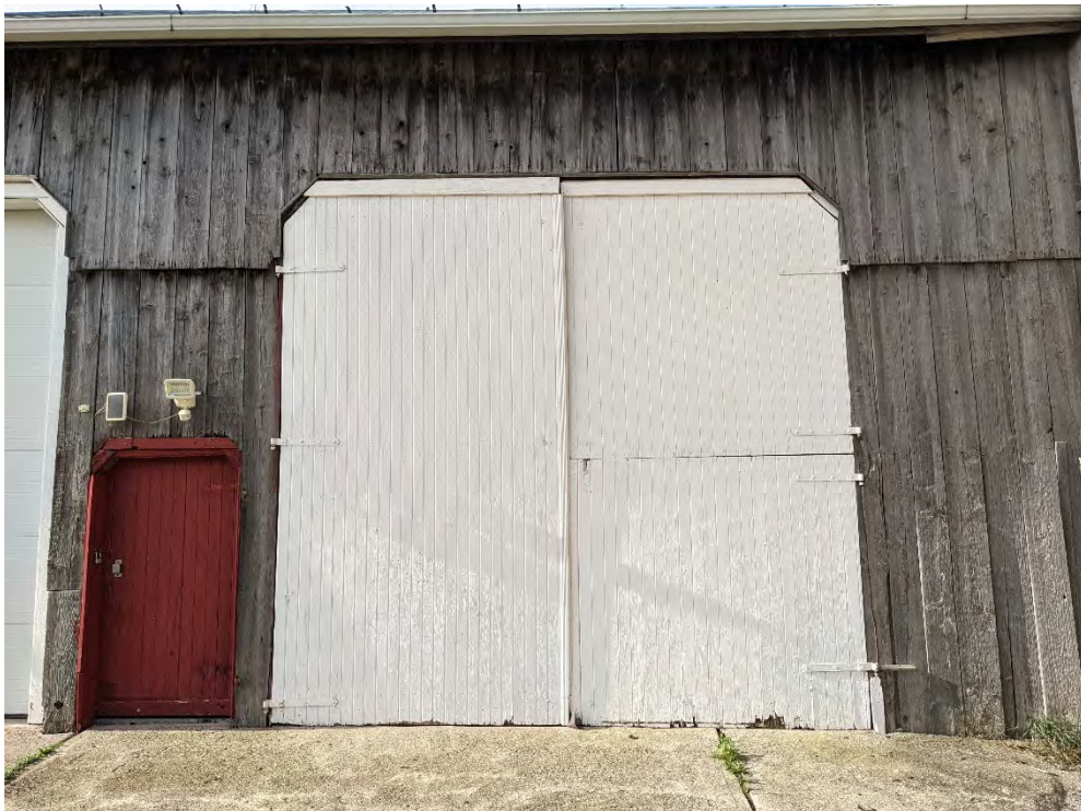
Figure 72: Large door on east elevation of the large barn
