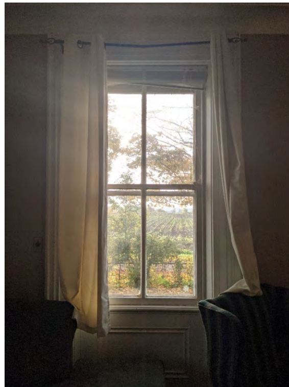
Figure 30: Wood window surround and paneling in south front room (also representative of paneling in north front room)
