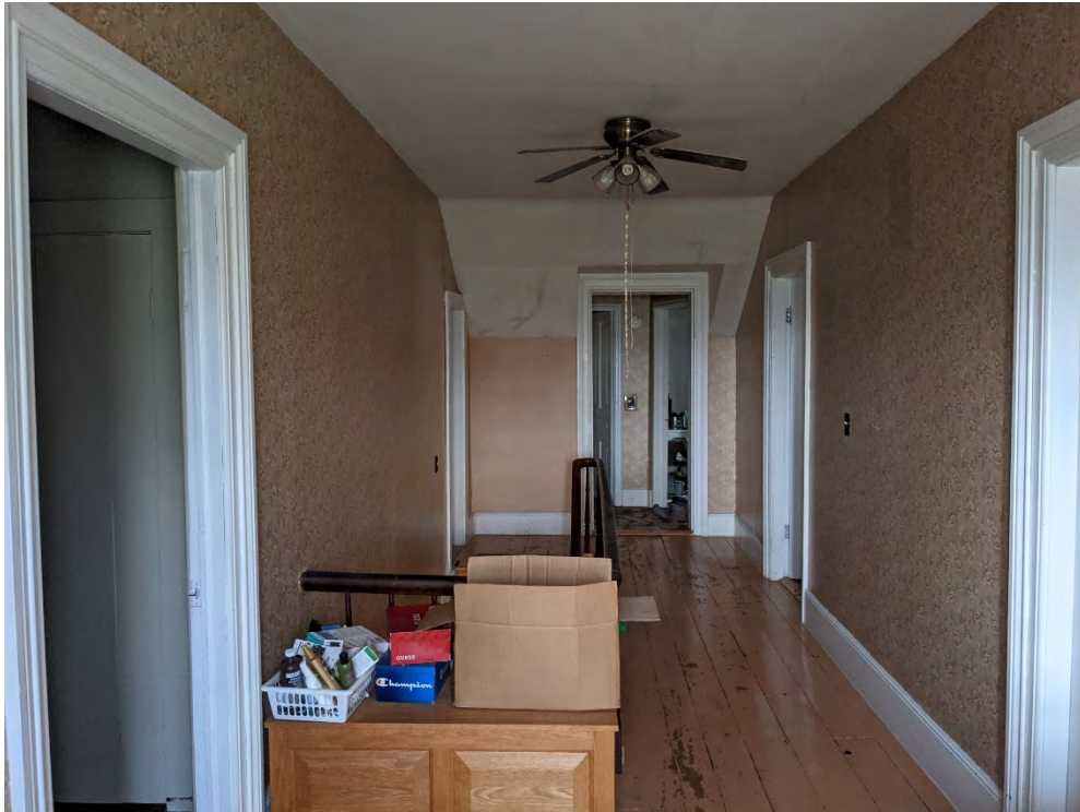
Figure 39: Second level hall landing, looking west
