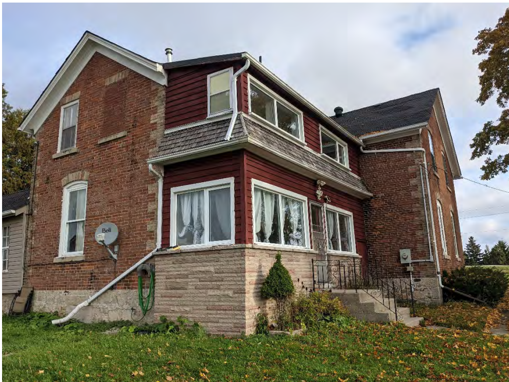
Figure 59: The south and west elevation of the south addition
