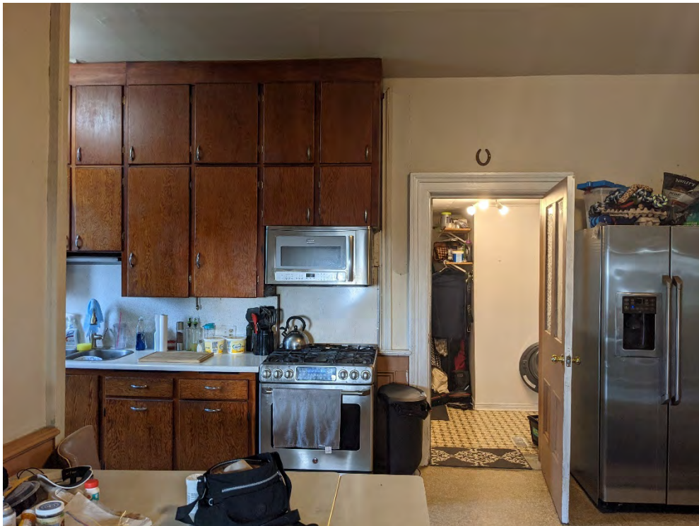
Figure 33: Kitchen Cabinets on north wall
