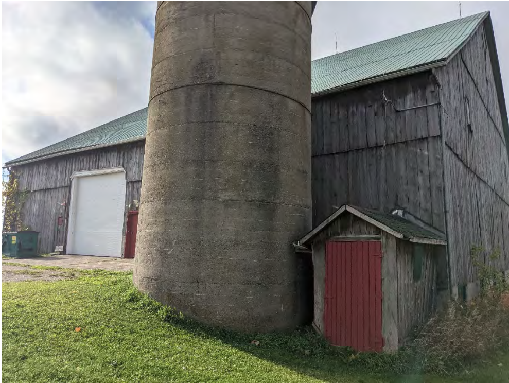
Figure 71: East elevation of the large barn
