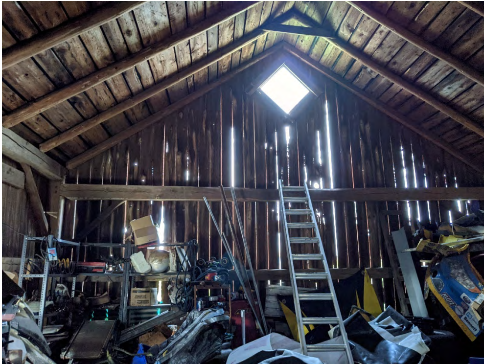
Figure 69: Dimension cut rafters
