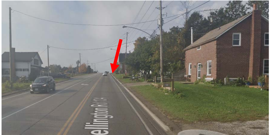
Exhibit 6-11: Stopping Sight Distance – East of Proposed Access Location (Looking Westbound from a point 130 m east of the Proposed Access Location)
