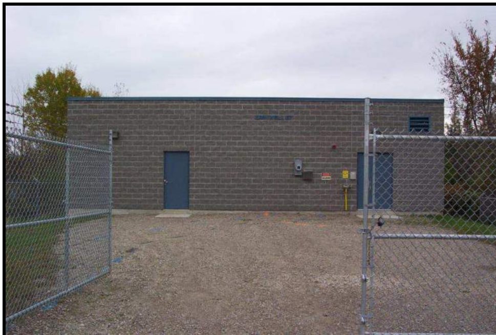
Image 12: Example of Well House Construction (Triton Engineering: Email dated January 4, 2018)
