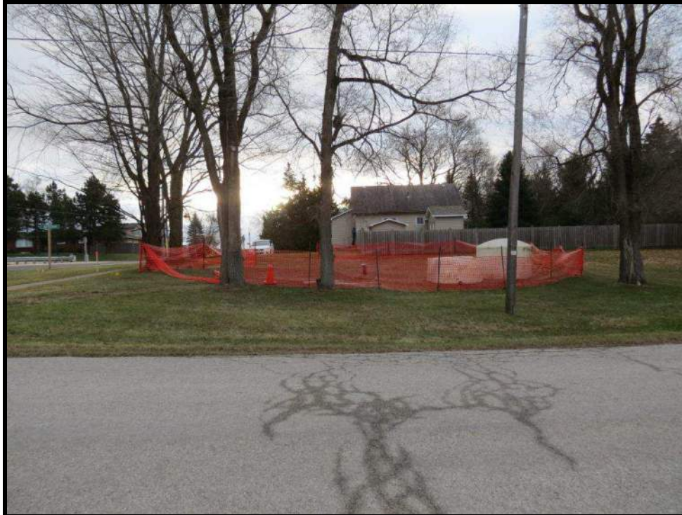
Image 6: View of Mountainview Well Site, 5378 9 th Line (November 29, 2017; View Facing Southeast)
