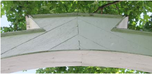
Figure 18: The back of the Stanley Park Gates arch. The planks for the sign are arranged in a uniform diagonal fashion and there is a seam in the middle that joins two curved planks of wood. (Photograph by M. Laszczuk).
