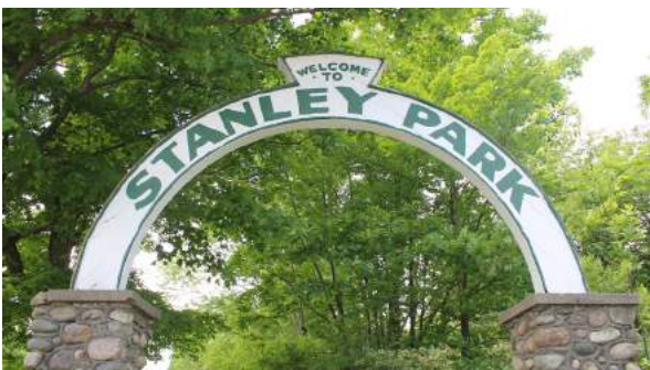
In descending order, Figure 19: Fieldstone arrangement and V-joint type mortar on the gate pier (Photograph by M. Laszczuk), Figure 20: Wooden arch and lettering of the Stanley Park gates (Photograph by M. Laszczuk).
