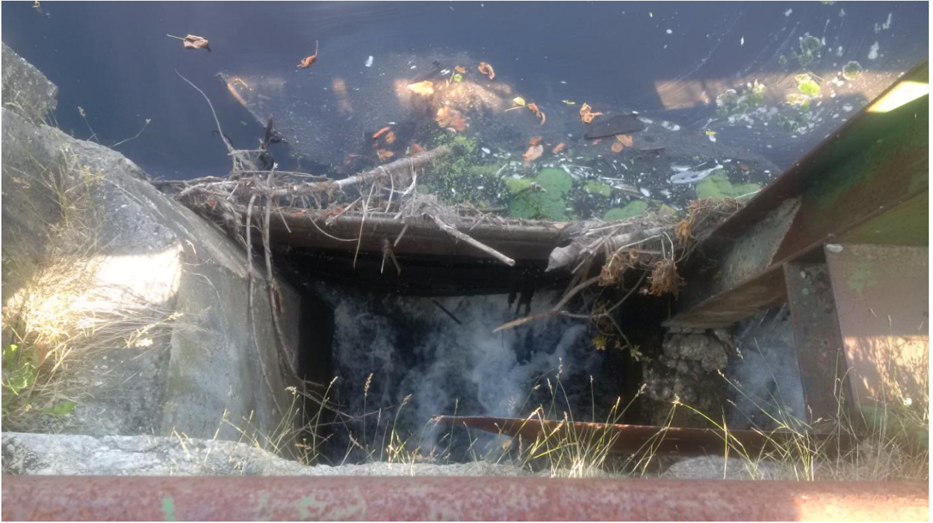
Overhead view of dam
