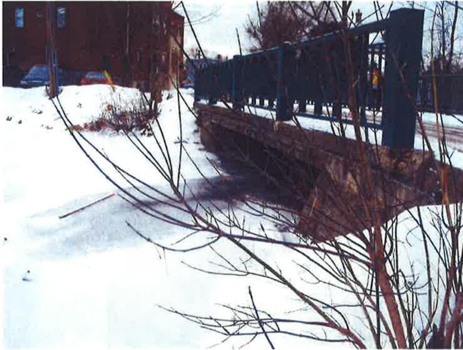
Figure 10-11 Charles Street Dam
