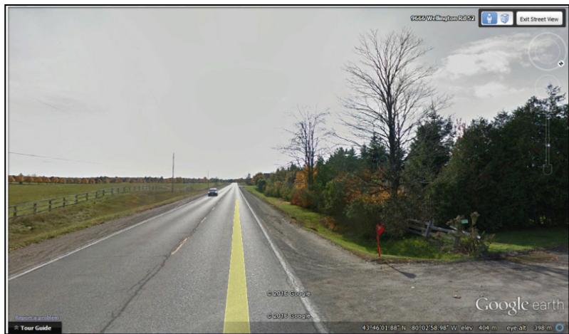
Looking west on Wellington Road 52 with vegetation screen on right side adjacent to subdivision (Aspen Court).
